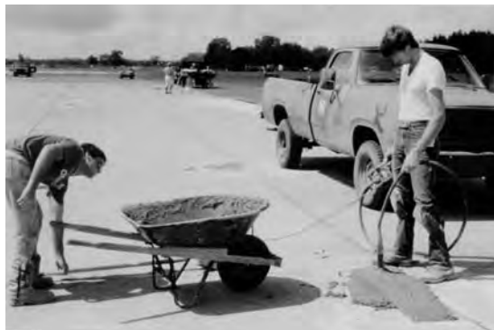
Figure 16.2. Consolidation of the repair material by vibration
