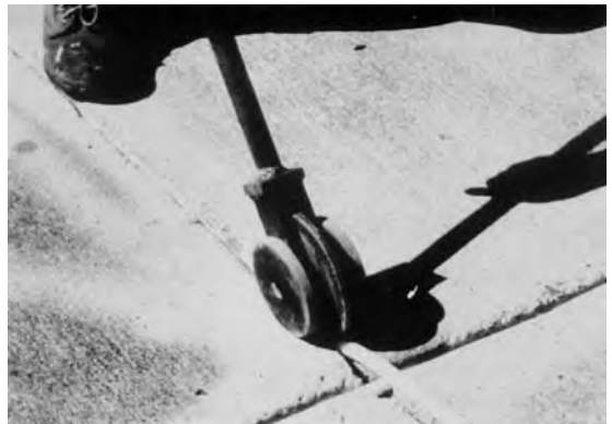
Figure 9.6. Installation of backer rod
