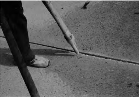
Figure 10.3. Sandblasting a joint face
