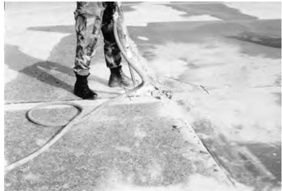
Figure 14.2. Using a jackhammer to remove damaged concrete
