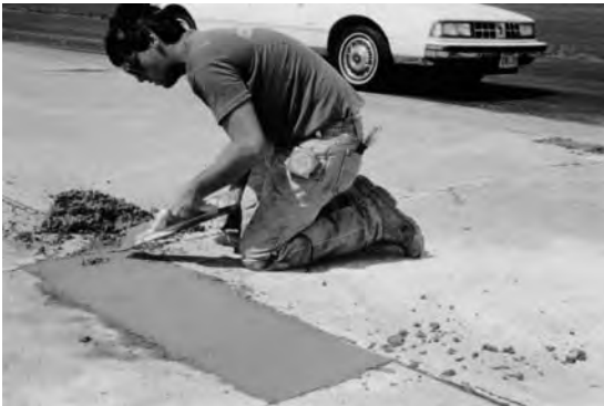
Figure 16.3. Finishing the patch surface
