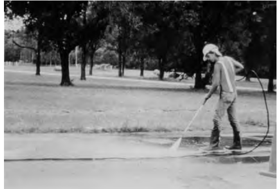
Figure 9.4. High-pressure water cleaning
