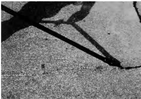
Figure 11.1. Sealing a crack
