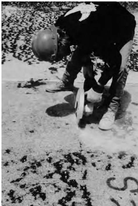
Figure 10.1. Hand sawing a crack
