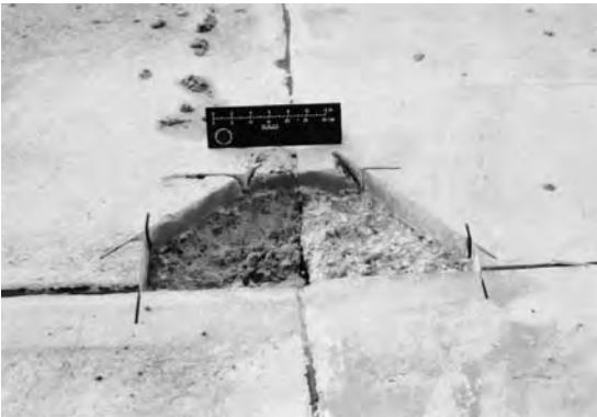
Figure 15.1. A spalled area on both sides of an expansion joint ready for installation of joint filler
