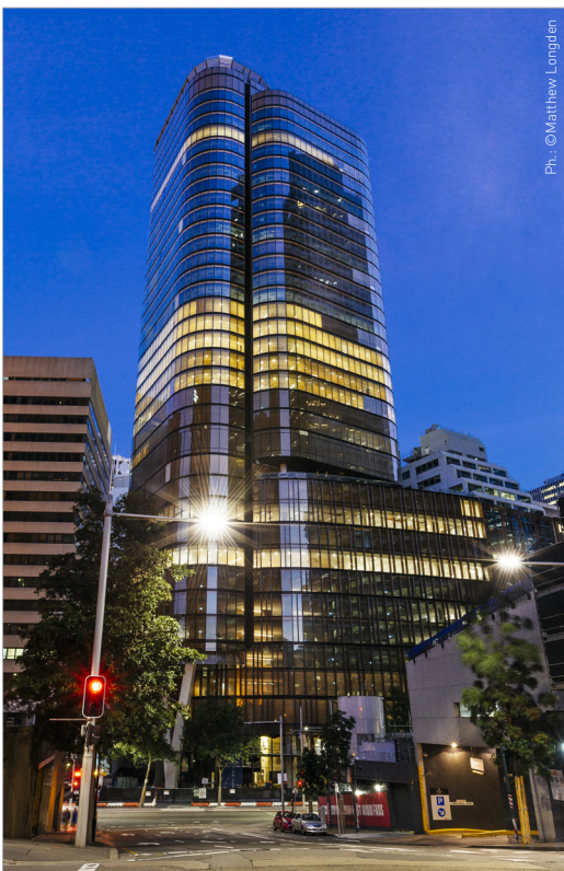
200 GEORGE STREET, SYDNEY | AUSTRALIA 20,000 m 2 mfree-S CCF including 2,900 façade integrated wooden venetian blinds. The façade performance is managed by Permasteelisa blind control system.
