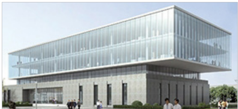
OPPLE INDUSTRIAL PARK, SUZHOU | P.R. OF CHINA The building resisted a typhoon in 2012. 24,300 m 2 mfree-S CCF with façade integrated venetian blinds. The façade performance is managed by Permasteelisa BlindTech.
