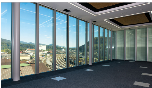
SBB OPERATIONS CONTROL CENTRE, OLTEN | SWITZERLAND 2,150 m 2 façade of which 1,400 m 2 mfree-S CCF with façade integrated automated venetian blinds.
