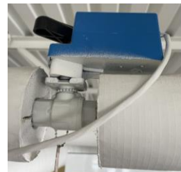
Hot Water Control Valve and Actuator
