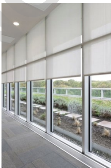
Figure A-12 Example of Solar-Adaptive Shading
