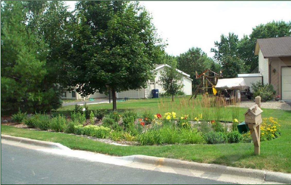
Figure A-16 Typical Bio-infiltration ‘Rain Garden’
