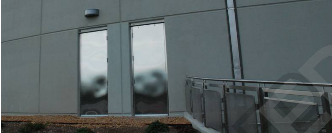
Figure 3-4 Emergency Exit Doors
