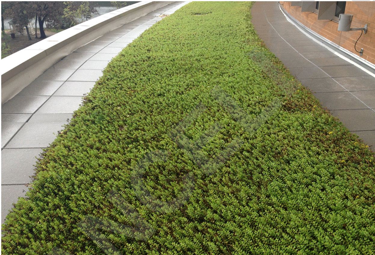
Figure A-3 Extensive Green Roof
