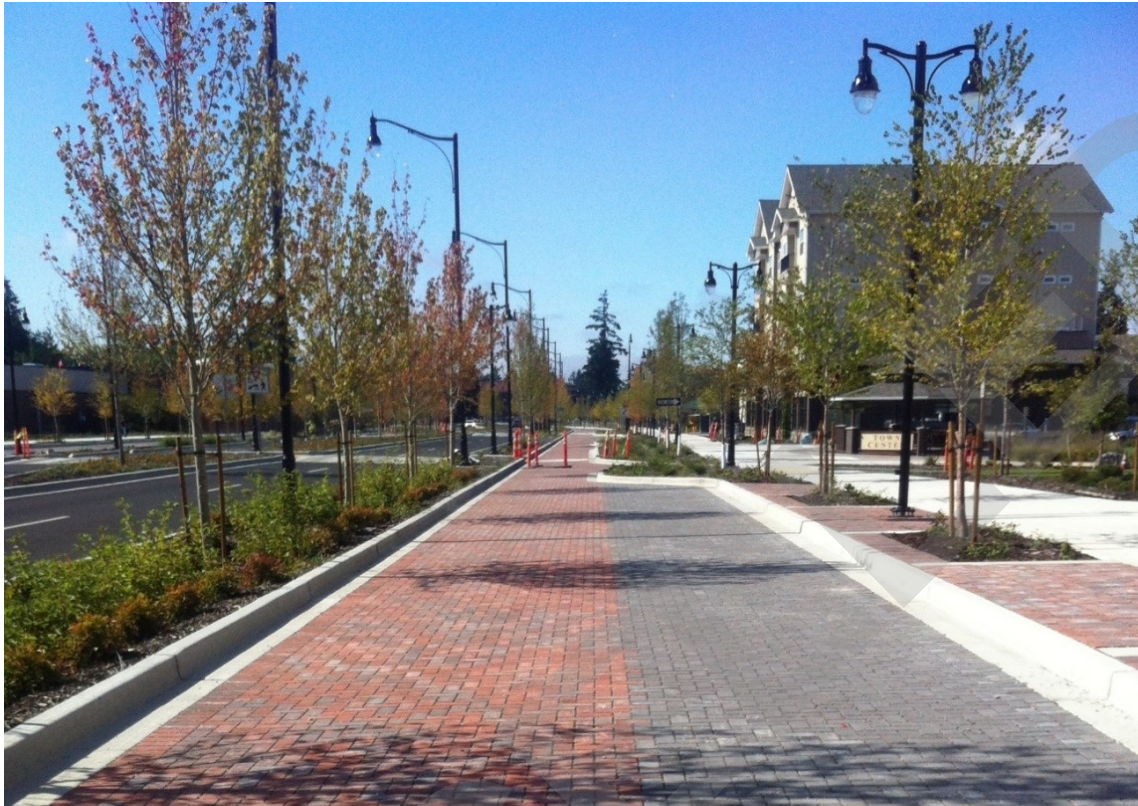
Figure A-4 Vehicular-Grade Pervious Pavement Systems 1
