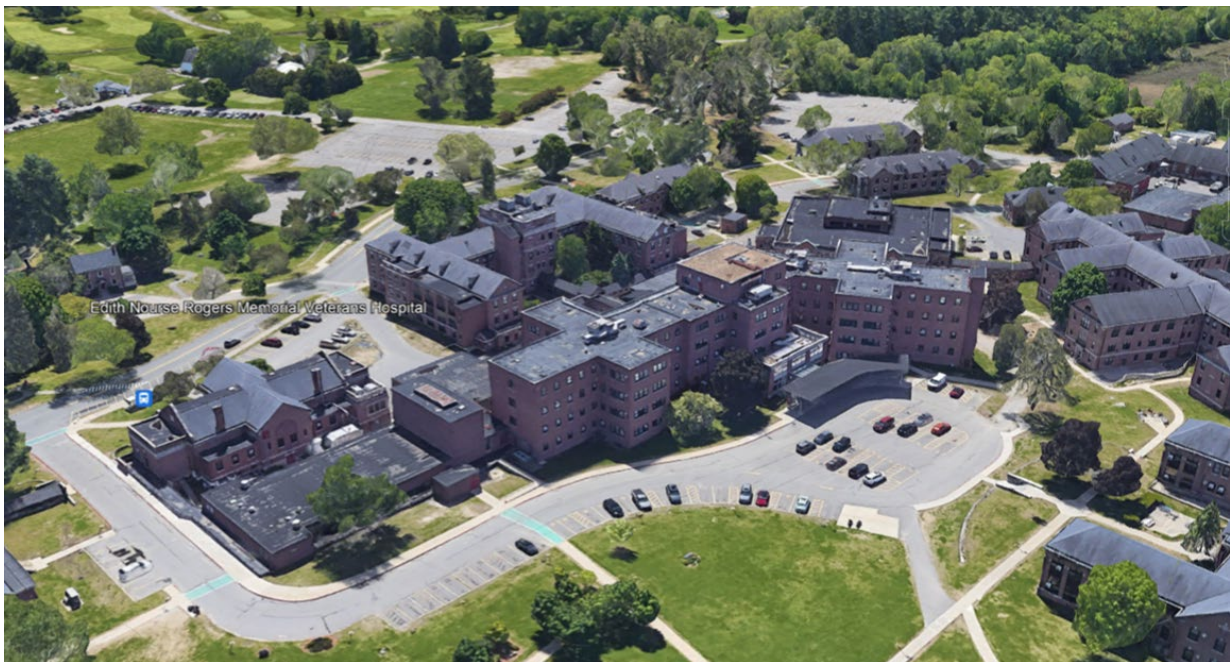
Bedford VAMC - Aerial View looking to the Southeast at Walk-In Entrance.
