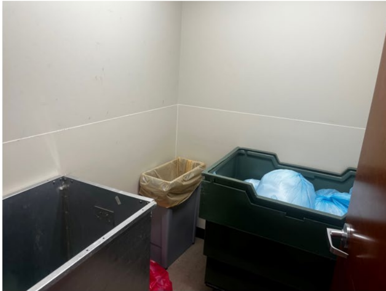
No hopper sink
