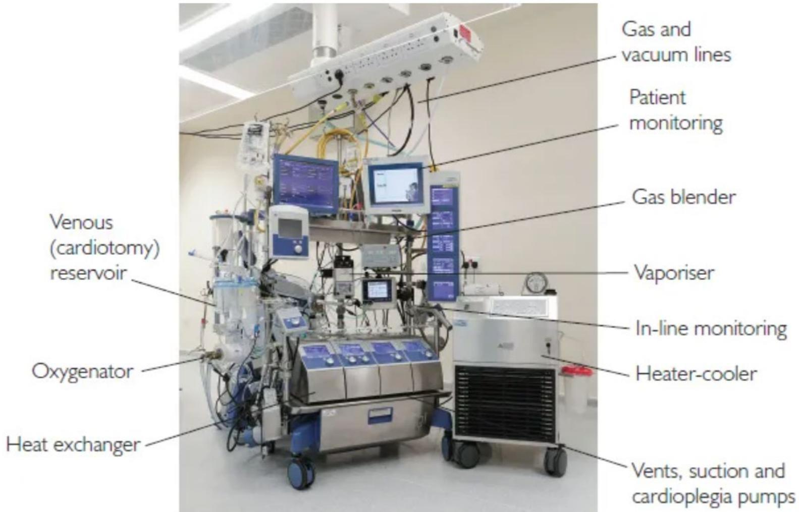
The Heart–lung Machine Room or "the pump room" is located adjacent to or proximal to both the cardiothoracic and hybrid operating rooms and is not directly accessible to either room as there is an open source of water within the pump room that may contribute to pathogens entering the OR's.
