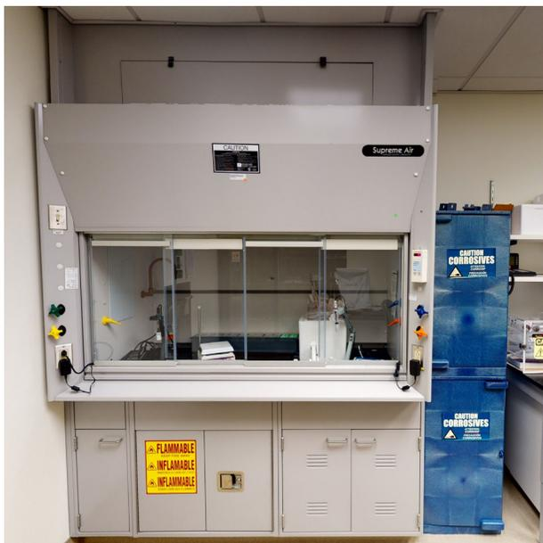
*Figure 21 A Fume Hood at the New Orleans VAMC R&D Facility is located next to a corrosive storage cabinet, and shares ventilation.*
