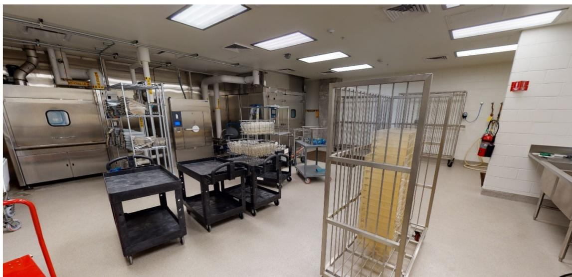
*Figure 30 The Soiled Cage Room at the New Orleans VAMC R&D Facility includes a pass-through autoclave, a cage washer, and a rack which can be used to wash bottles and other equipment in the cage washer if the bottle washer is down.*
