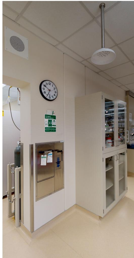
Figure 25 The Safety Shower / Eyewash Station is centrally located in the biomedical laboratory at the Rocky Mountain VAMC R&D Facility.
