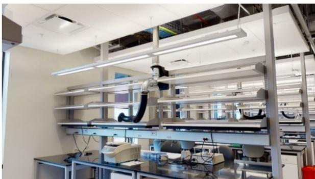
Figure 13 The adaptability of the Lab Bench Units at the New Orleans VAMC R&D Facility is enhanced with snorkel exhaust systems. (Note that the power and lab gases on the bench at the reagent shelf, pictured here, may inhibit long-term adaptability.)
