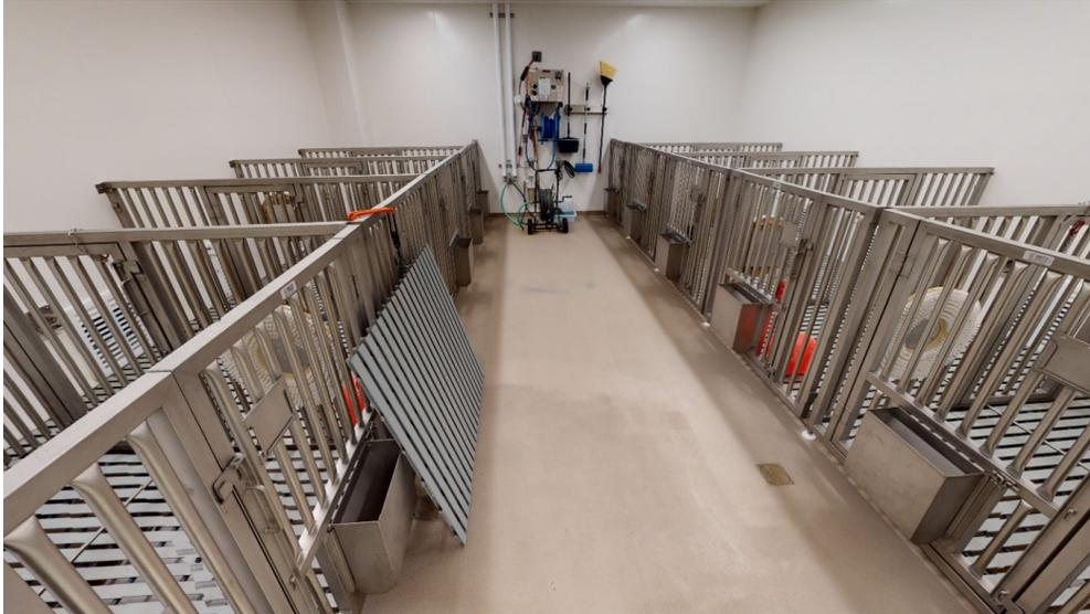
*Figure 27 Cages in the Large Animal Holding Room at the Rocky Mountain VAMC R&D Facility include openings for social interactions and open grate flooring for cleaning.*
