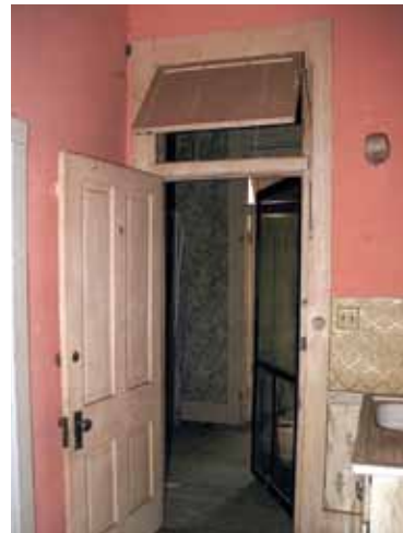
42 Recommended: [43] The wall and door glazing ensures that the corridor receives natural daylight and the operable transom helps air to circulate in this historic office building.
