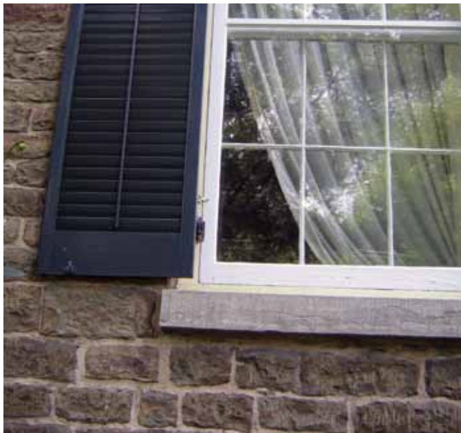
Recommended: [23-25] Historic exterior storm windows have been well maintained and continue to perform as intended.
