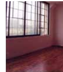
Recommended: [36-38] Original metal windows were retained and made operable during the rehabilitation of this historic mill complex. Installing patio slider doors as interior storm windows was a creative and successful solution to improve the energy efficiency of the existing windows.
