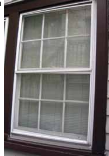
Not Recommended: [31-32] Ill-fitting exterior aluminum storm windows viewed from both inside and outside are clearly not energy efficient.
