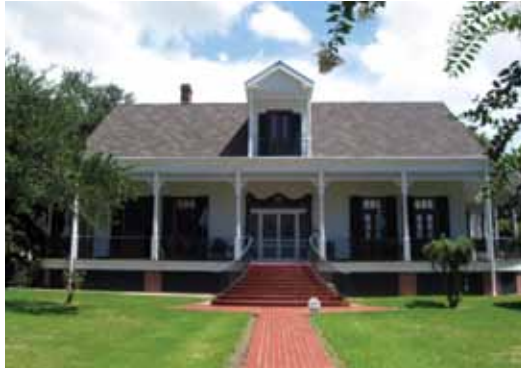
[16-18] Inherently sustainable features of historic buildings: Shutters and a deep porch keep the interior cool in a historic house in a warm climate (top); a skylight provides natural light to the interior of this mid-20th century house (center); partially glazed partitions and doors allow natural light into the corridor of a historic office building (bottom).
