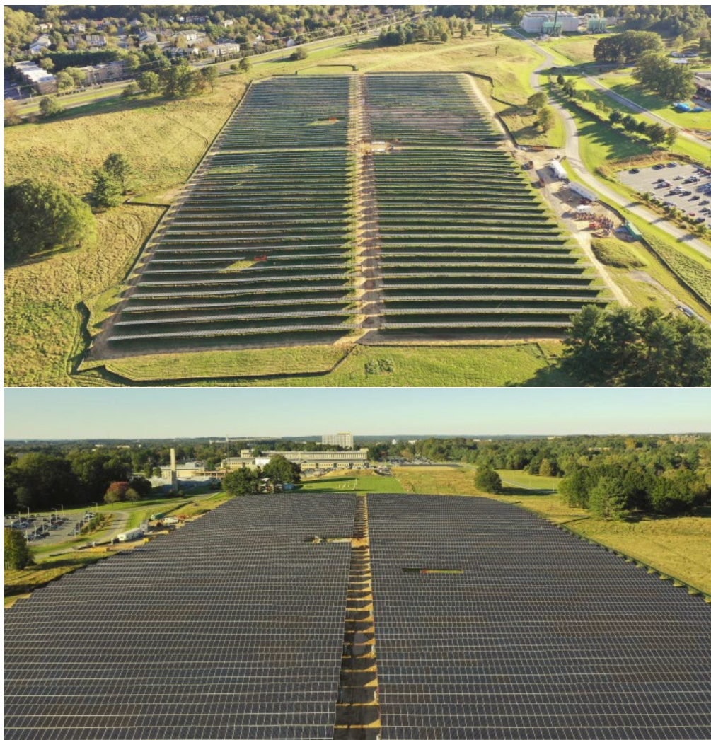
Figure 11-5 5 MW Solar Photovoltaic System (NIST Campus in Gaithersburg, MD)
