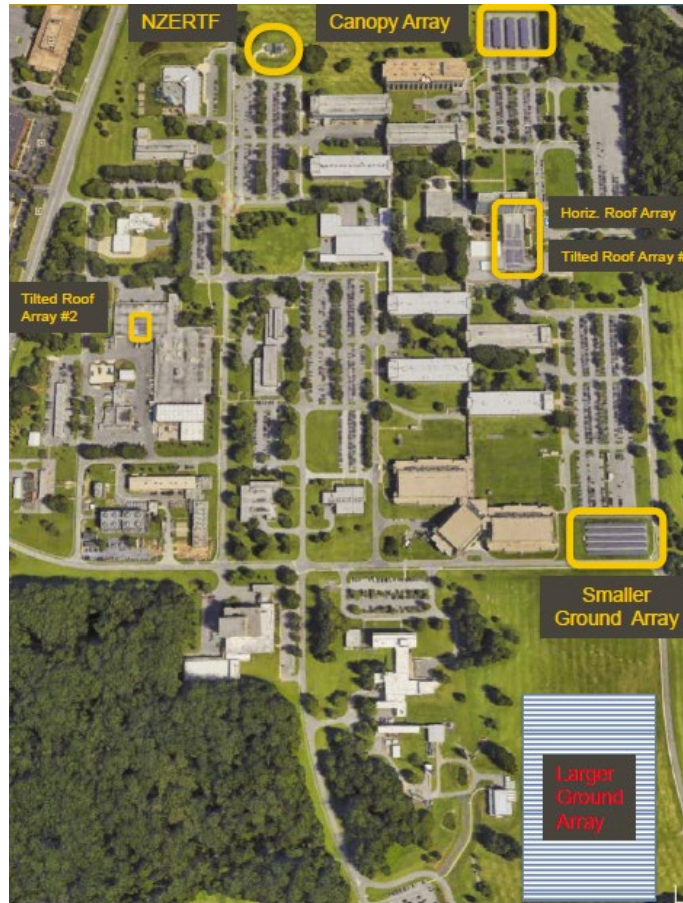
Figure 11-4 Solar Photovoltaic Systems on NIST Main Campus
