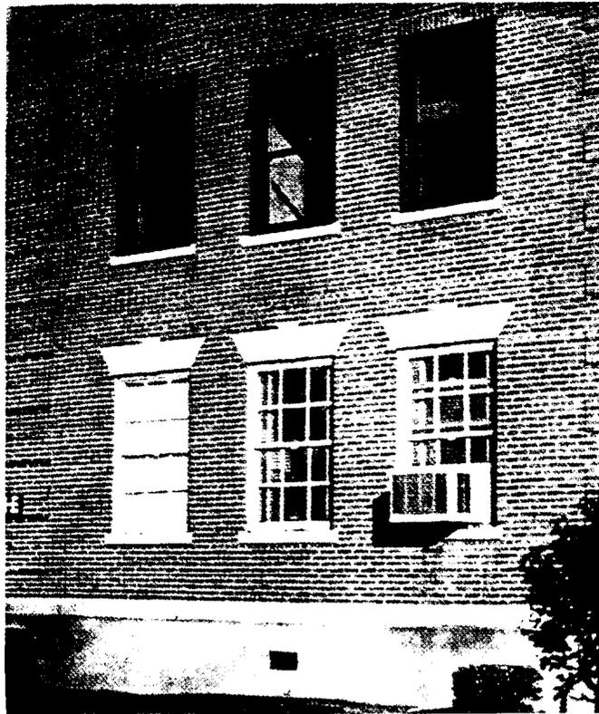
Figure 4-18. Historic Windows Inappropriately Replaced.
