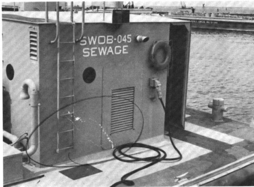
FIGURE 2-8 Shore Power Receptacle
