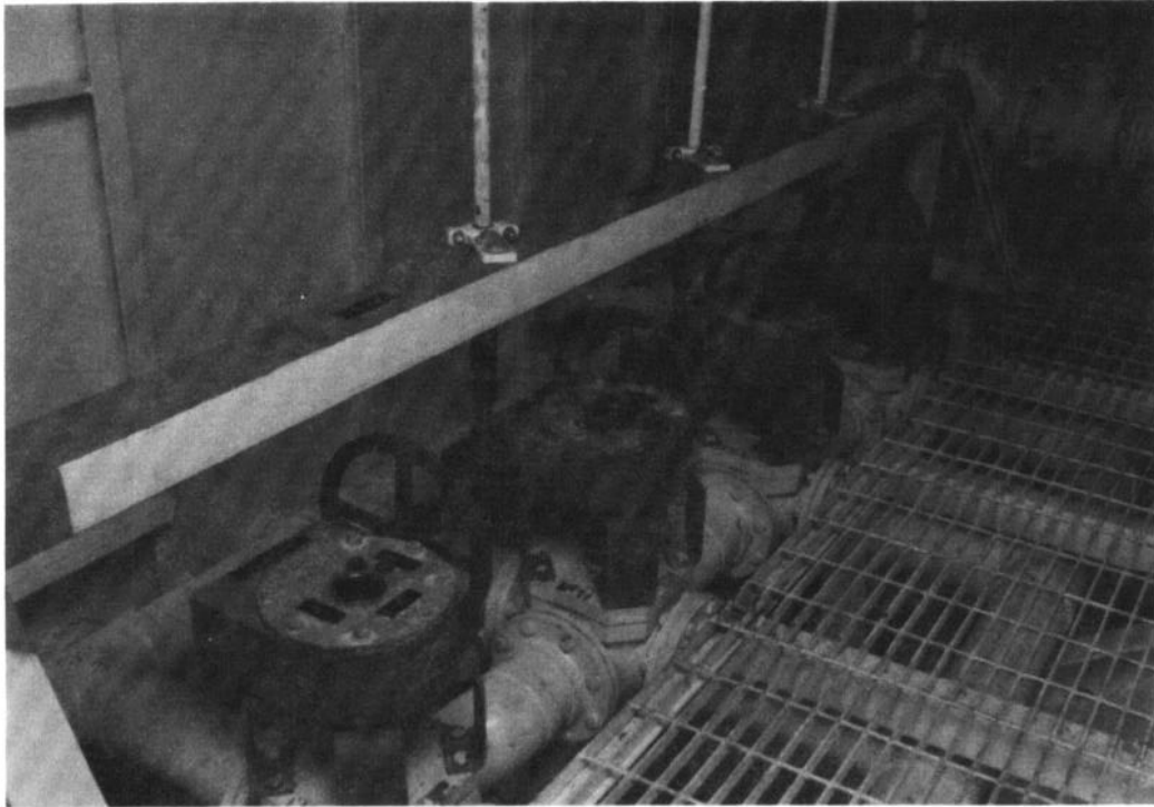
FIGURE 2-15 Pump Room Manifold
