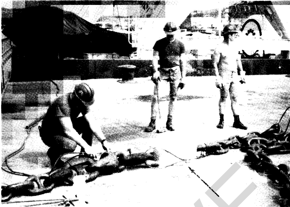
Figure 8-7. Link Anode Installed in a Chain Section
