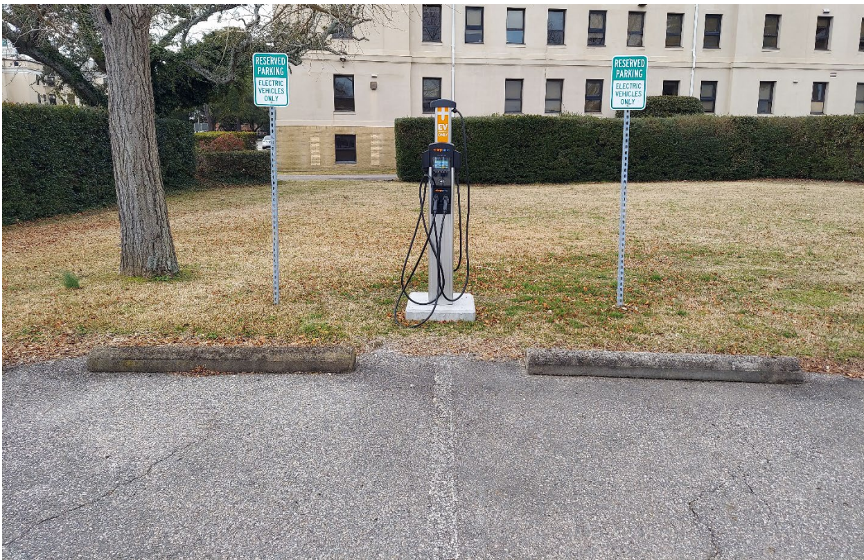
Figure 1-1 Electric Vehicle Parking Stalls
