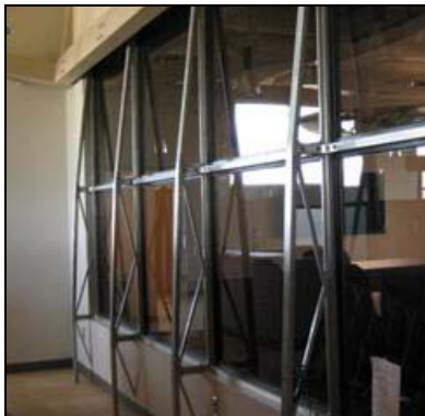
Figure 5 - Salvaged Window and Bow Trusses, Propellants North Facility, Kennedy Space Center
