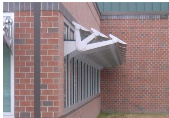
Figures 2-12 and 2-13. U.S. EPA New England Regional Laboratory, Chelmsford, Massachusetts (LEED Gold Rating, Version 1.0) Reflective light tubes, with diffusers designed to fit suspended ceiling systems, and exterior light shelves bring daylight deep into the building. (Photo: Don Horn)
