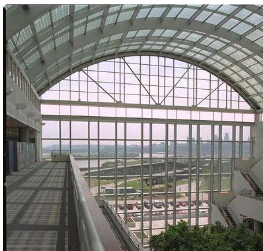
Figure 2-10. Atrium at the U.S. EPA Regional Headquarters, Kansas City, Kansas. The atrium design allows most of the office space in the building to receive natural light. The atrium's glass has a low-emissivity coating to allow visible light to enter while reflecting large percentages of the infrared spectrum, thereby controlling heat gain. (Photo: From Off the Shelf , Koll Development Company)
