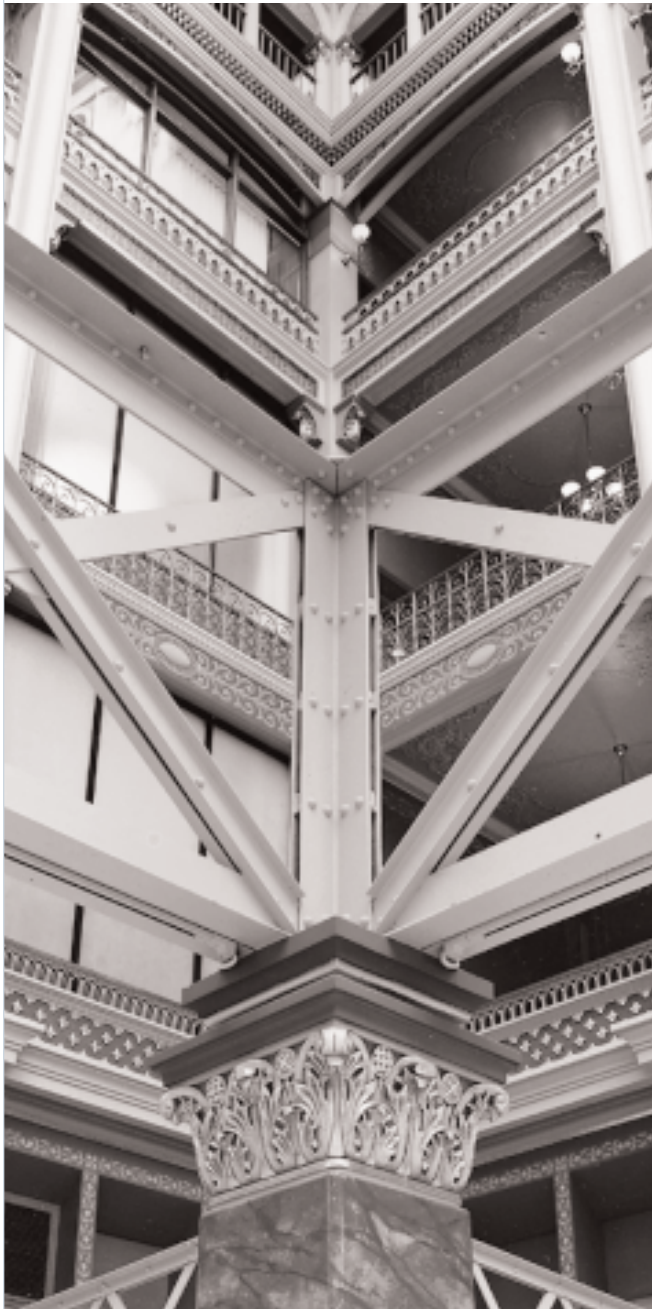
Steel bracing in the Milwaukee Courthouse
