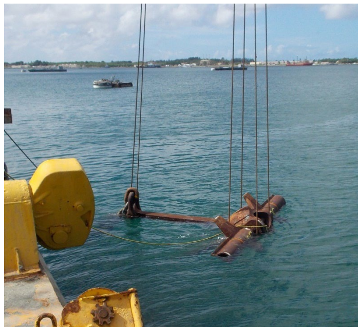
Figure 5-8 Stockless Anchor Deployment
