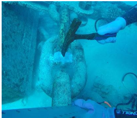
Figure 3-51 Tapping the Zinc Anode
