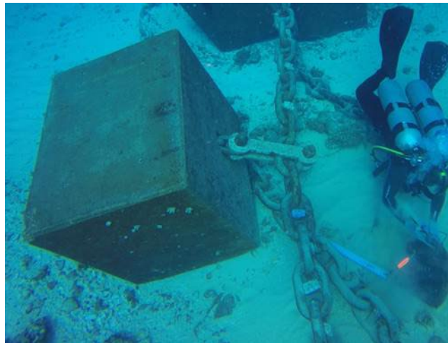
Figure 3-45 Sinker and Plate Shackle
