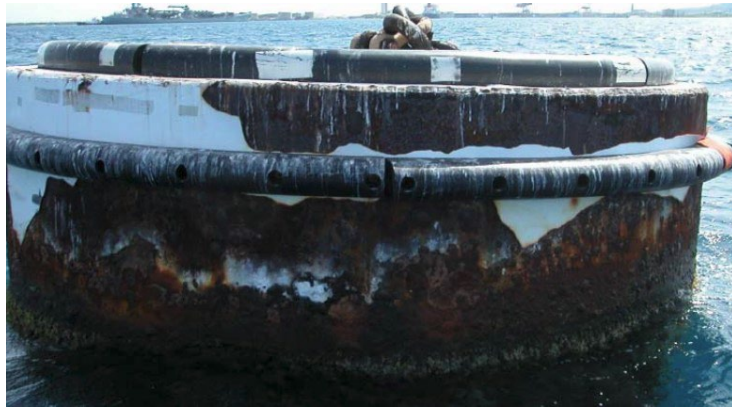
Figure 3-30 Outer Coating Loss on Steel Buoy
