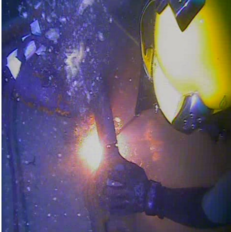
Figure 5-11 Navy Diver Cutting Connecting Shackle
