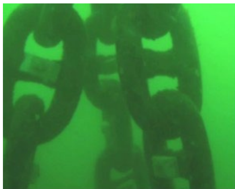
Figure 3-46 Ground Legs Just Below the Ground Ring
