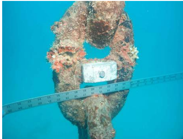
Figure 3-50 Zinc Anode Installed on a Chain Link
