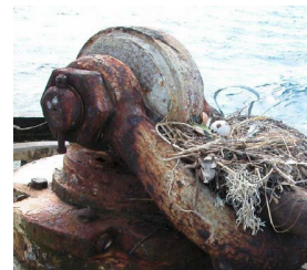
Figure 3-23 Heavy Corrosion
