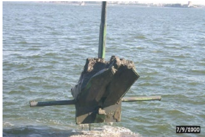
Figure 5-12 NAVMOOR Anchor Recovery
