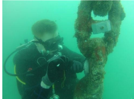
Figure 3-54 Diver Attaching Anode to Chain
