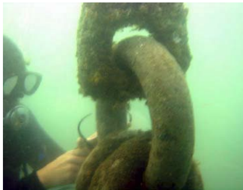
Figure 3-44 Ground Ring Assembly
