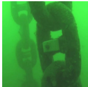
Figure 2-50 Chain Stud Anode Installed
