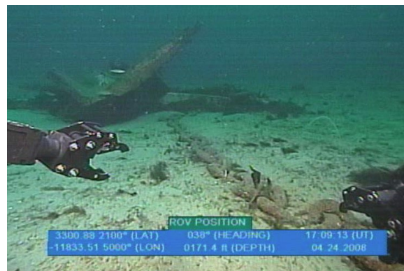
Figure 3-49 Upside Down Anchor and Incorrect Alignment
