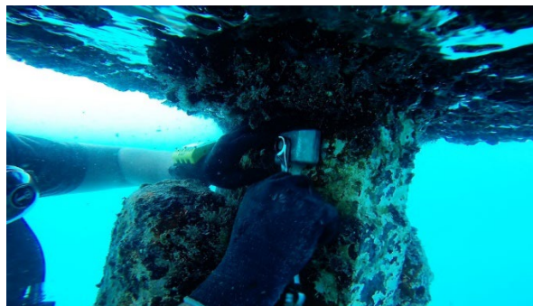
Figure 3-55 Diver Installing a Zinc Anode on the Bottom Buoy Padeye
