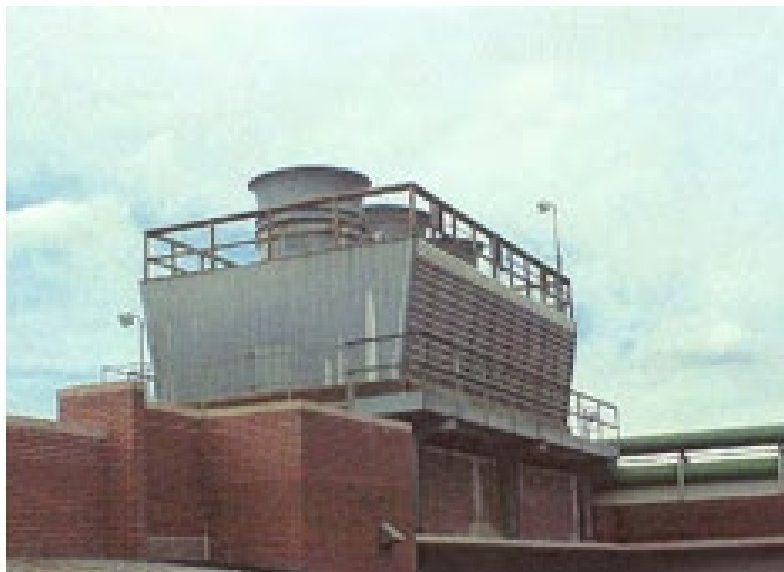
Figure 5-7 Cross-Flow Cooling Tower
