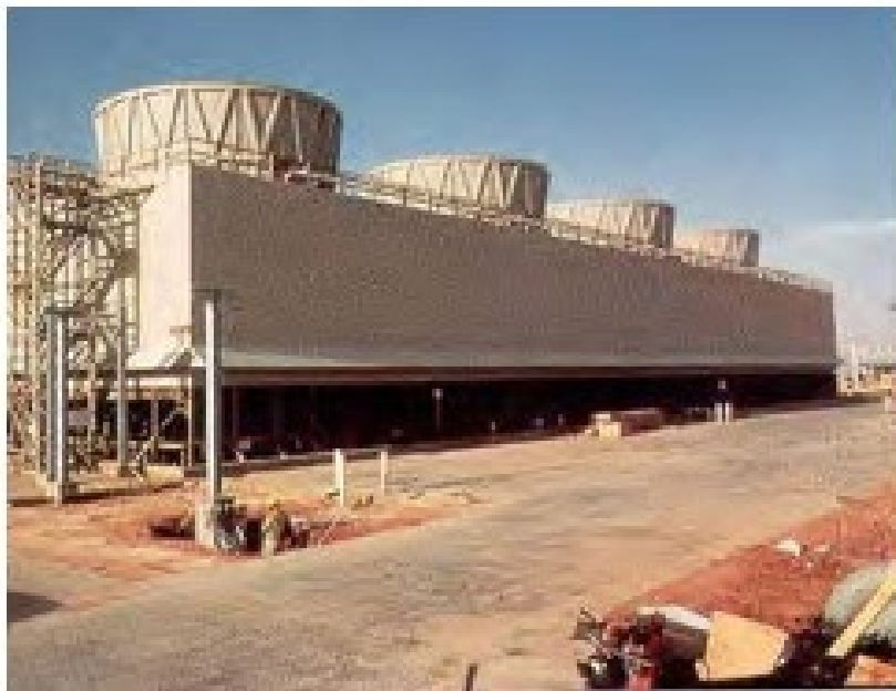
Figure 5-9 Counter-Flow Cooling Tower
