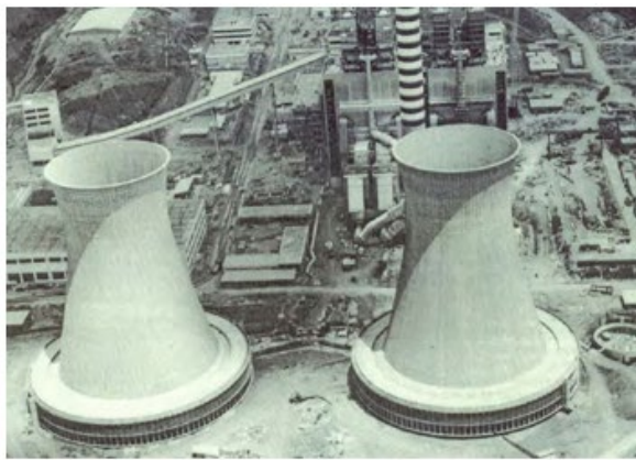
Figure 5-5 Hyperbolic Natural-Draft Cooling Towers
