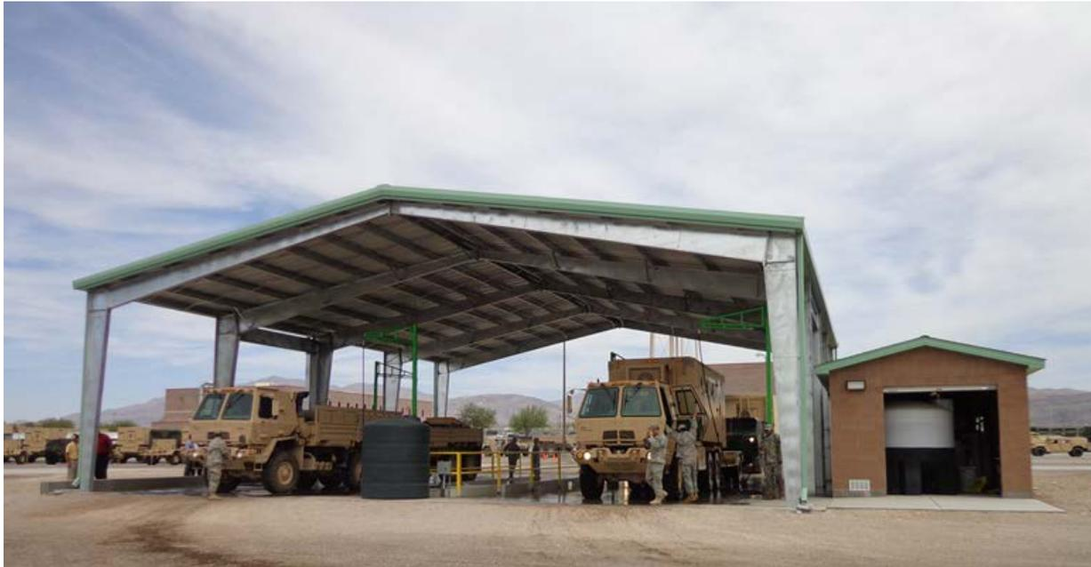
Because of limited space at the facility and the number of vehicles to be washed, a decentralized, Net Zero dual lane wash facility was constructed.
