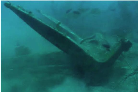
Figure 3-49 Upside Down Anchor and Incorrect Alignment
