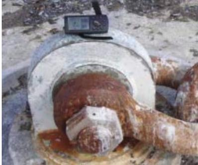
**Figure 3-28 Excessive Corrosion on Tension Bar Padeye**
