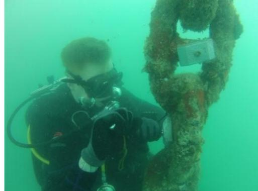
Periodically, the diver will find chain links where the anode bolts were sheared at the stud during installation, preventing anodes to be attached to the chain link. The quantity of chain links unable to attach a zinc anode to should be recorded in the comment section of the mooring's inspection data sheet.
