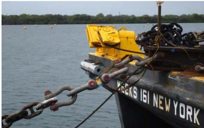
Embedment anchors installed in mud or soft sediments may have a wire rope between the anchor and the mooring chain to aid in the leg cutting through the soil and to minimize the keying (or net upward movement) distance to obtain the required test load.
