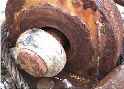
**Figure 3-21 Nut on Shackle Pin Not Fully Seated**
