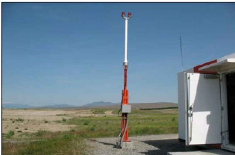
Figure 3-2 Omni-Directional Distance Measuring Equipment (DME) Antenna
