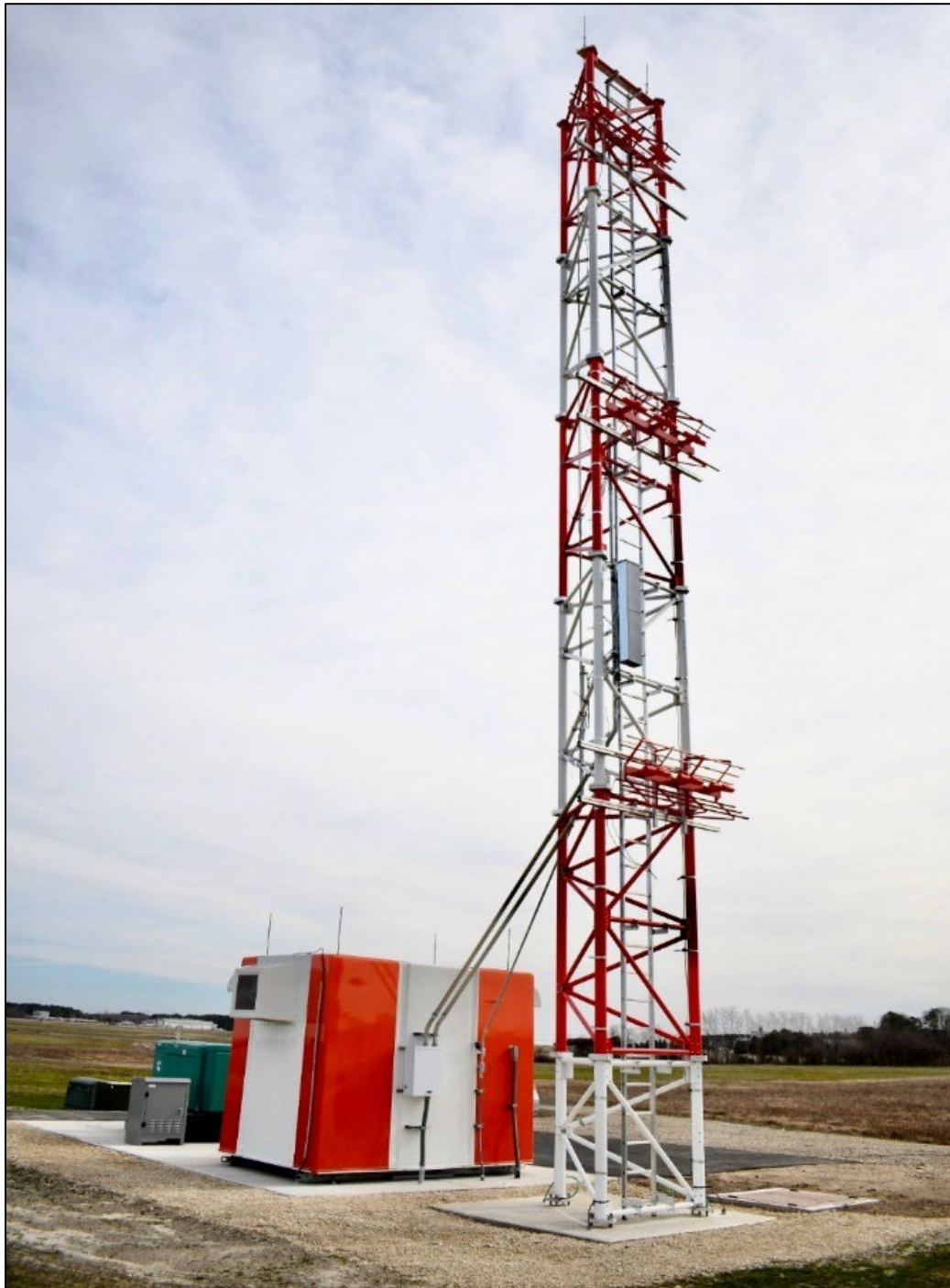
Figure 4-4 ILS Glide Slope Antenna and Equipment Shelter
