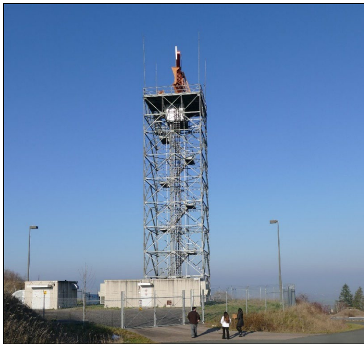
Figure 5-3 Typical DASR without Antenna Cover (Army)
