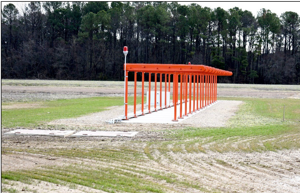
Figure 4-3 ILS Localizer Antenna Array
