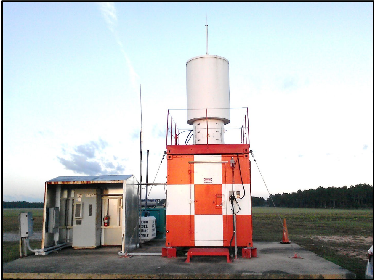
Figure 3-14 Typical Shelterized TACAN Antenna with Adjacent Electrical Shed
