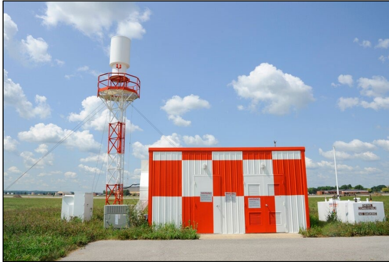
Figure 3-3 Typical TACAN Facility
