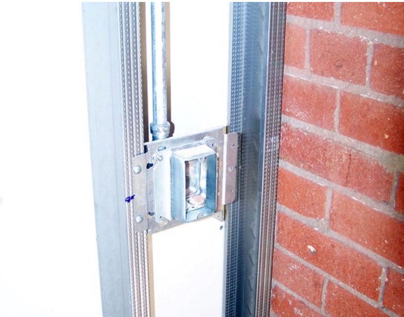
Figure 3-7 Furred Out Wall for Utilities
