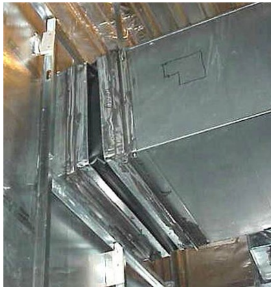
Figure 3-11 Duct Penetrations
