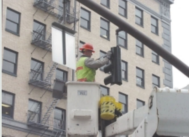
A City-bired contractor installs one of more than 13,000 LED lamps during the fall of 2001.
