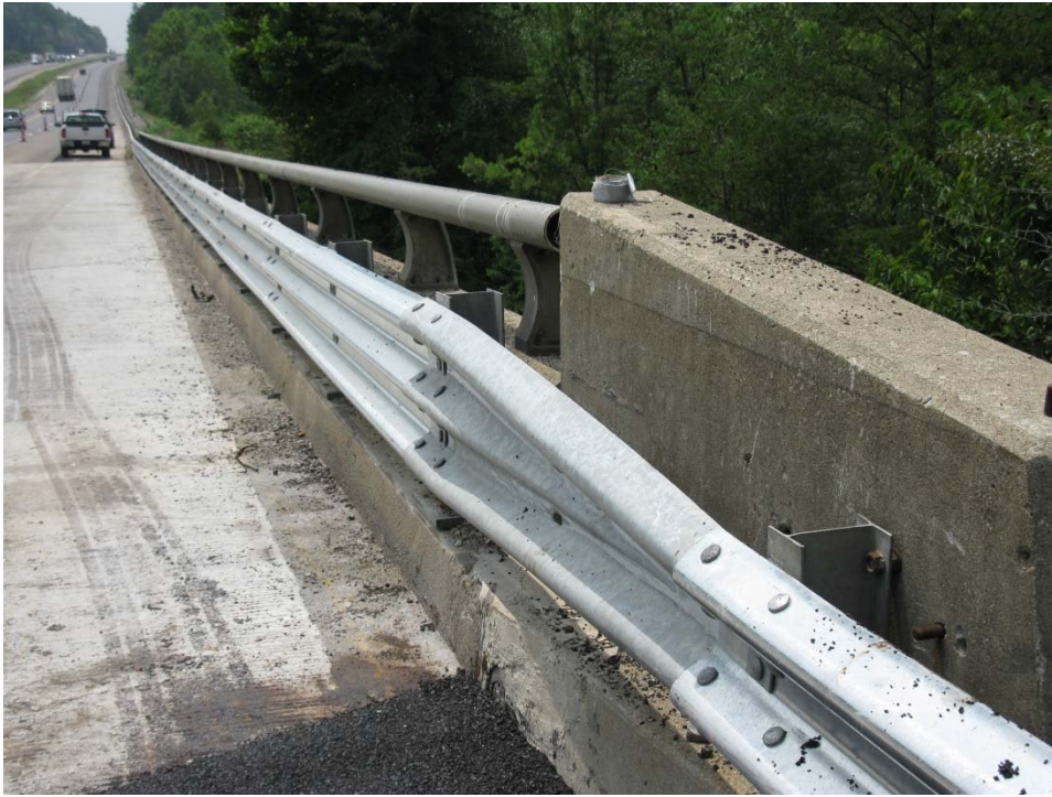
Figure 3.2-Bridge rail retrofit with thrie beam
