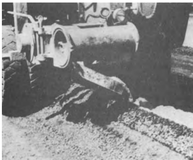
Figure 4-9. Windrow-type mechanical spreader placing cement on windrow.
