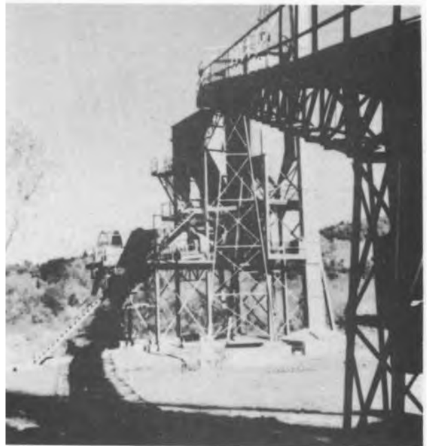
Figure 4-5. Batch-type central plant used for mixing soil-cement.
