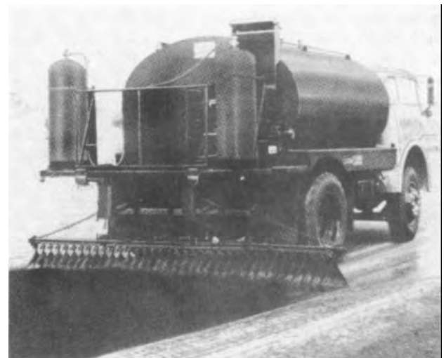
Figure 4-51. Distributor applying asphalt.
