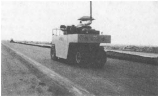
Figure 4-42. Pneumatic roller completes compaction of LCF base.
