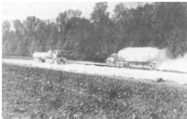
Figure 4-25. Application of lime by a bulk pneumatic truck.
