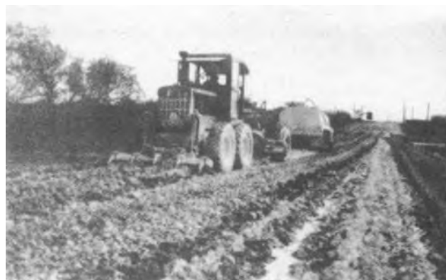
Figure 4-33. Grader-scarifier cutting slurry into stone base.
