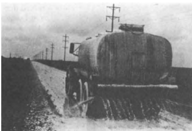
Figure 4-31. Spreading of lime slurry.
