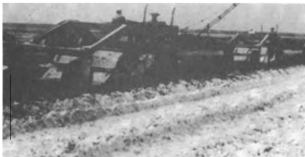
Figure 4-38. Train of rotary mixers.
