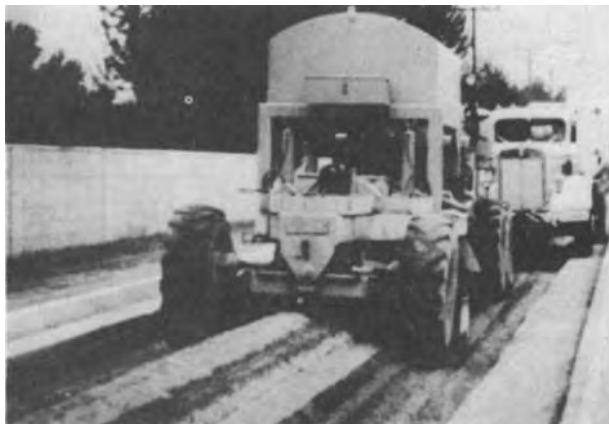
Figure 4-3. Windrow-type traveling pugmill mixing soil-cement from windrows of soil material.
