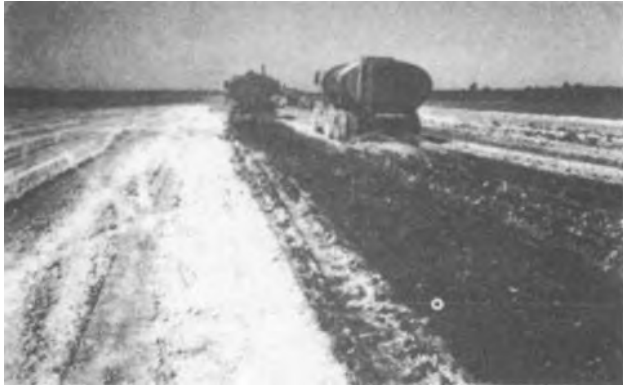
Figure 4-35. Watering of lime-treated clay on airport project.
