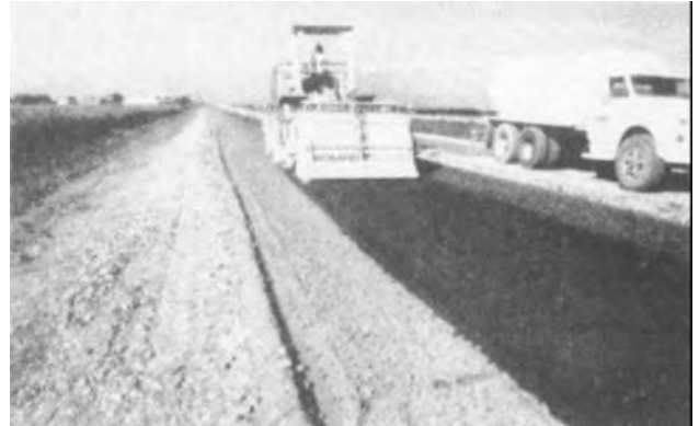
Figure 4-39. Rotary mixer on primary road project.
