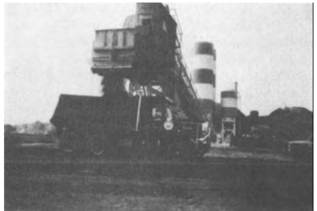
Figure 4-21. Lime-cement-fly ash aggregate base course.
