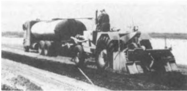
Figure 4-48. Single-shaft rotary mixer with asphalt supply tank.
