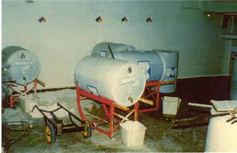
Figure 8-3 **Automatic Chemical Feed System**
