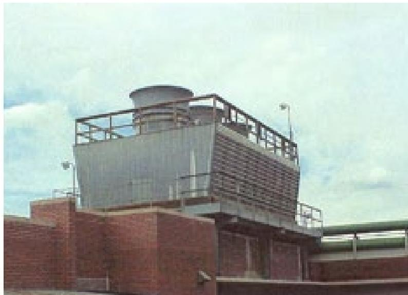
Figure 5-8 Counter-Flow Cooling Tower Diagram
