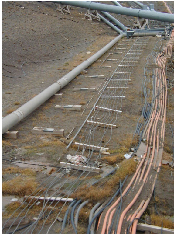
Figure 2-1 Unprotected Insulated Power Lines at Thule Air Base, Greenland
