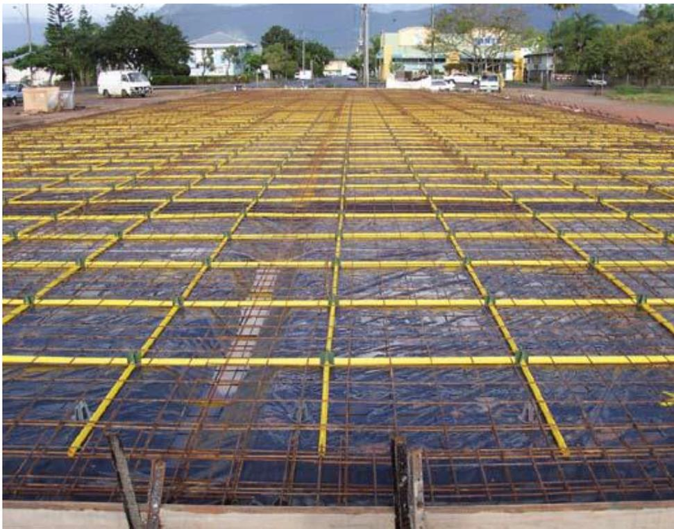
Figure 6-8 Crack-Inducer Tubes
