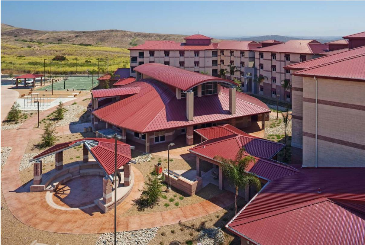
Building design and site design: Example of using shading structures for outdoor gathering spaces, deep overhang to provide shade and shadow and minimize heat gain in Summer time, walkway connecting all elements of projects to each other, enhanced paving materials at important nodes in the circulation paths. Note site planning and building design to offer optimum views to all rooms in the UH.
