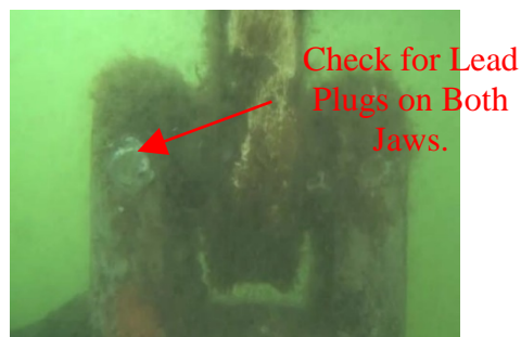
Figure 3-37 Lead Plugs in Riser Swivel Shackle Jaw
