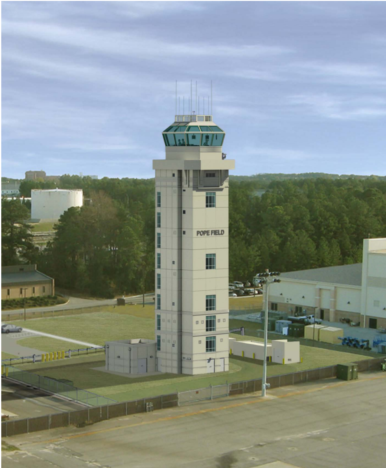
Figure 2-5 ATCT Functional Shaft without Support Building
