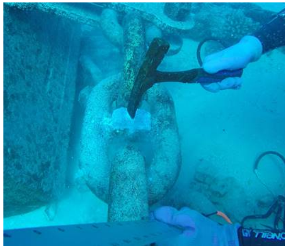
Figure 3-51 Tapping the Zinc Anode
