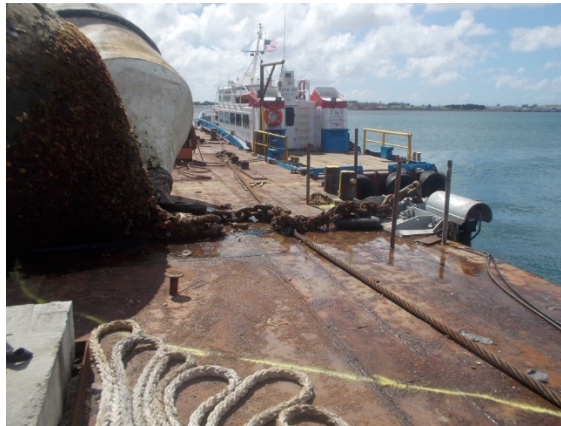
Figure 5-2 Mooring Riser Secured into a CCD
