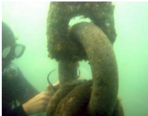
Figure 3-44 Ground Ring Assembly
