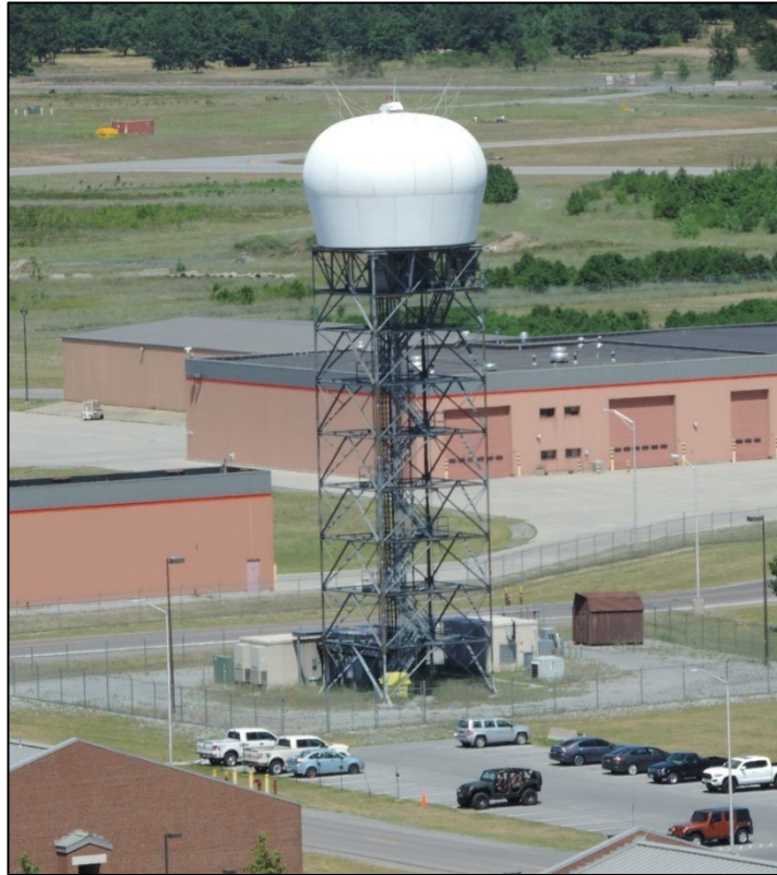
Figure 5-3 Typical DASR without Antenna Cover (Army)
