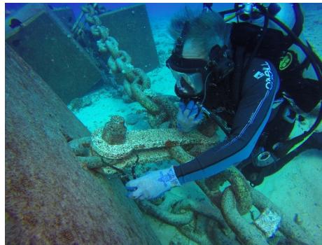
Figure 2-39 Plate Shackle Attaching Sinkers to Chain
