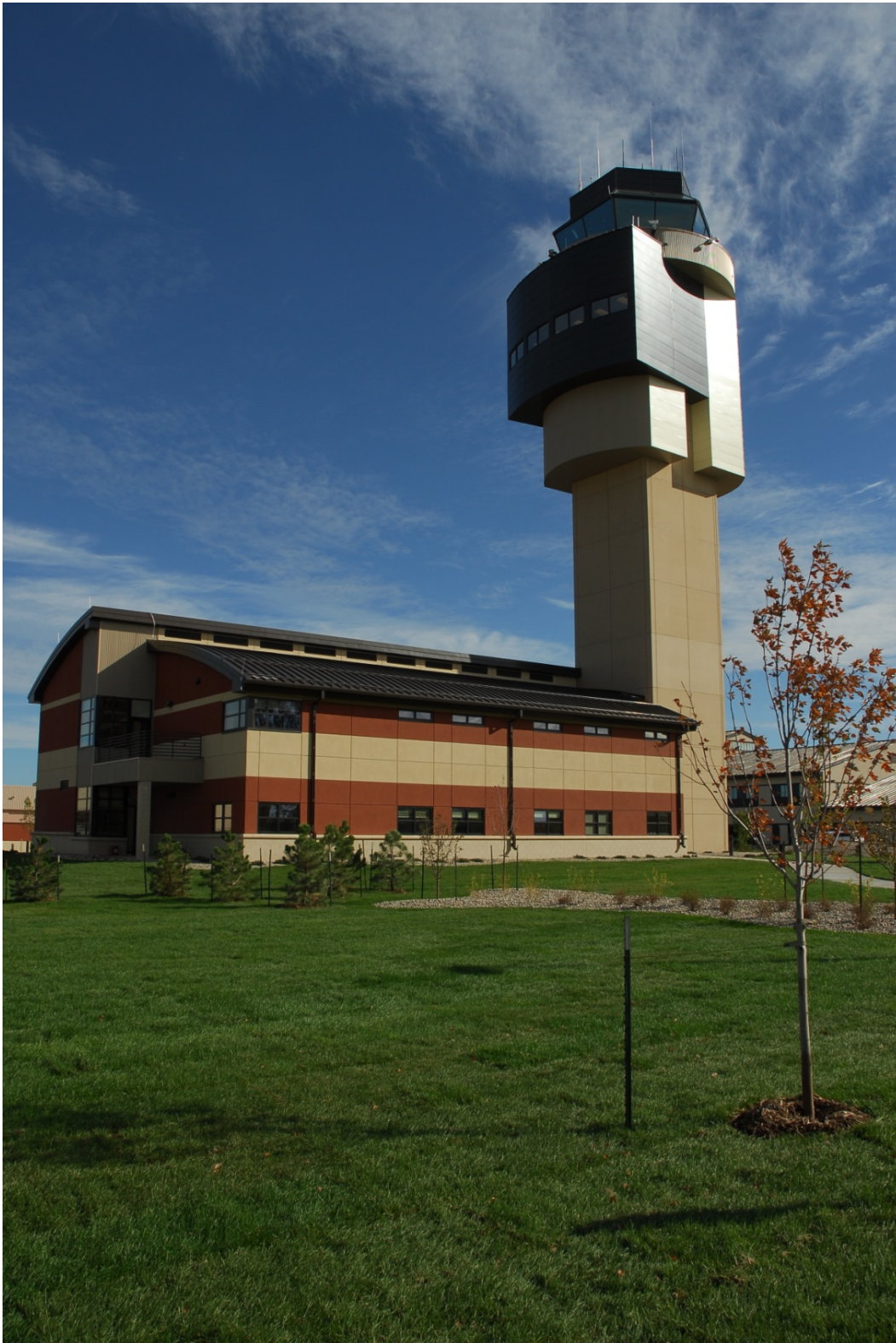
Figure 2-4 ATCT Non-Functional Shaft with Support Building
