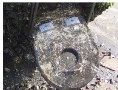
Figure 2-51 Chain Stud Anode on Buoy Tension Bar
