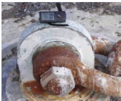
Figure 3-27 Minimal Corrosion on Tension Bar Padeye
