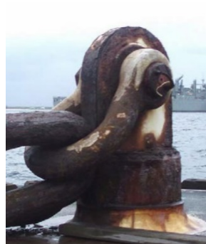
Figure 3-28 Excessive Corrosion on Tension Bar Padeye
