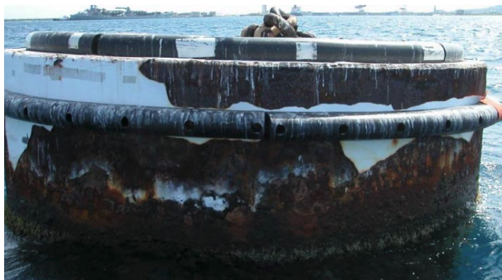
Figure 3-30 Outer Coating Loss on Steel Buoy
