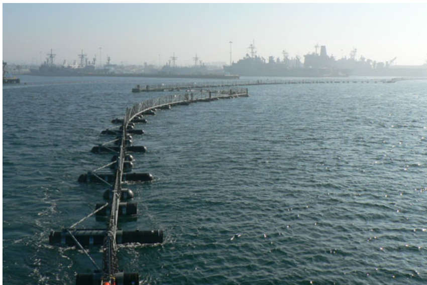
Figure 5-2 Boat Barrier System (Port Security Barrier)
