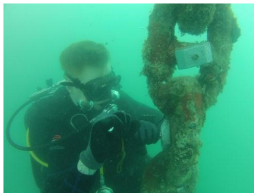
Figure 3-54 Diver Attaching Anode to Chain
