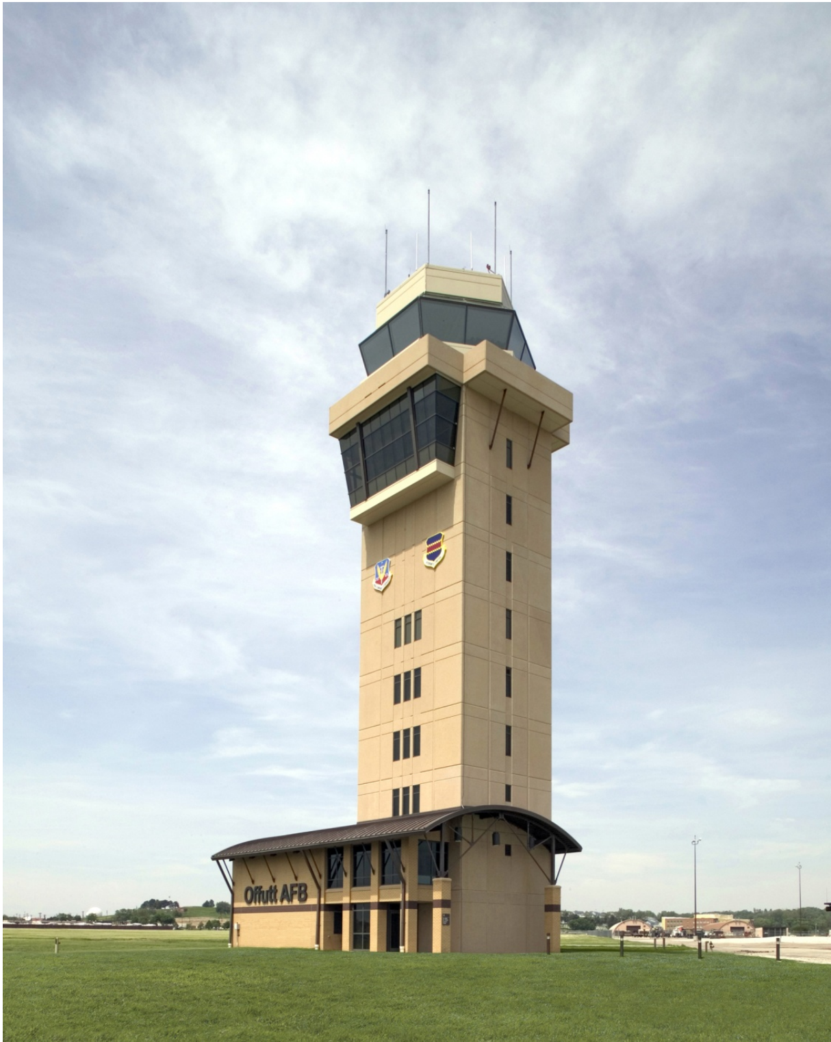
Figure 2-6 ATCT Functional Shaft with Support Building
