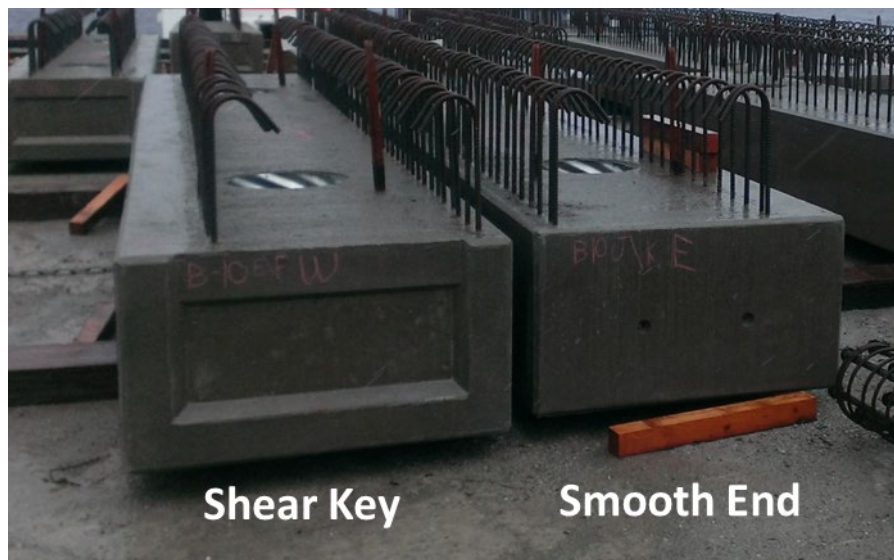
Precast Pile Cap Showing End Configurations
