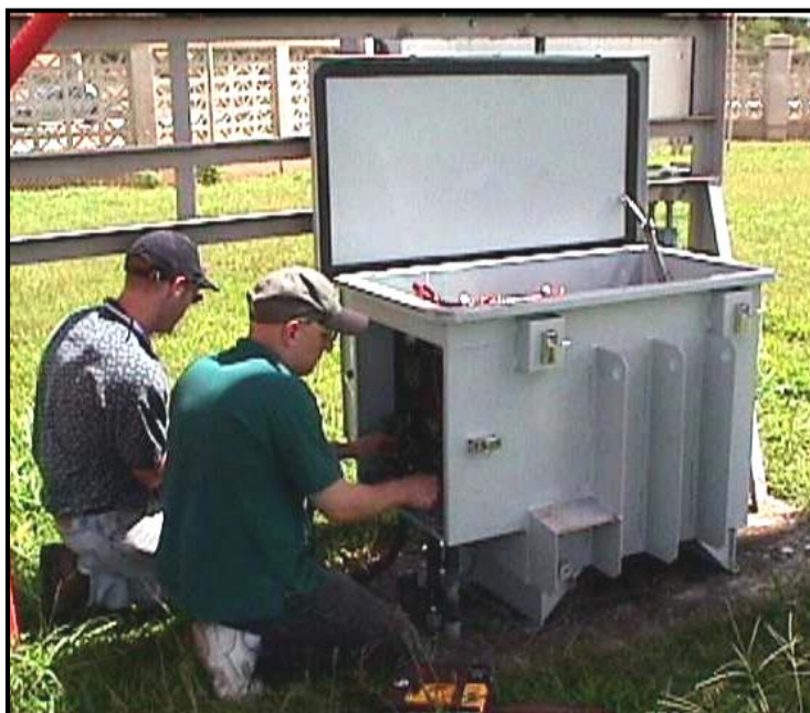
Figure B-12 Rectifiers Located for Ease of Maintenance. .
