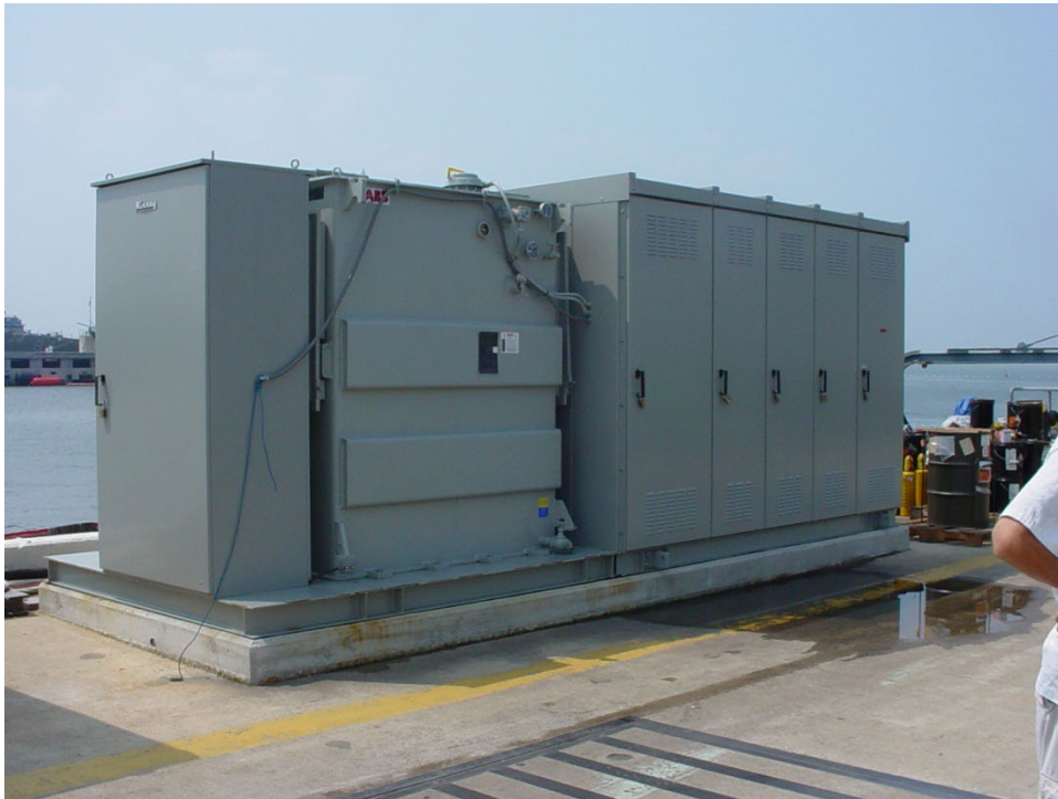
Figure 12-5. Skid-Mounted Substation with Single-Pole Connections
