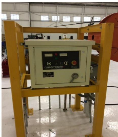
Figure 3-2 Recent Converter Installations (400Hz & 28 VDC) - Example 2
