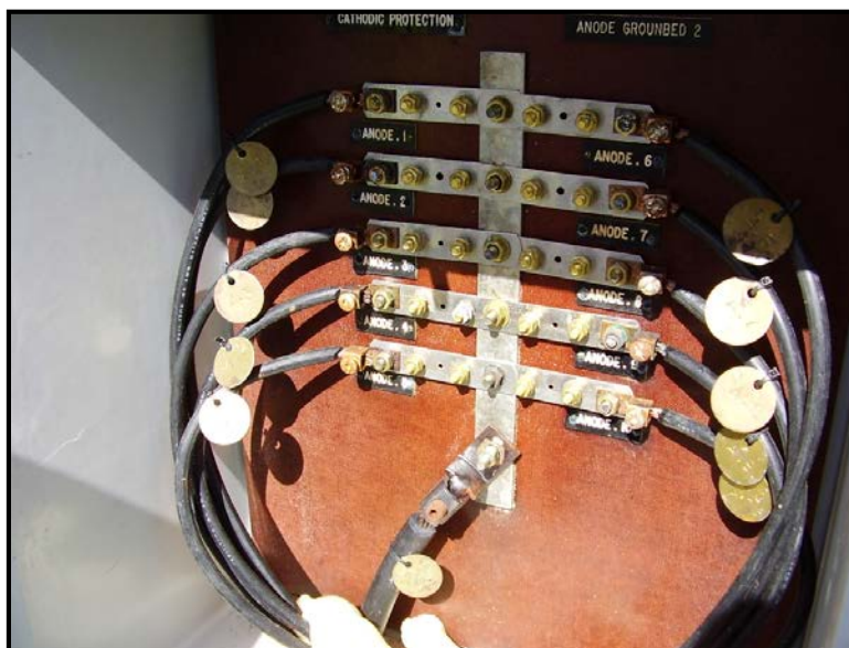
Figure B-18 Anode Junction Box
