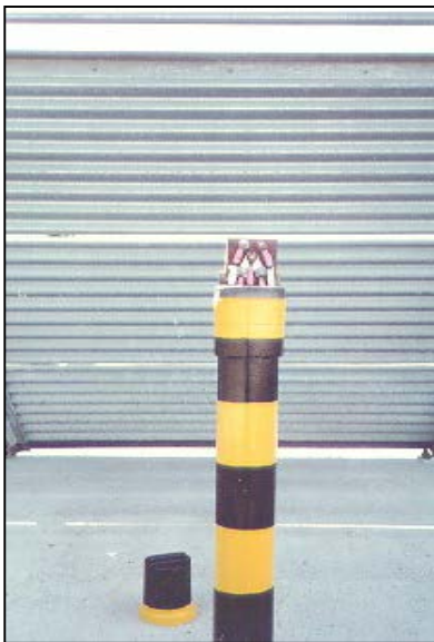
Figure B-7 Above Grade Test Stations. PVC Pipe Mount on the Left, Pole Mount in the Center, and Wall Mount on the Right.
