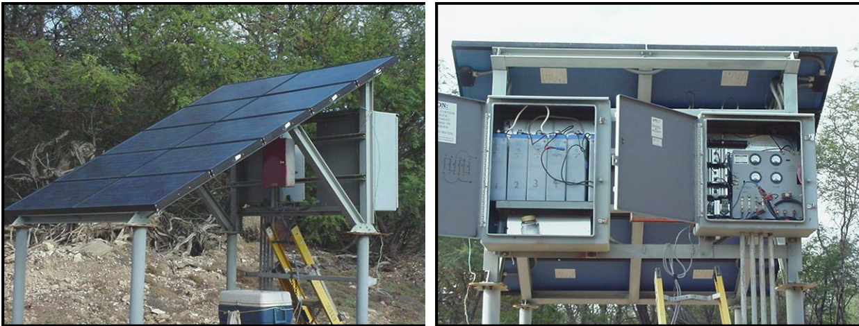
Figure 4-2 Small Solar Powered CP System. Solar Panels Shown in Picture on Left. Battery Bank and Control Center Shown on Right.
