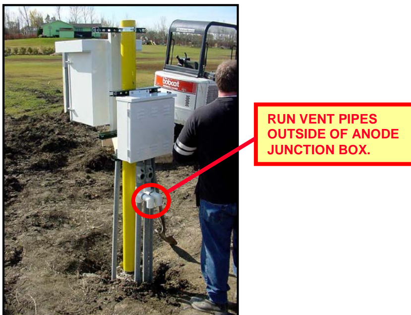
Figure B-23 Anode Column Vent Pipes Run Outside of Anode Junction Box.
