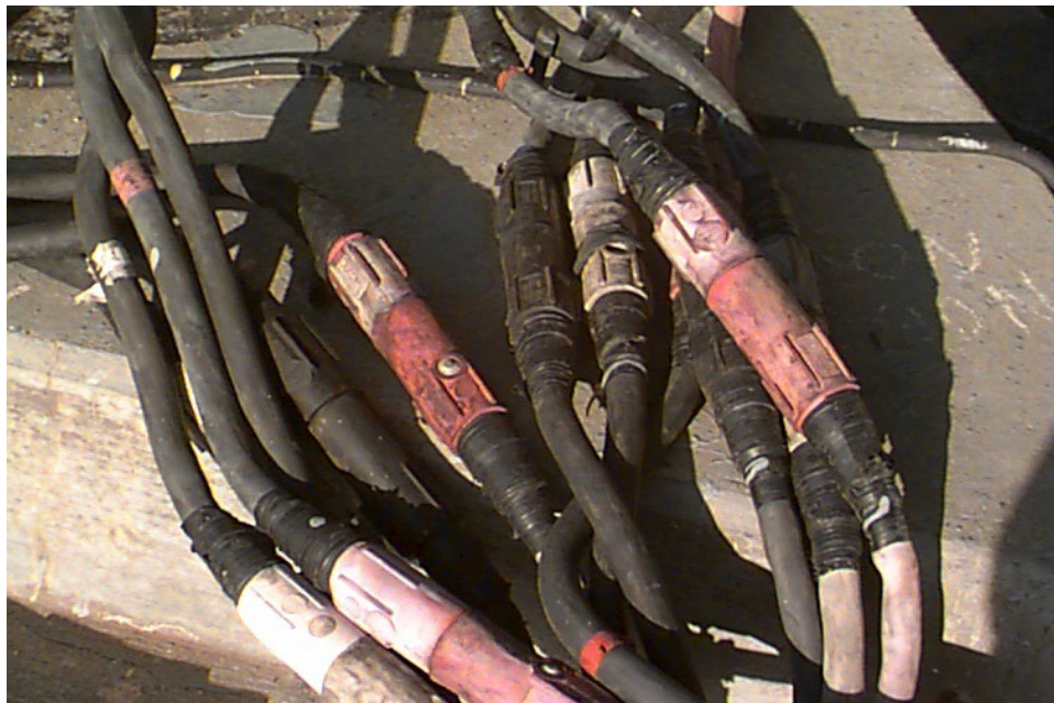
Figure 12-12. 480 Volt Shore-Cable to Ship-Cable Plug and Receptacle Connection In Place
