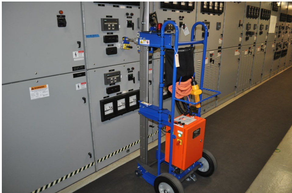
Figure 1. Remote Racking Mechanism
