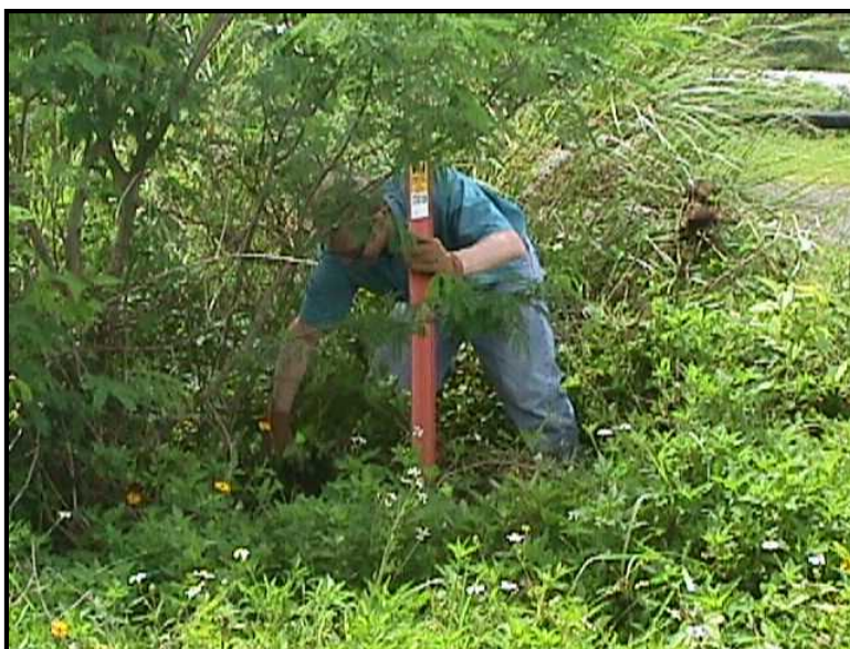
Figure B-13 Test Station Marker for Flush Mount Test Station.
