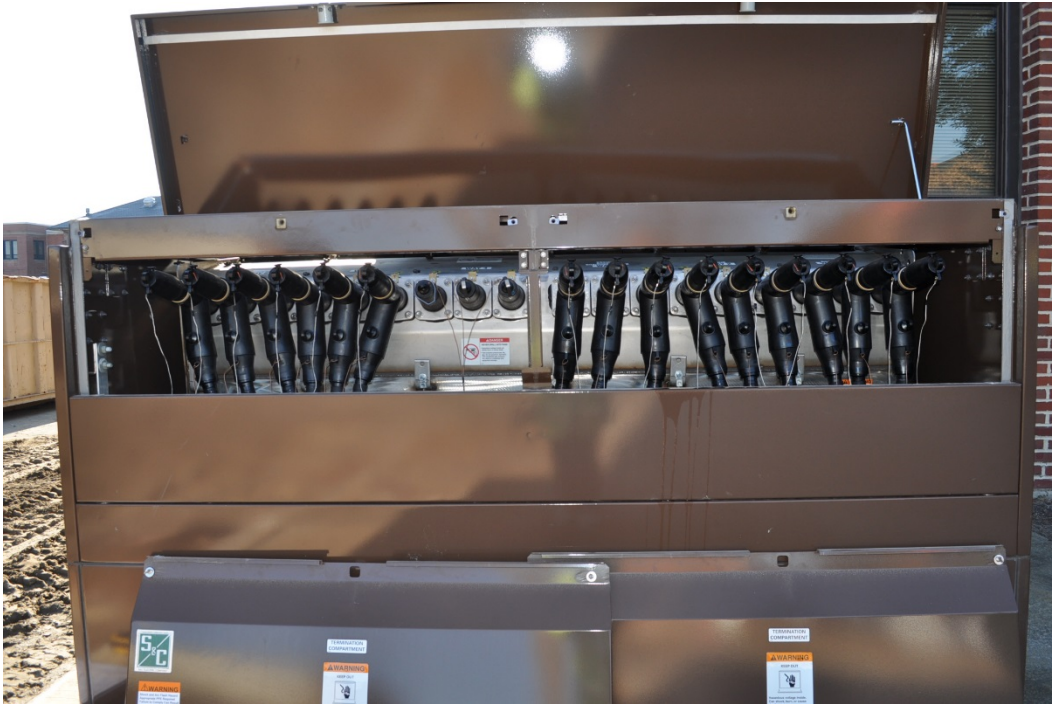
Figure D-1 S&C Vista Switchgear
