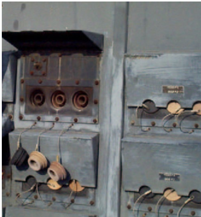
Figure 12-5. Skid-Mounted Substation with Single-Pole Connections
