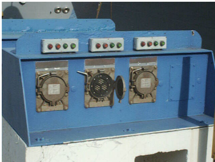
Figure 12-8. 4.16 kV Pier Electrical Outlet Assembly and Outlets – Existing Installations
