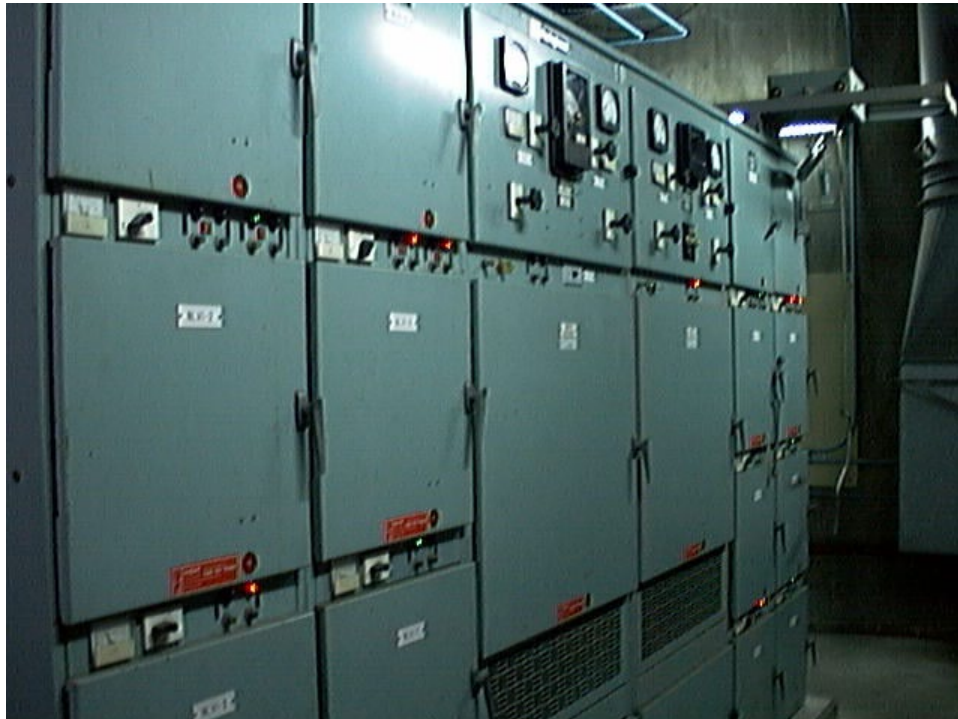
Figure 12-3. Inside a Pier Vault Housing a Substation
