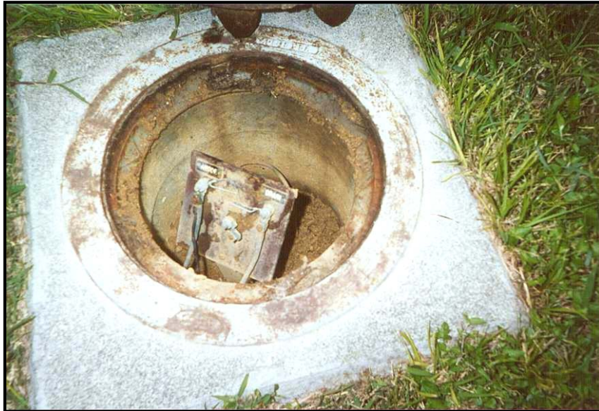
Figure B-9 Flush Mounted Current-Potential Test Station
