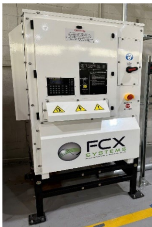
Figure 3-3 - Recent Converter Installations (270 VDC & 400 Hz) – Example 3
