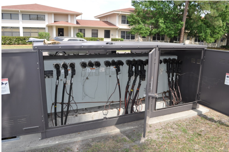
Figure D-2 G&W VFI Switchgear
