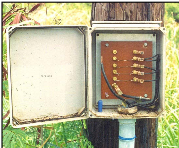
Figure B-11 Wall/Pole Mount Type Test Station.
