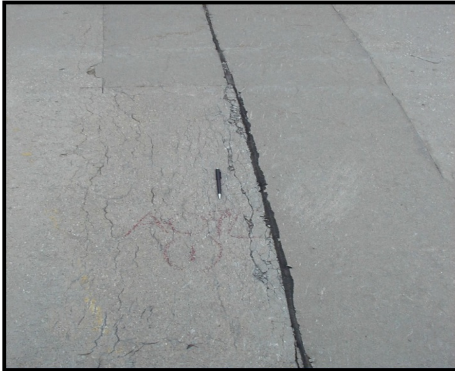
Figure B-14 High-Severity “D” Cracking
