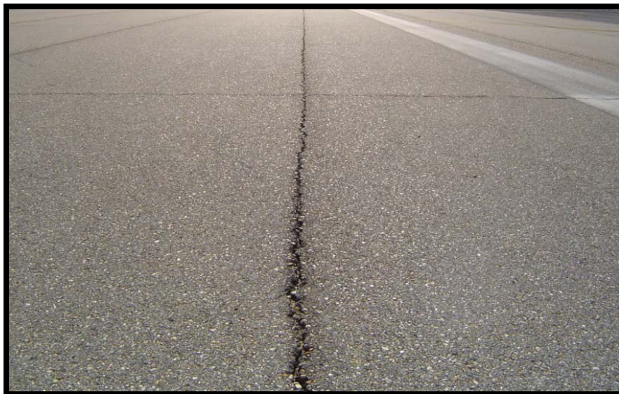
Figure A-21 Low-Severity Joint Reflection Cracking
