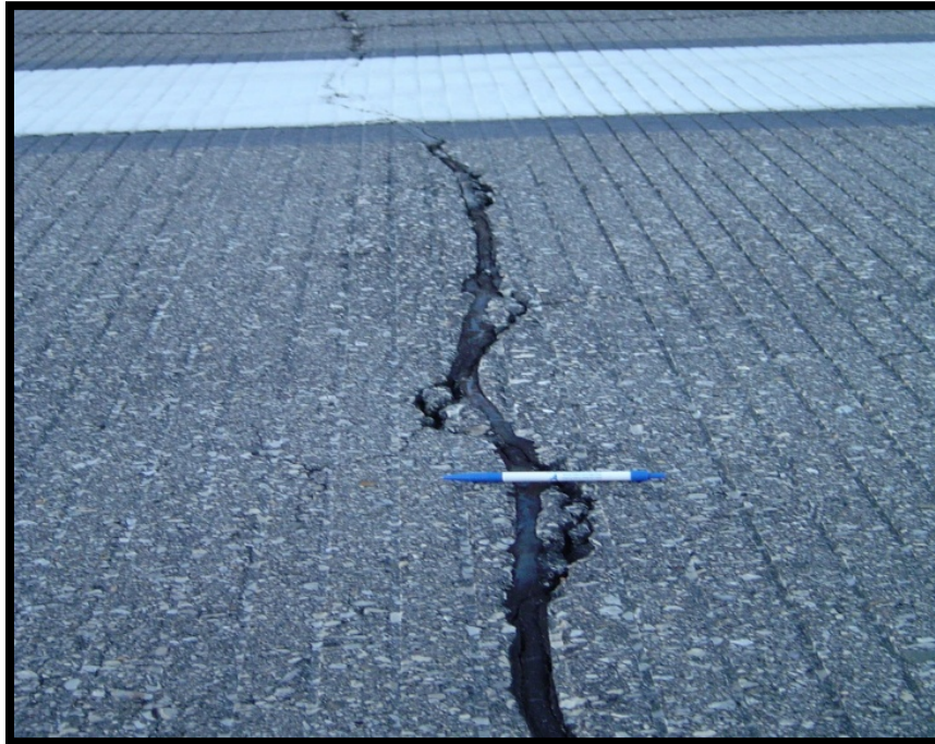
Figure A-26 High-Severity L&T Cracking
