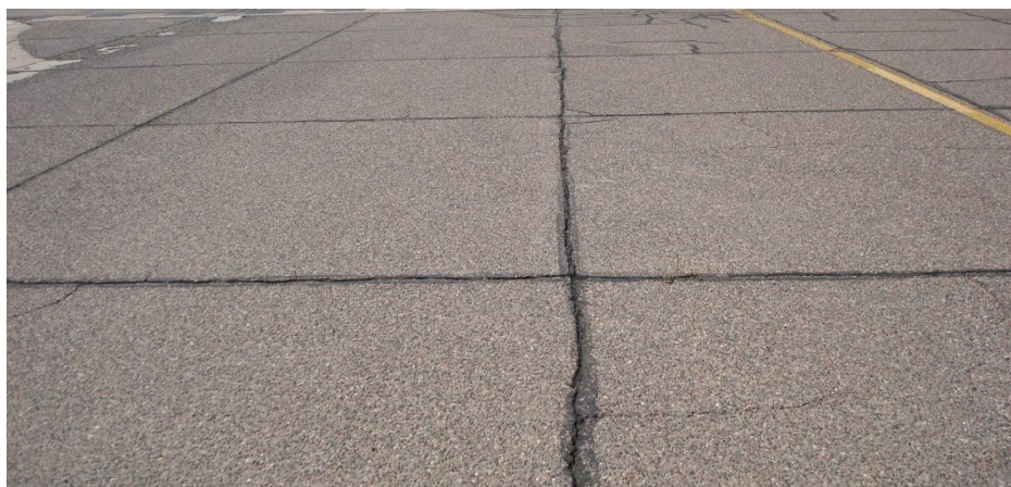
Figure 3-3 Reflective Cracking
