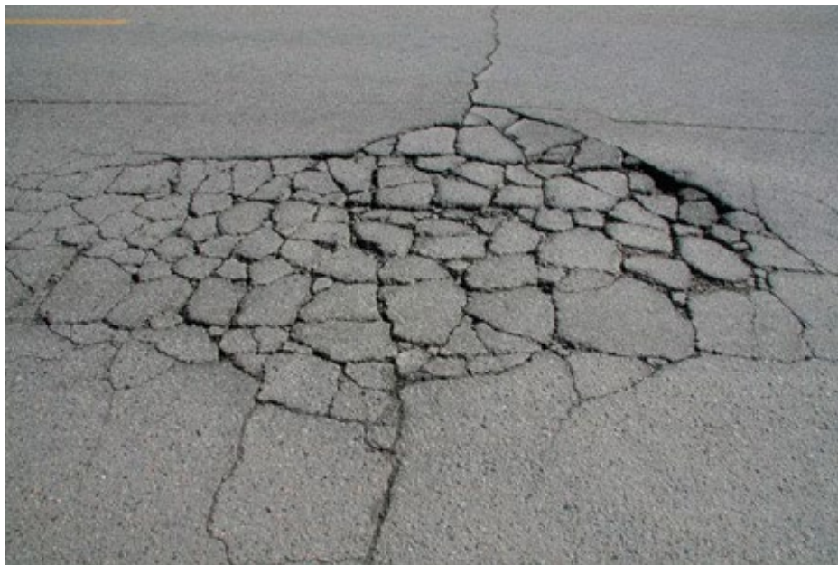
Figure 9-1 Alligator Cracking
