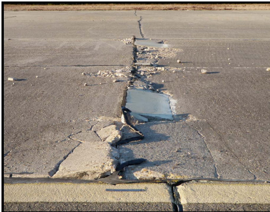
Figure B-4 High-Severity Blowup
