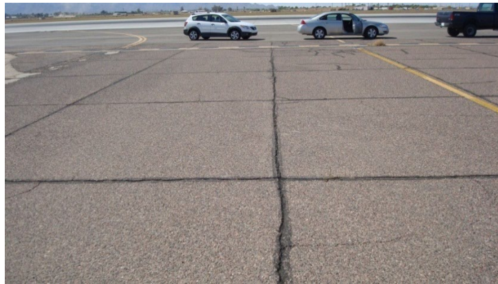
Figure 9-3 Longitudinal Cracking
