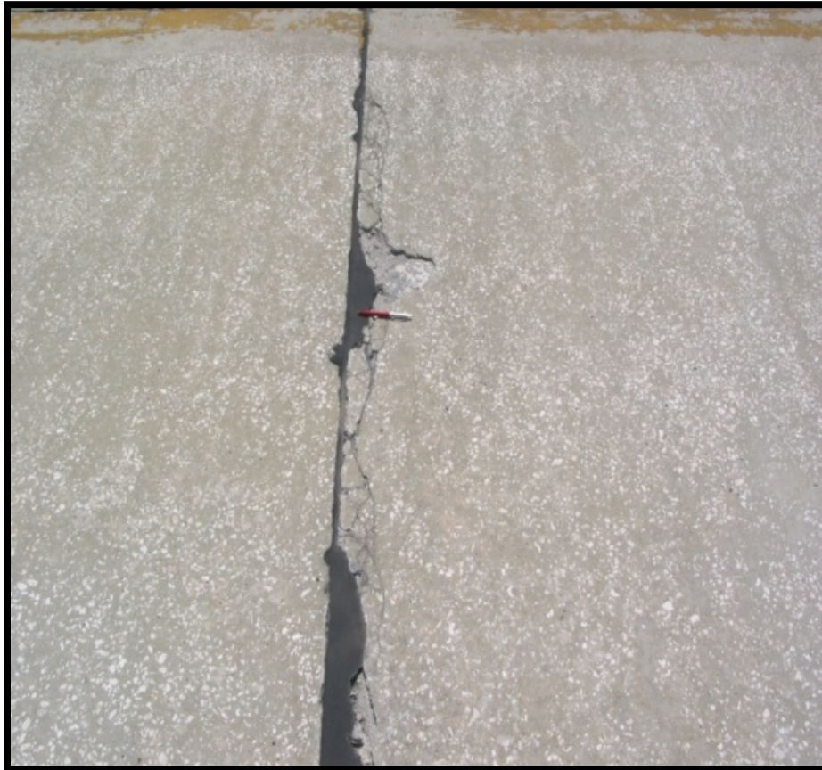
Figure B-40 High-Severity Joint Spall
