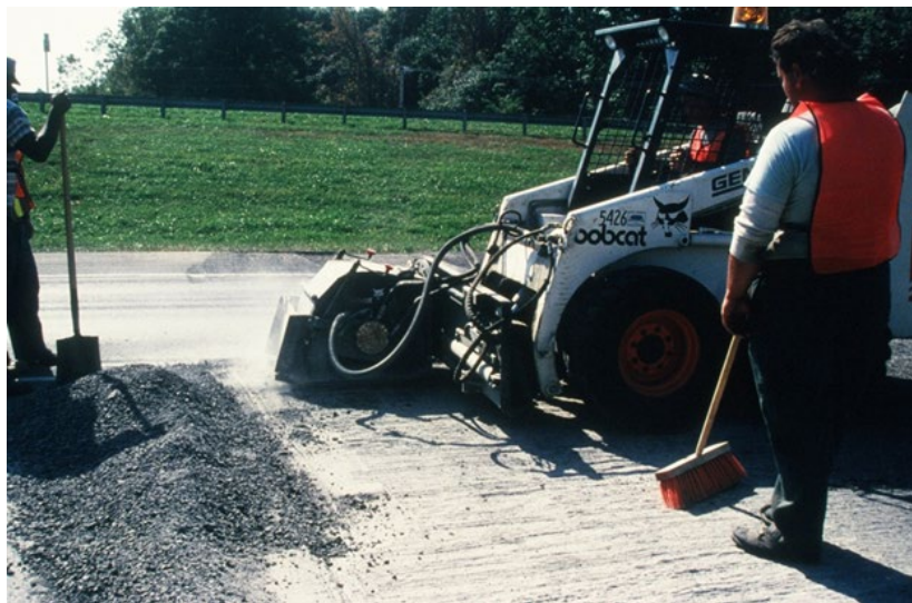
Figure 3-4 Small Milling Head Attachment
