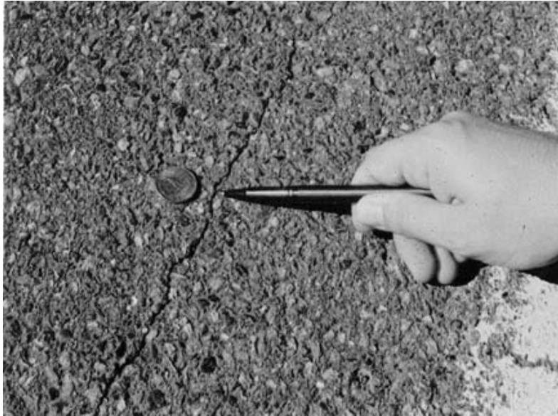
Figure 9-5 Small Crack
