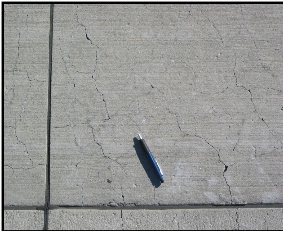
Figure B-45 Medium-Severity ASR
