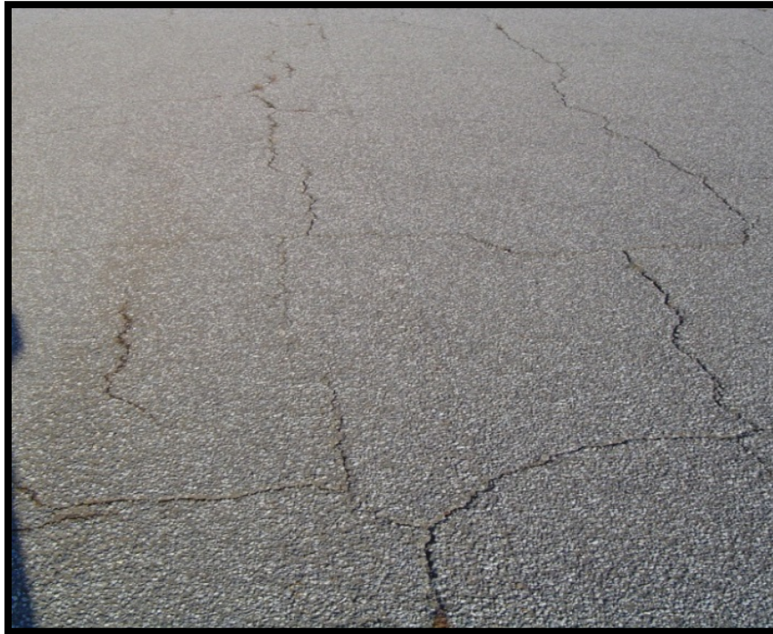
Figure A-10 High-Severity Block Cracking
