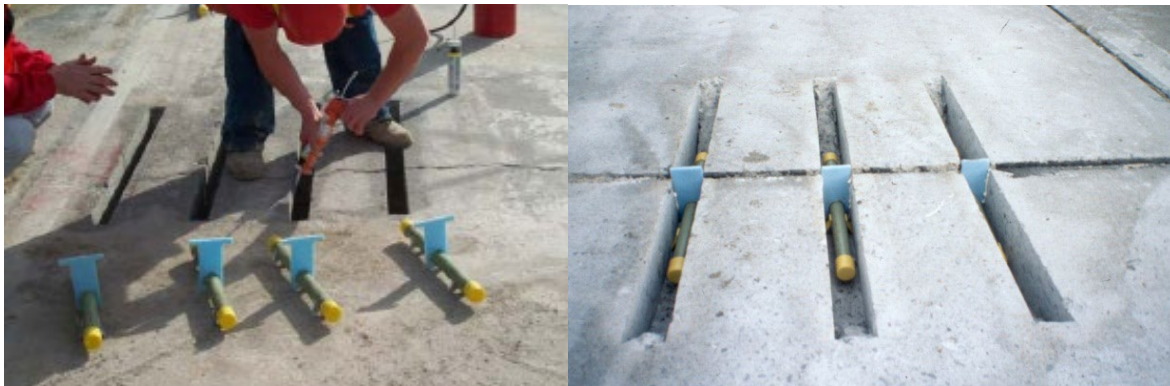
Figure 18-6 Use of Compressible Insert
