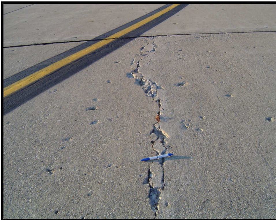
Figure B-10 High-Severity Linear Cracks
