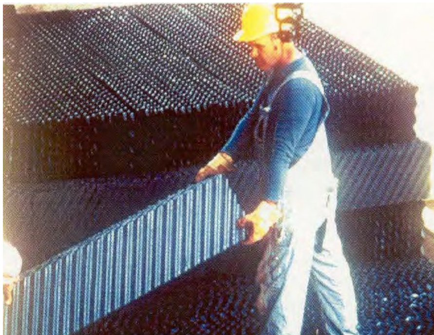
Figure 5-11 High-Efficiency Cooling Tower Film Fill
