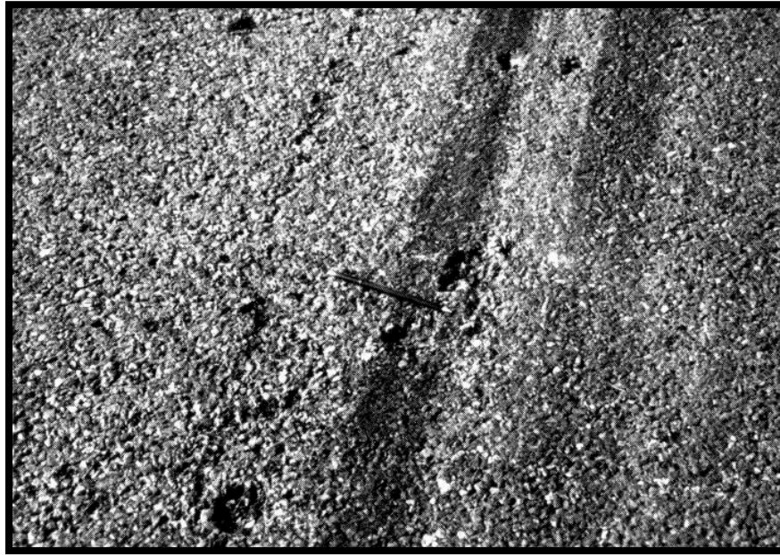
Figure A-45 High-Severity Raveling (PFC)
