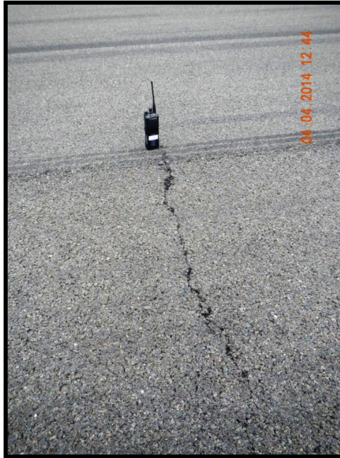
Figure A-29 Medium-Severity PFC L&T Cracking
