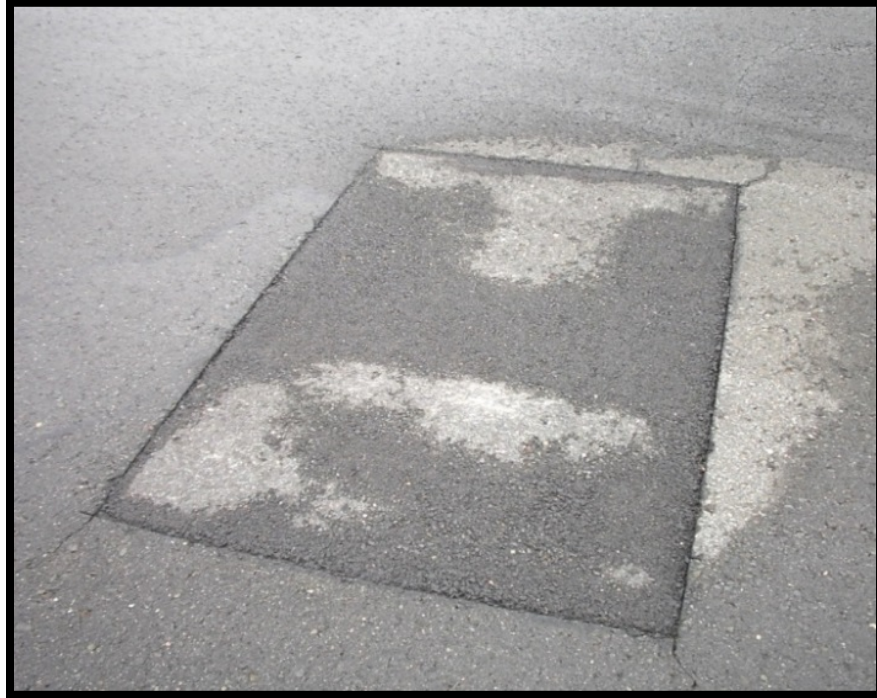
Figure A-33 Medium-Severity Patching
