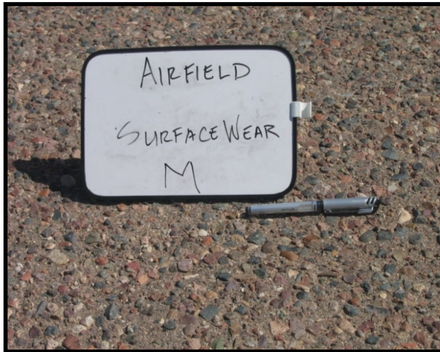
Figure A-56 High-Severity Weathering
