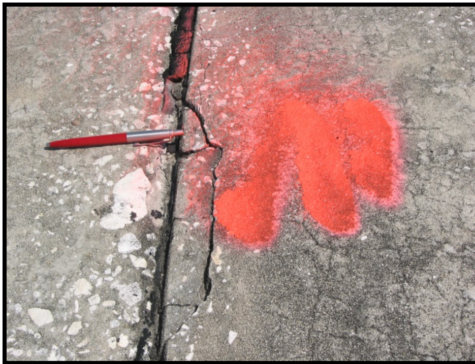
Figure B-38 Medium-Severity Joint Spall
