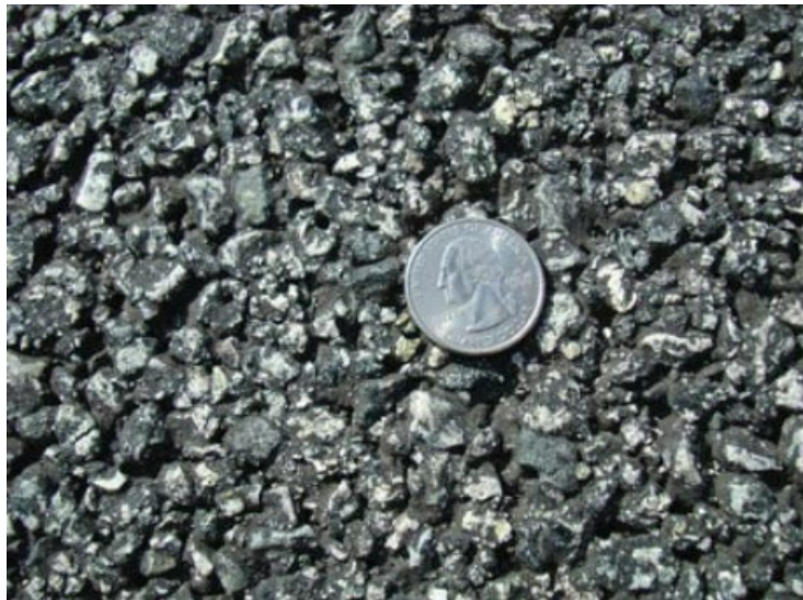
Figure 10-1 View of a Porous Friction Surface (PFS)
