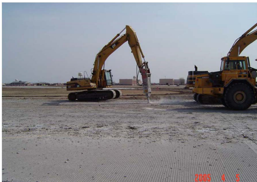
Figure 6-10 Excavator W/Hydraulic Impact Hammer (Ram Hoe) Attachment*
