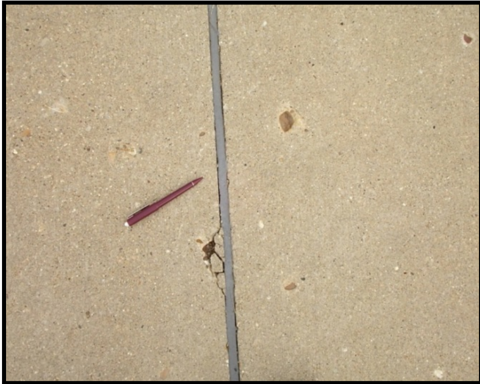
Figure B-38 Medium-Severity Joint Spall
