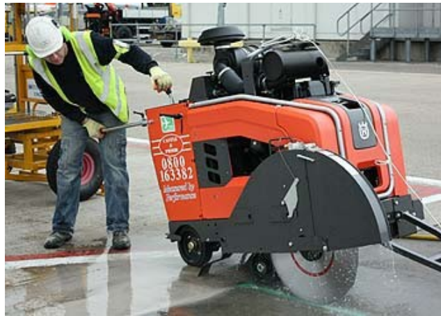
Figure 14-3 Diamond Blade Sawing
