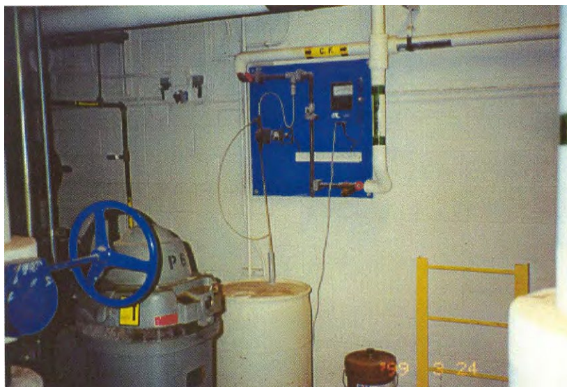
Figure 8-4 Automatic Neat Chemical Feed
