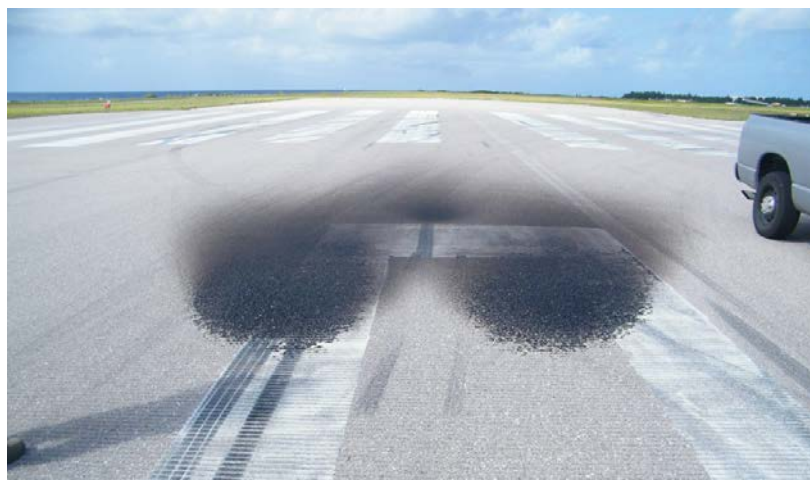
Figure 3-2 Jet Blast Damage
