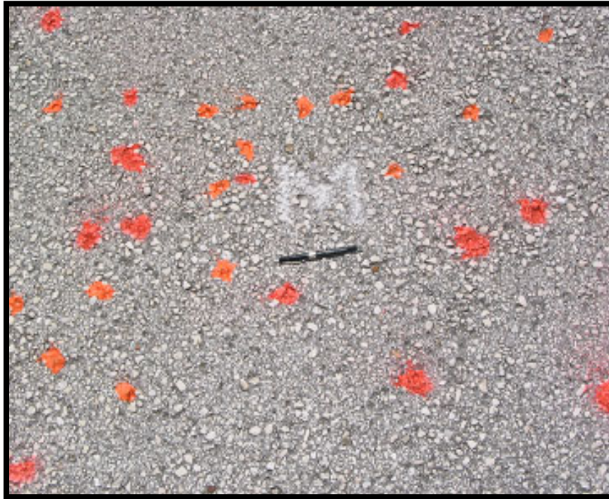
Figure A-38 High-Severity Raveling (Dense Mix)
