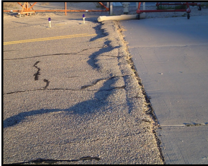
Figure A-49 High-Severity Shoving
