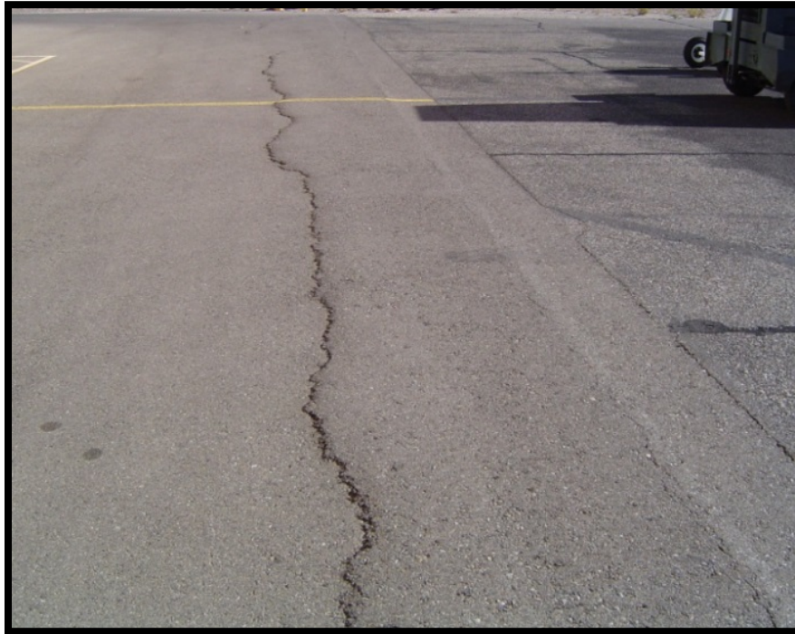
Figure A-48 Medium-Severity Shoving
