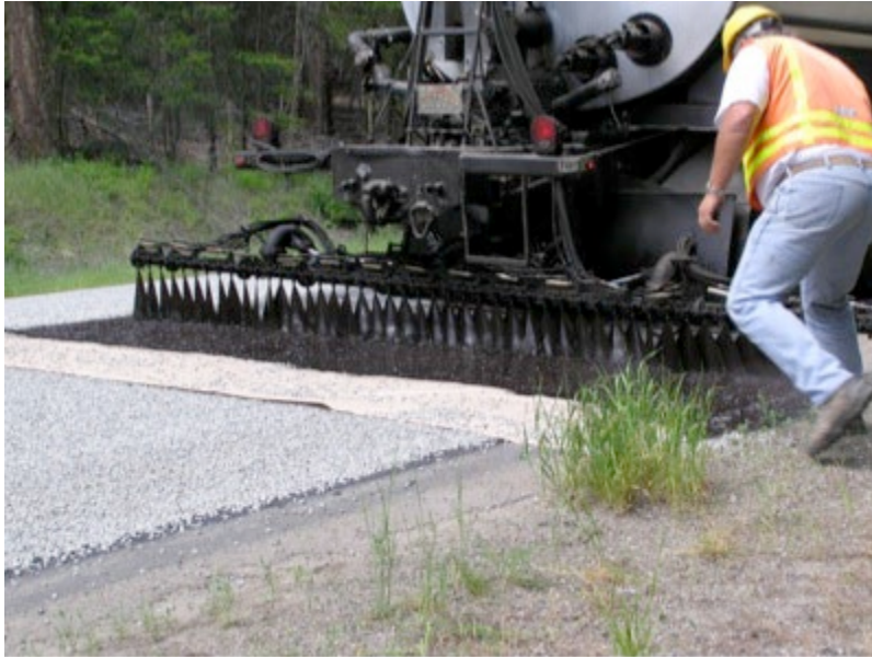
Figure 6-3 Use Paper for Straight Edge
