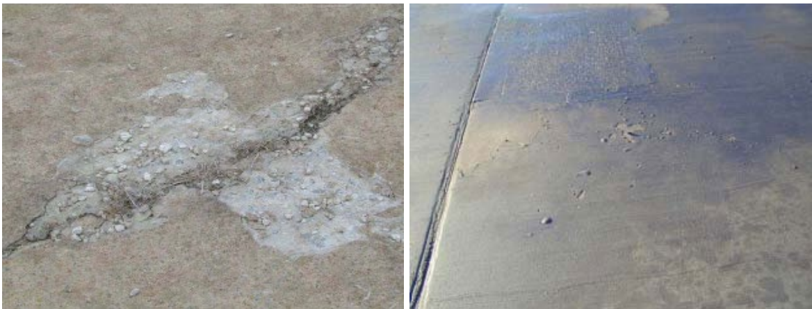
Spalling and Scaling
