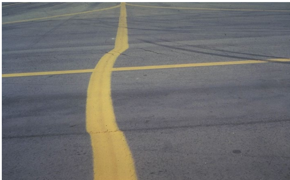
Figure 3-10 Slippage due to Loss of Bond
