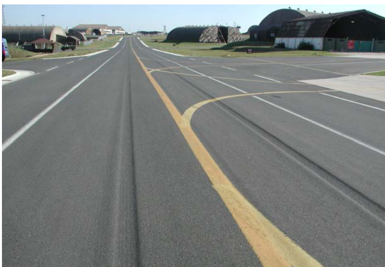
Figure 3-9 Rutting in the HMA Layers
