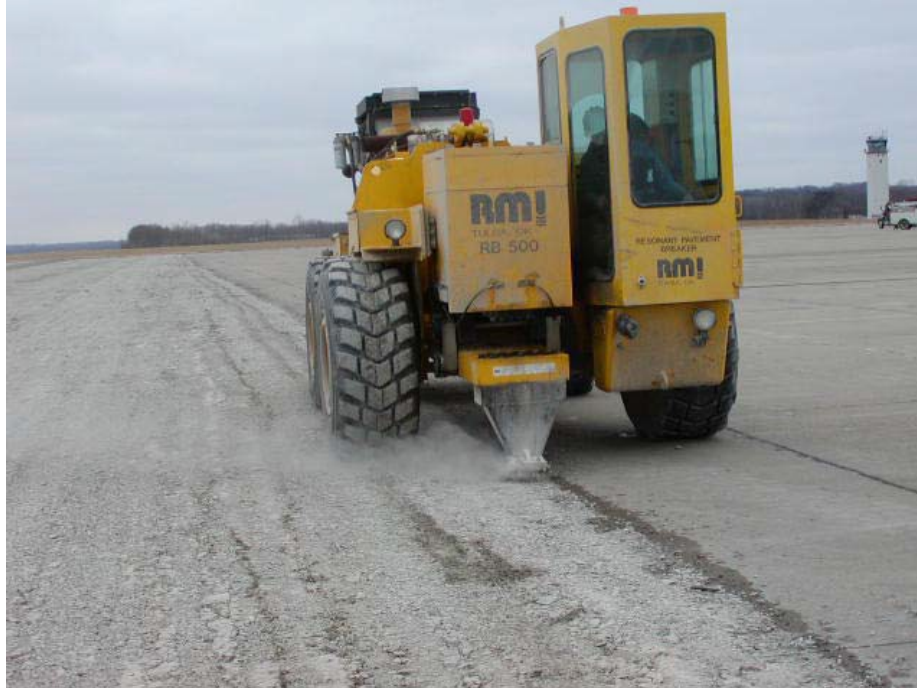
Figure 6-6 Rubblization Using RPB*
