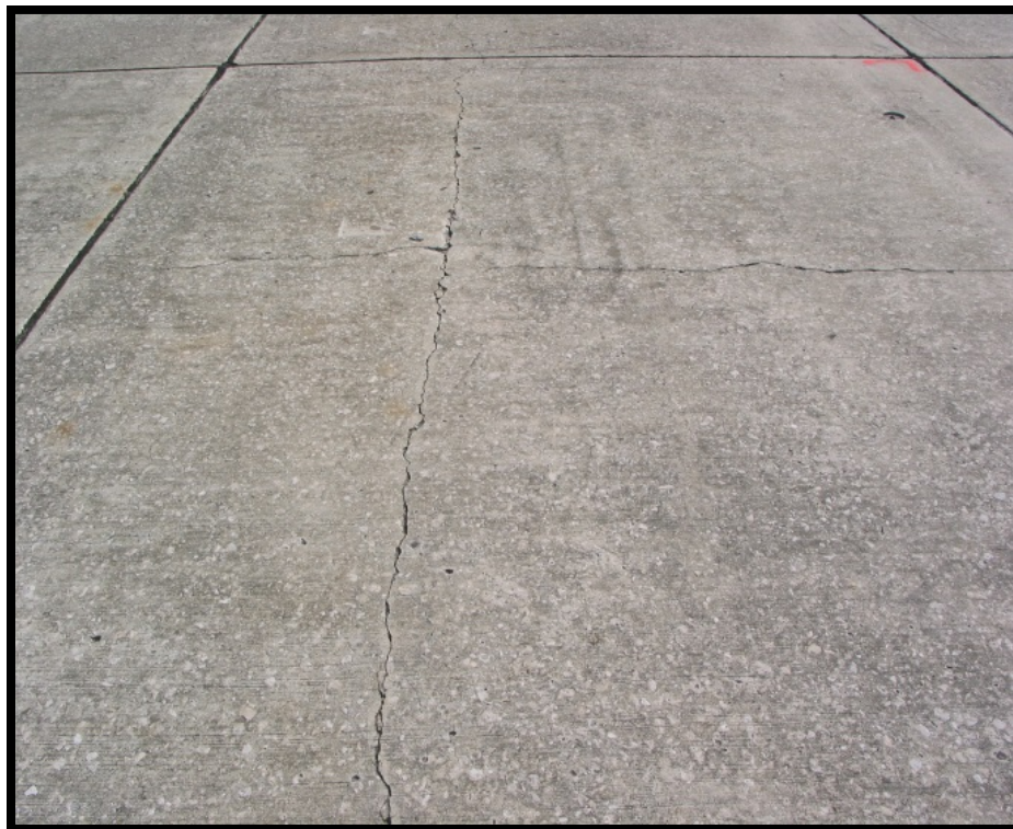
Figure B-33 Low-Severity Shattered Slab/Intersecting Cracks
