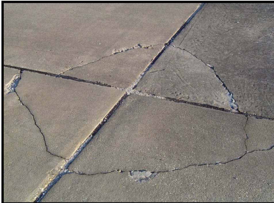
Figure B-6 Medium-Severity Corner Break
