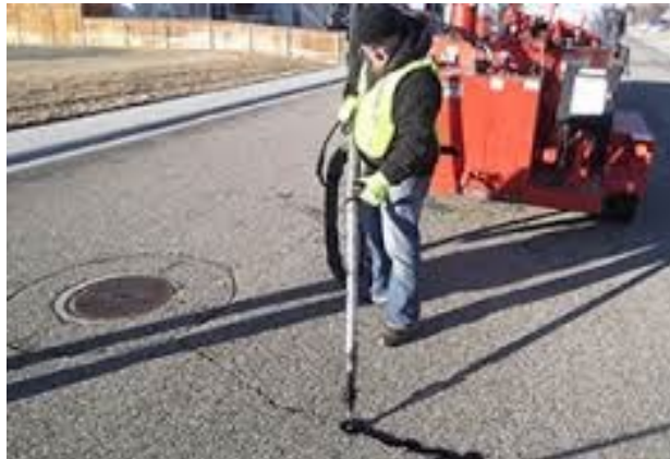
Figure 9-9 Filling Crack with Sand Emulsion Mixture
