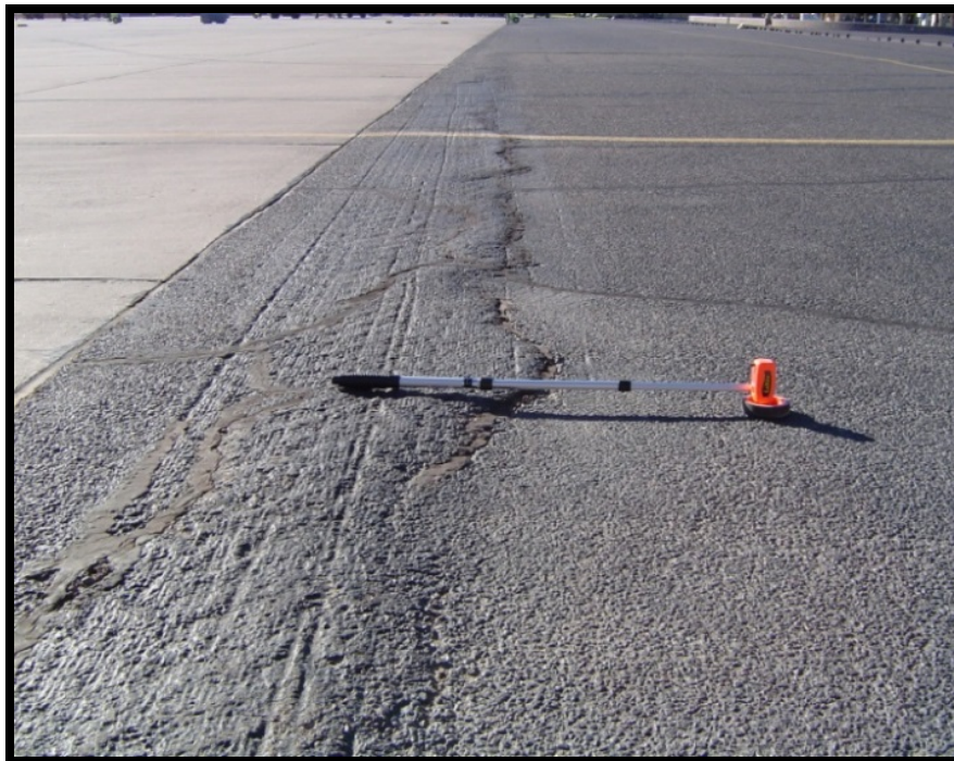
Figure A-48 Medium-Severity Shoving
