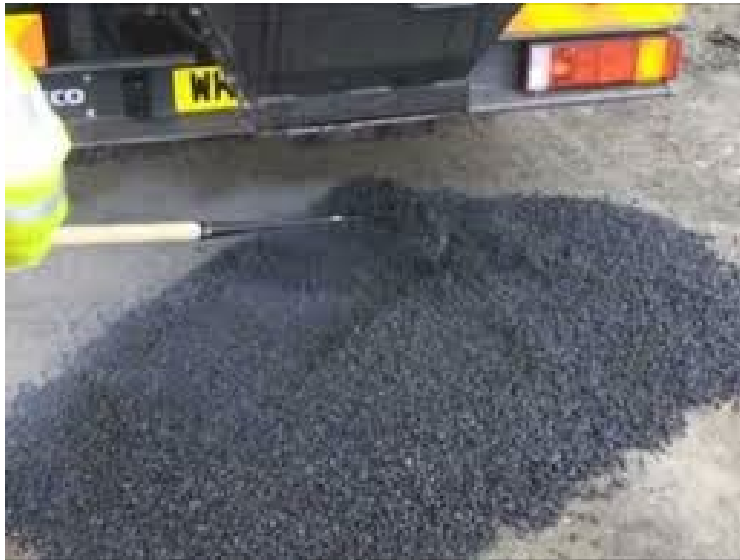
Figure 3-6 Overfill Prior to Compaction
