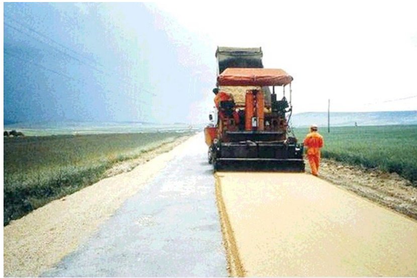
Figure 4-12 Granular Material Added to Achieve Compacted Thickness*
