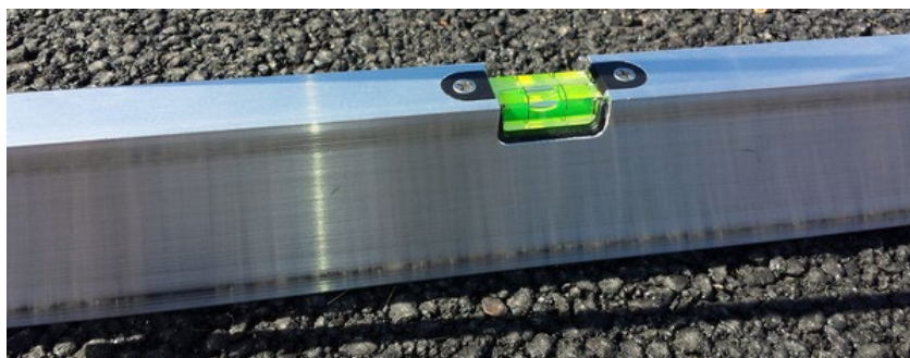
Figure 3-9 Check Level of Patch Surface
