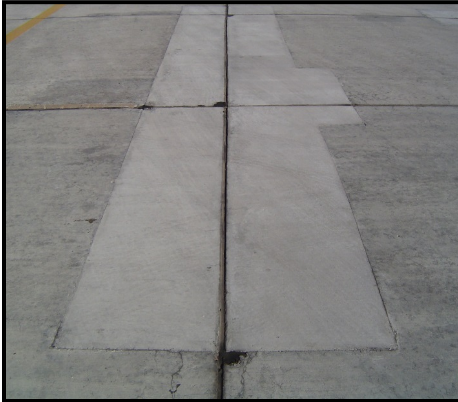
Figure B-22 Medium-Severity Large Patch
