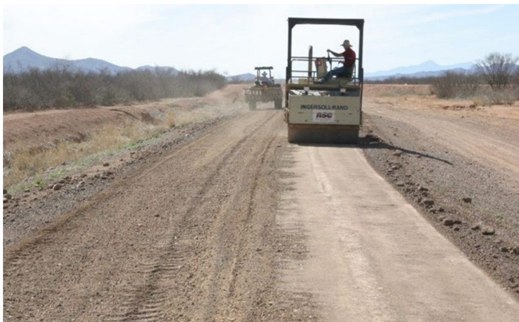
Figure 5-3 Compacting Road Surface After Mixing
