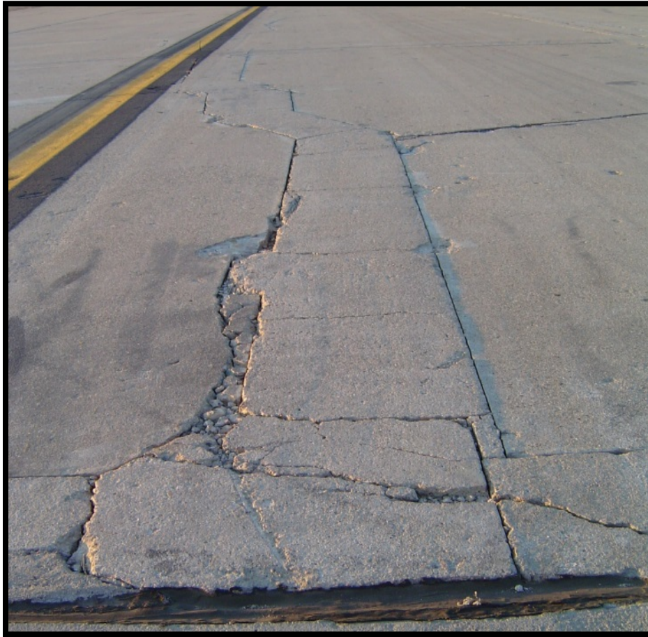
Figure B-23 High Severity Large Patch
