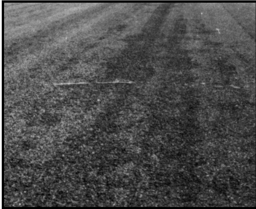
Figure A-44 Medium-Severity Raveling (PFC)
