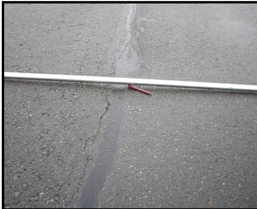
Figure A-16 Low-Severity Depression
