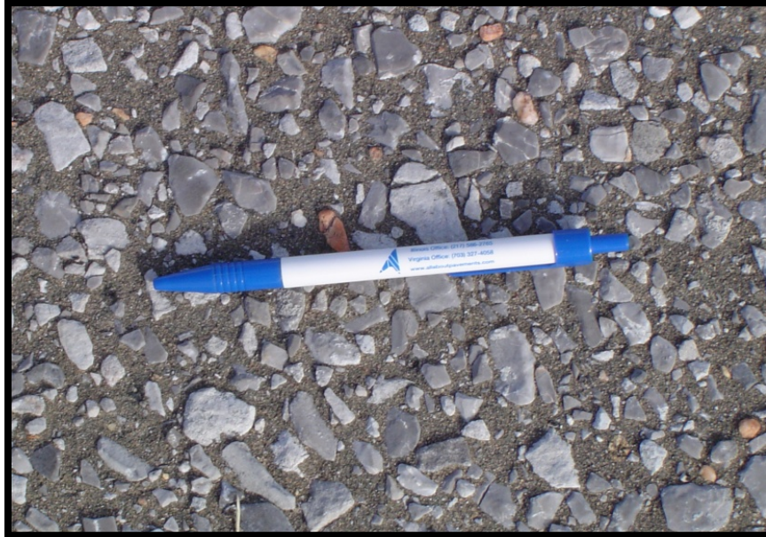
Figure A-35 Polished Aggregate
