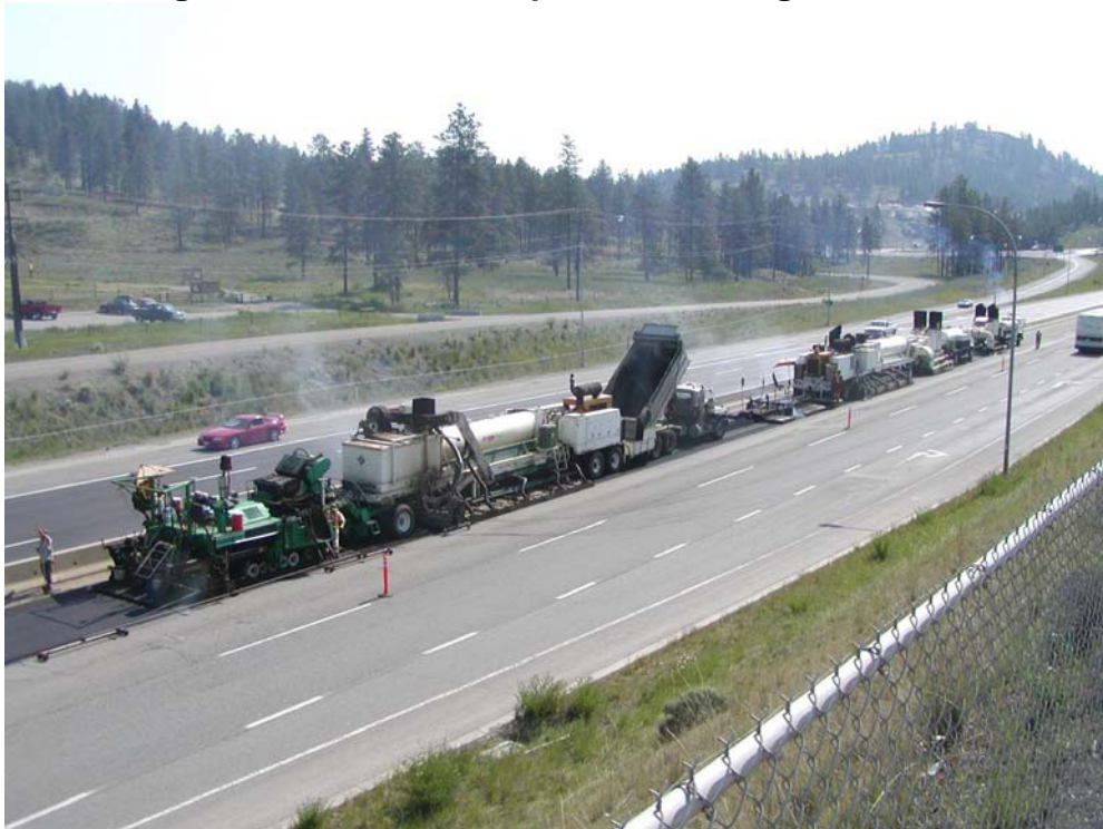
Figure 5-11 Example of Single Stage Remixing Train
