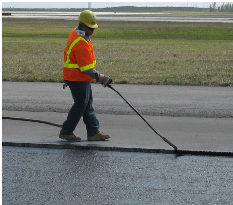
Figure 3-5 Hand-spraying Edge of Cut
