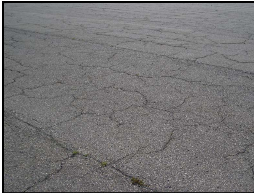
Figure A-10 High-Severity Block Cracking
