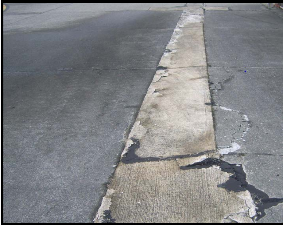
Figure B-2 Low-Severity Blowup
