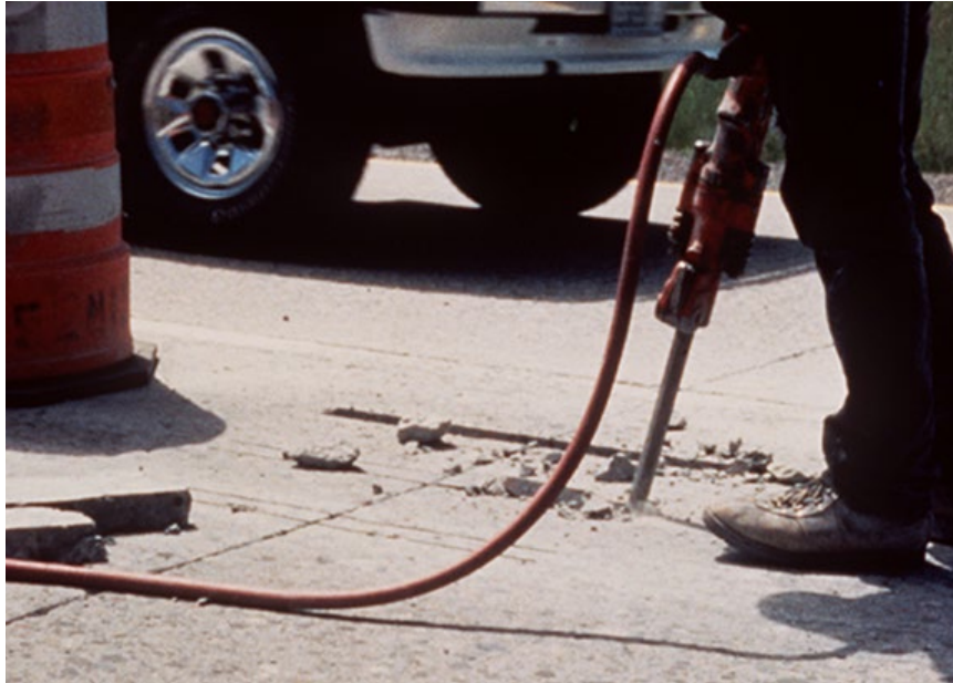
Figure 18-5 Use of Chipping Hammers to Remove Concrete
