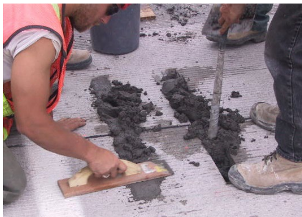
Figure 18-7 Placing and Consolidating Patch Material
