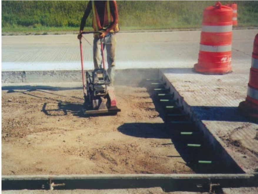
Figure 14-9 Patch Area Compaction
