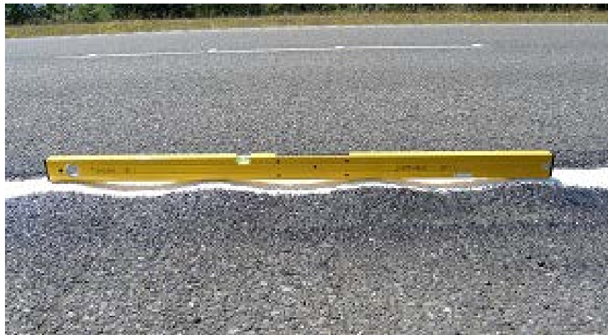
Figure A-14 Medium-Severity Corrugation
