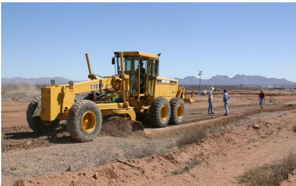
Figure 5-1 Grading Road Surface Prior to Treatment
