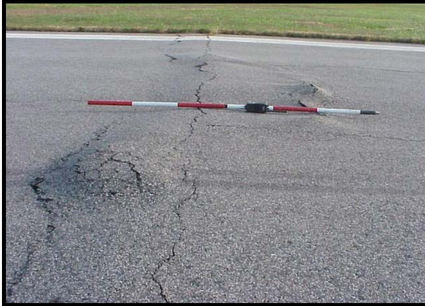
Figure A-53 High-Severity Swell
