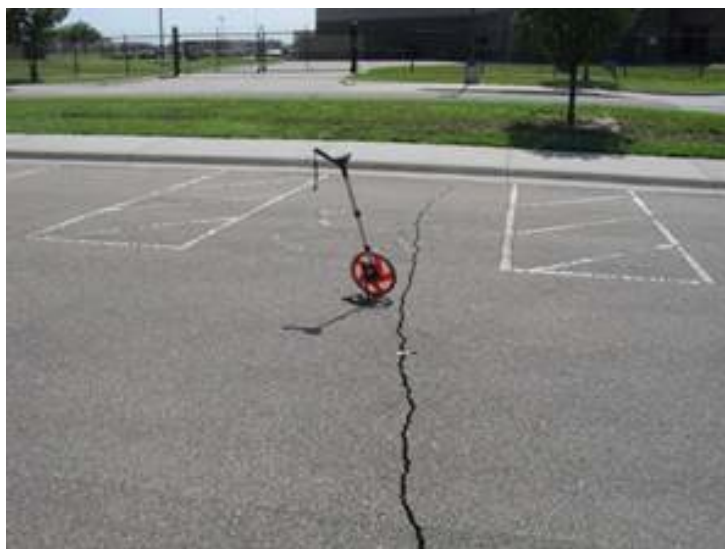
Figure 9-3 Longitudinal Cracking
