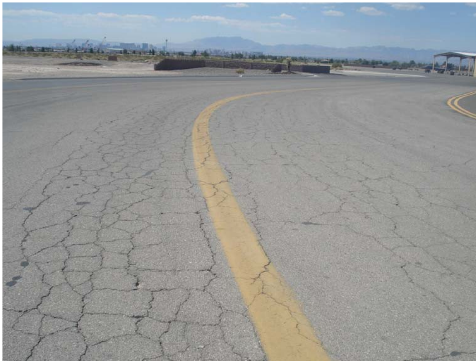
Figure 3-1 Alligator Cracking
