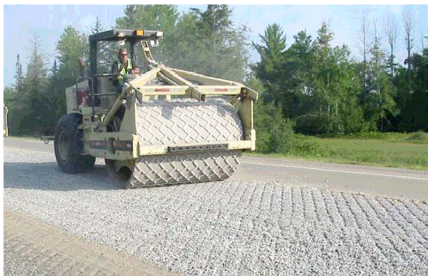
Figure 6-9 Z-Grid Roller Used on MHB Rubblized Pavement*
