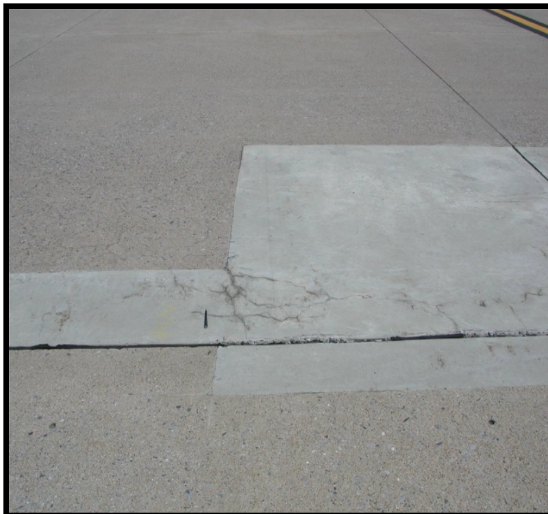
Figure B-22 Medium-Severity Large Patch
