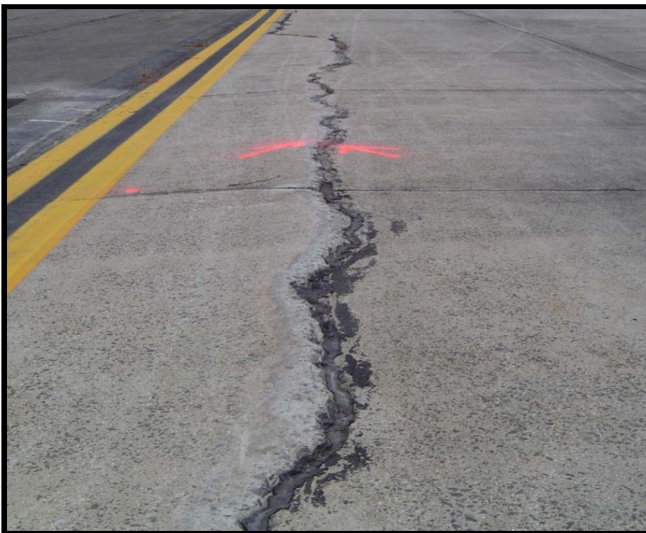
Figure B-2 Low-Severity Blowup
