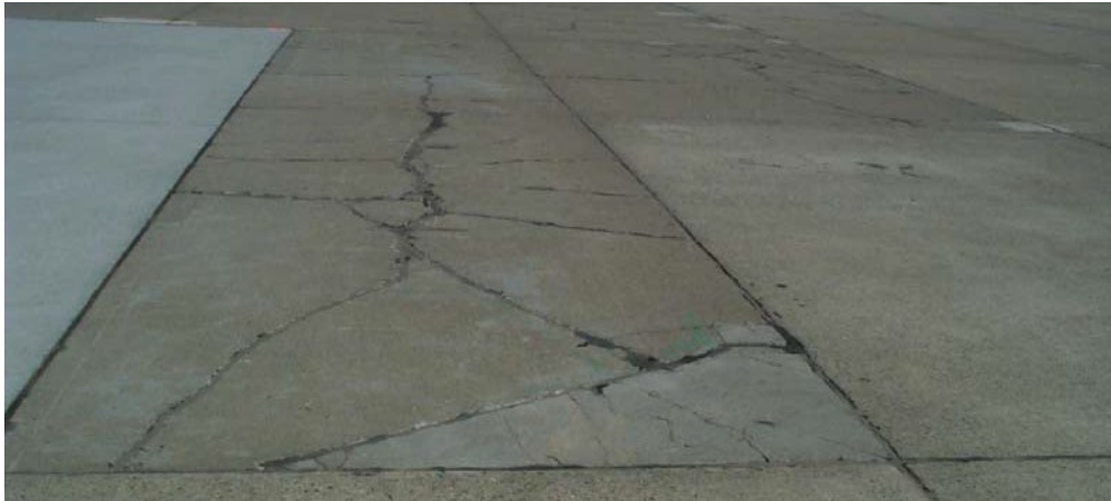
Figure 3-12 Shattered Slabs on Concrete Pavement
