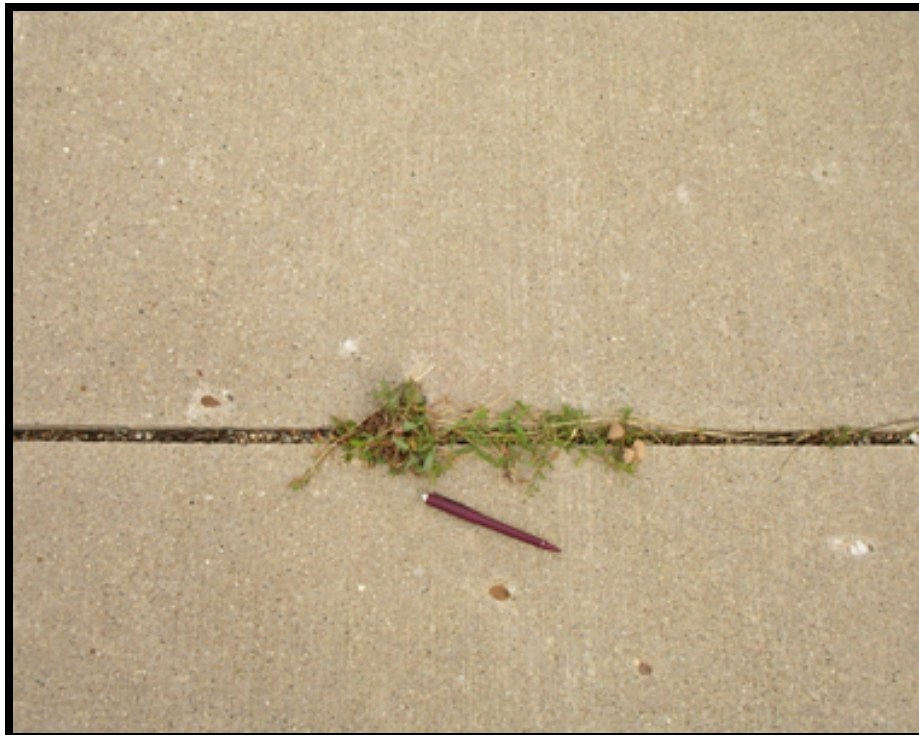
Figure B-17 High-Severity Joint Seal Damage
