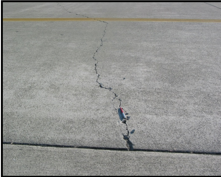
Figure B-10 High-Severity Linear Cracks
