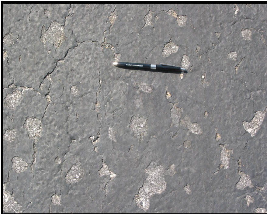
Figure A-41 High-Severity Raveling (Slurry Seal/Coal Tar Over Dense Mix)
