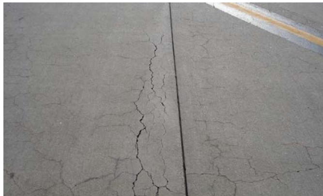
Figure 3-11 ASR Distress (Scaling/Map Cracking) on Concrete Pavement
