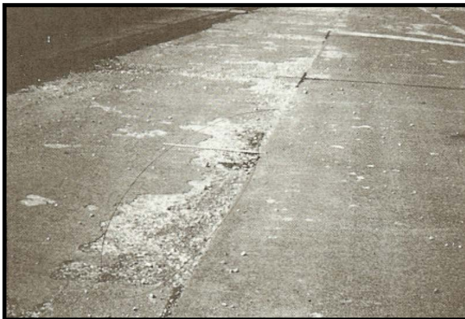
Figure B-29 High-Severity Scaling
