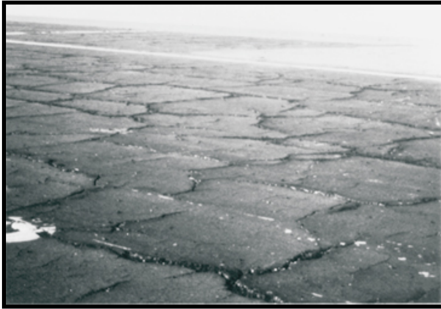
Figure A-11 High-Severity Block Cracking
