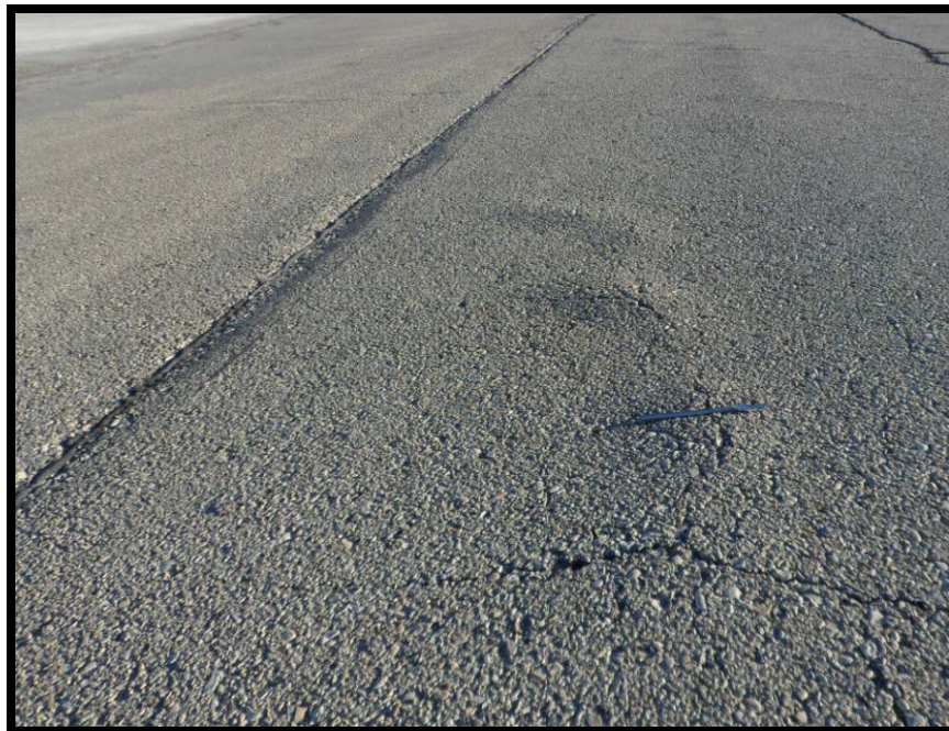
Figure A-51 Low-Severity Swell
