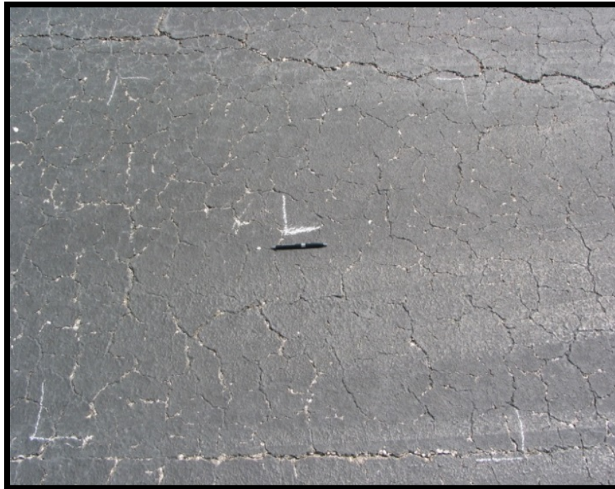
Figure A-39 Low-Severity Raveling (Slurry Seal/Coal Tar Over Dense Mix)
