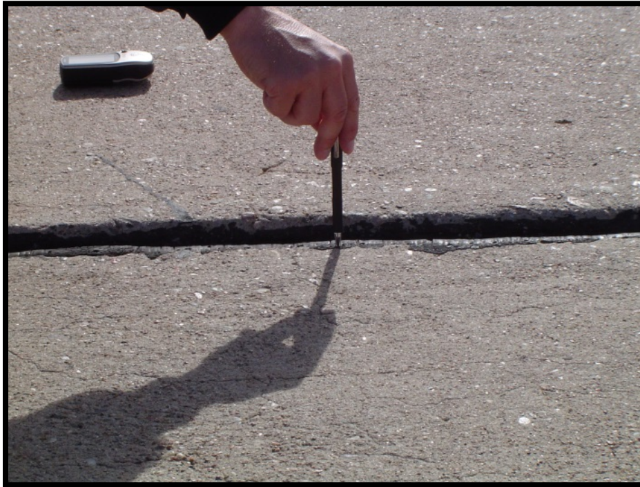
Figure B-32 High-Severity Settlement or Faulting
