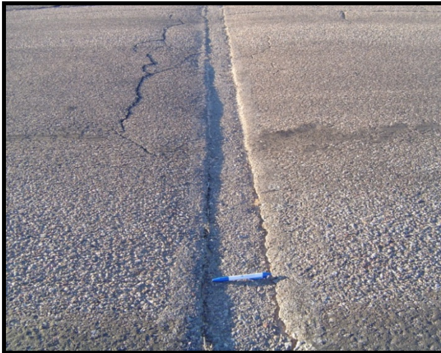
Figure A-33 Medium-Severity Patching
