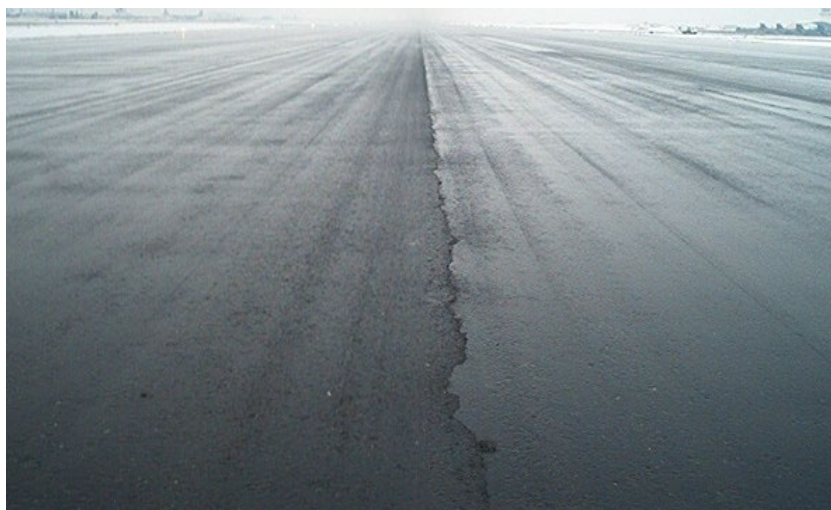
Figure 3-4 Longitudinal Cracking
