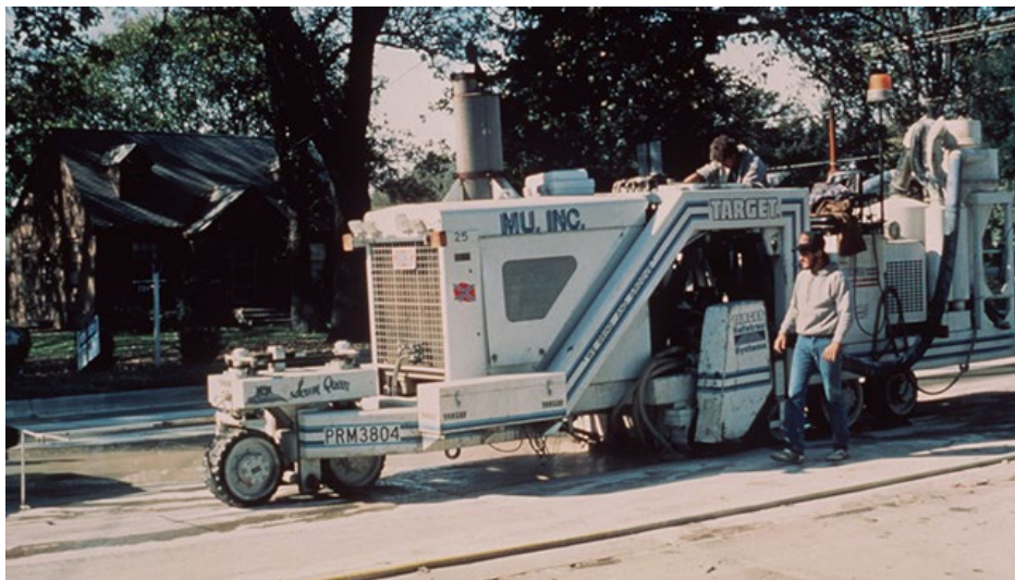
Figure 17-2 Gang-mounted Diamond Saw Blades
