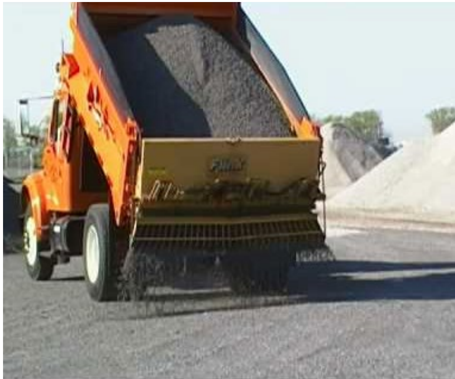
Figure 6-2 Applying Aggregate with Self-Propelled Hopper-type Spreader
