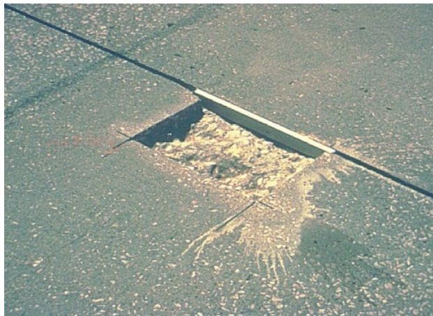
Figure 13-8 Compressible Insert
