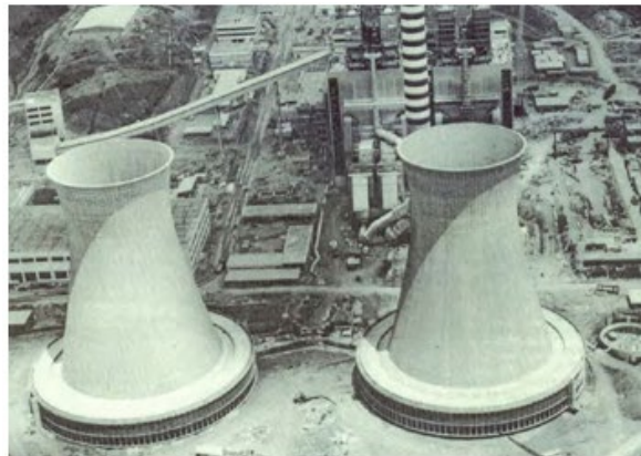
Figure 5-5 Hyperbolic Natural-Draft Cooling Towers
