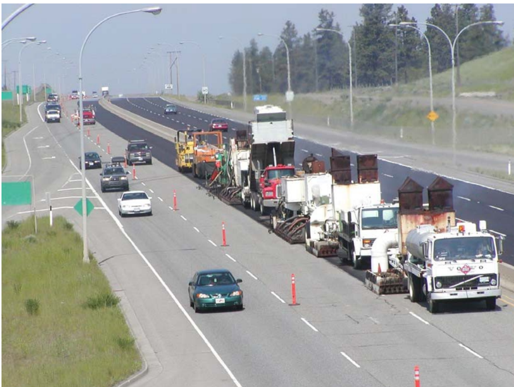
Figure 5-11 Example of Single Stage Remixing Train
