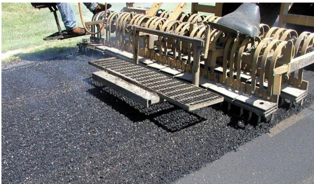
Figure 5-8 Surface Recycling Scarification Teeth*
