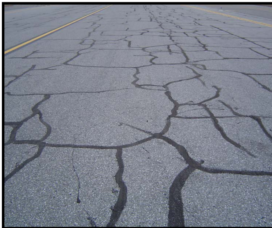
Figure A-6 Low-Severity Block Cracking
