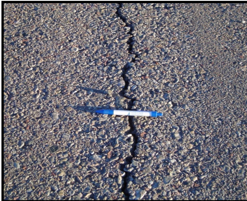
Figure A-25 Medium-Severity L&T Cracking
