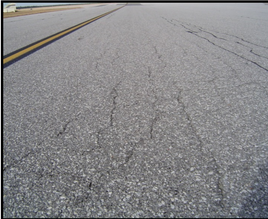
Figure A-2 Medium-Severity Alligator Cracking
