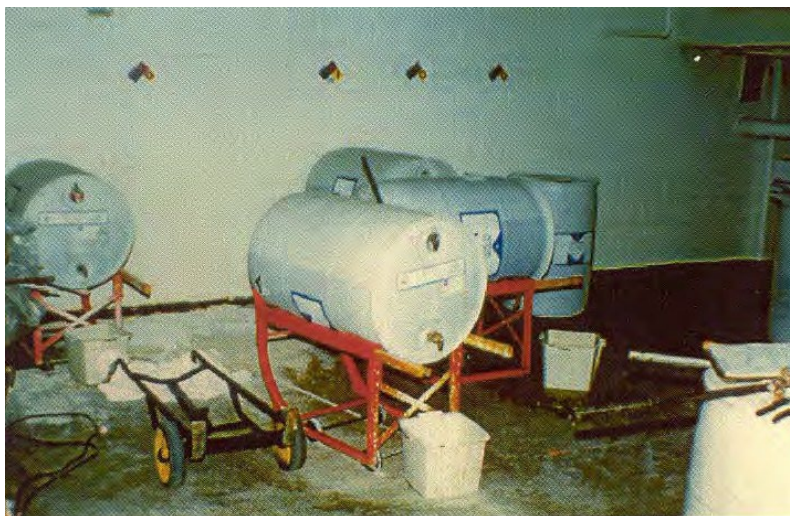
Figure 8-2 Manual Chemical Feed System
