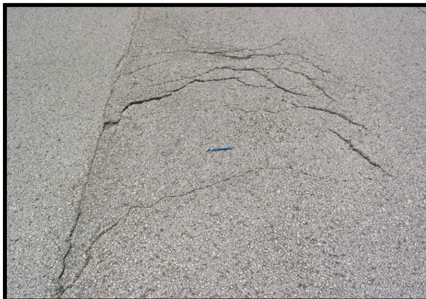
Figure A-50 Slippage Cracking
