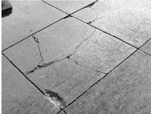
Figure 14-1 Shattered Slabs
