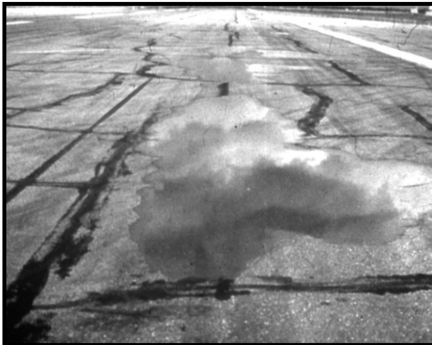
Figure A-18 High-Severity Depression
