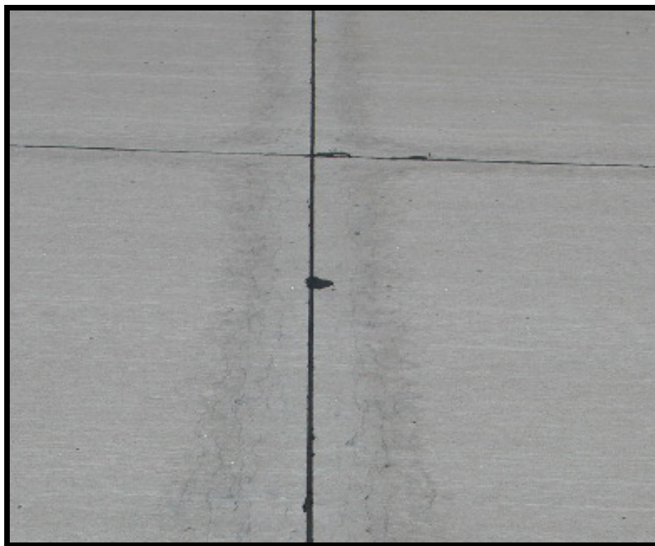
Figure B-12 Low-Severity “D” Cracking
