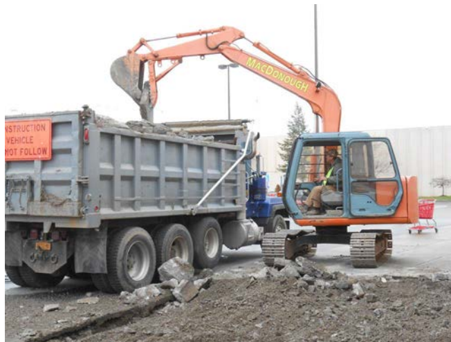
Figure 14-5 Concrete Removal Using Backhoe
