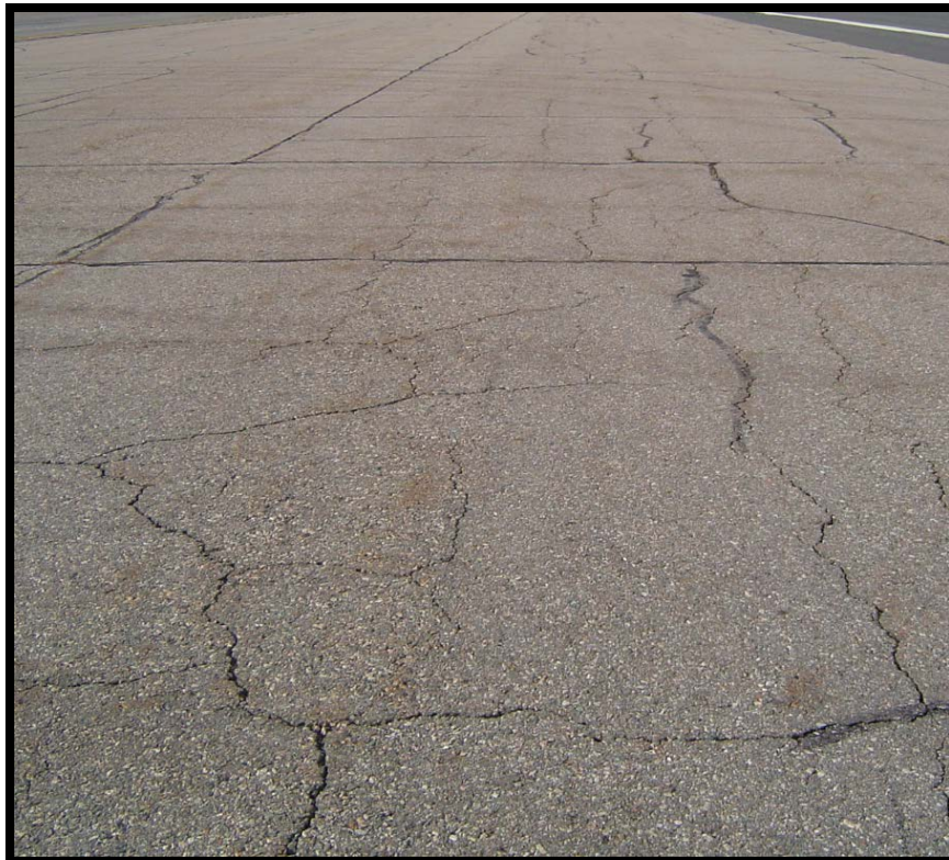
Figure A-8 Medium-Severity Block Cracking
