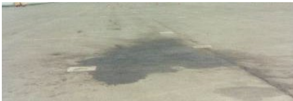
Figure 3-6 Fuel or Oil Spillage
