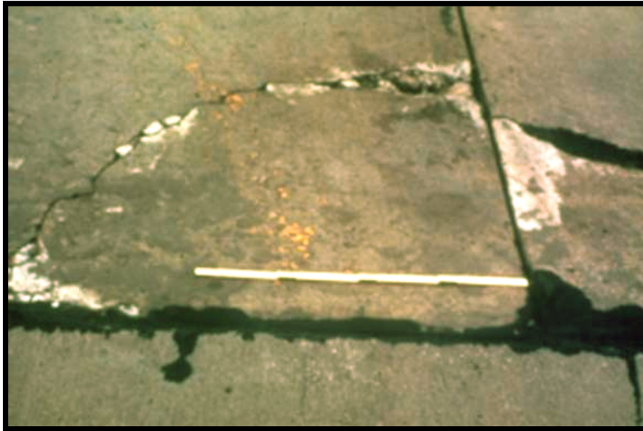
Figure B-7 High-Severity Corner Break
