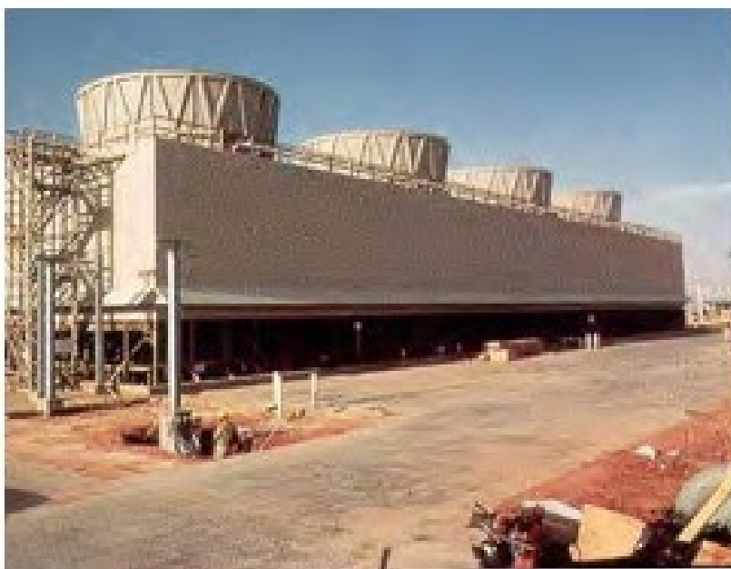
Figure 5-9 Counter-Flow Cooling Tower
