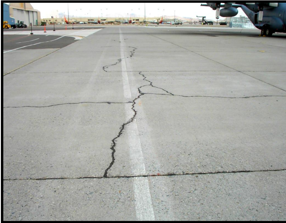
Figure B-35 High-Severity Shattered Slab/Intersecting Cracks
