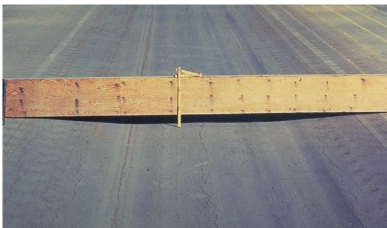
Figure 3-8 Rutting of the Pavement Structure
