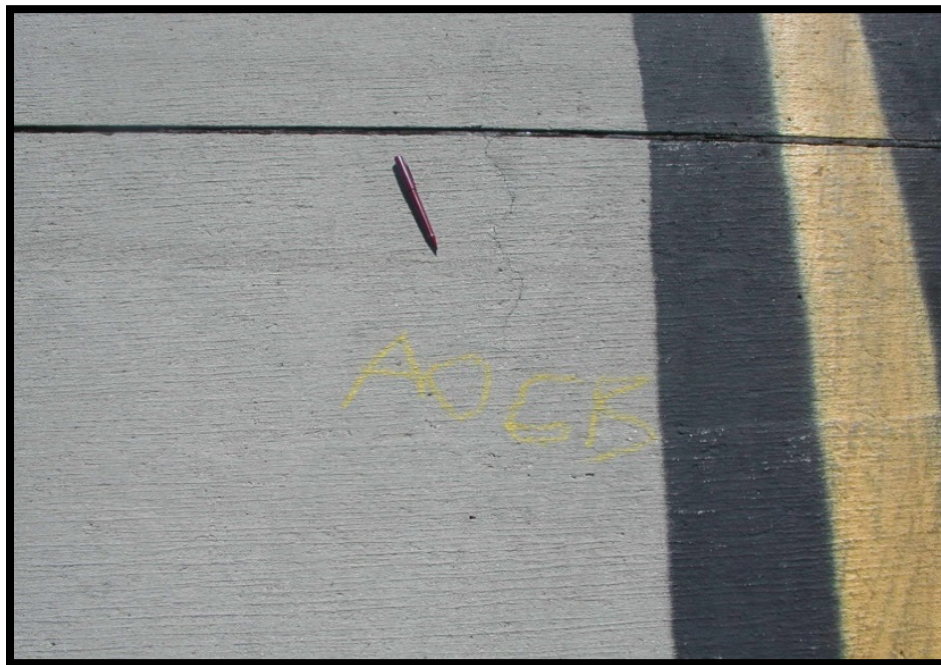
Figure B-36 Shrinkage Cracks
