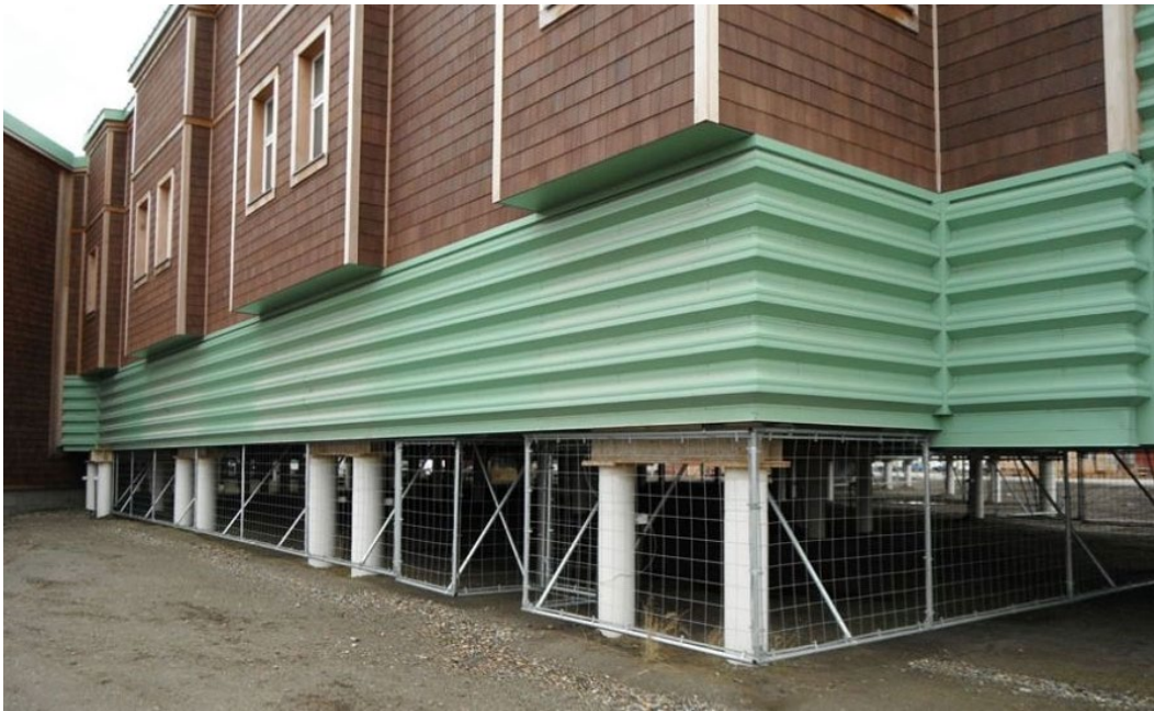
Figure A-18 Thermo-Helix Piles Supporting Elevated Structure (Kotzebue, Alaska)
