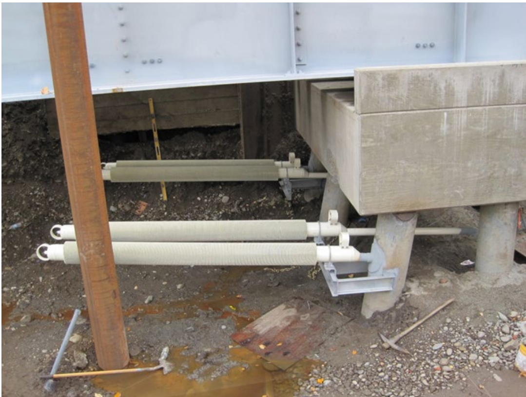
Figure A-14 Condensers (White) of Thermosyphons Configured within Foundation Piles (Goldstream Creek, Alaska)
