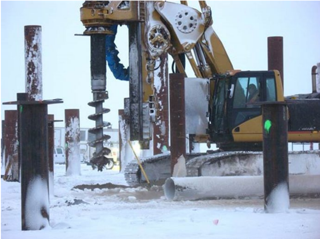
Figure A-16 Example Drilling Oversize Borehole (North Slope, Alaska)
