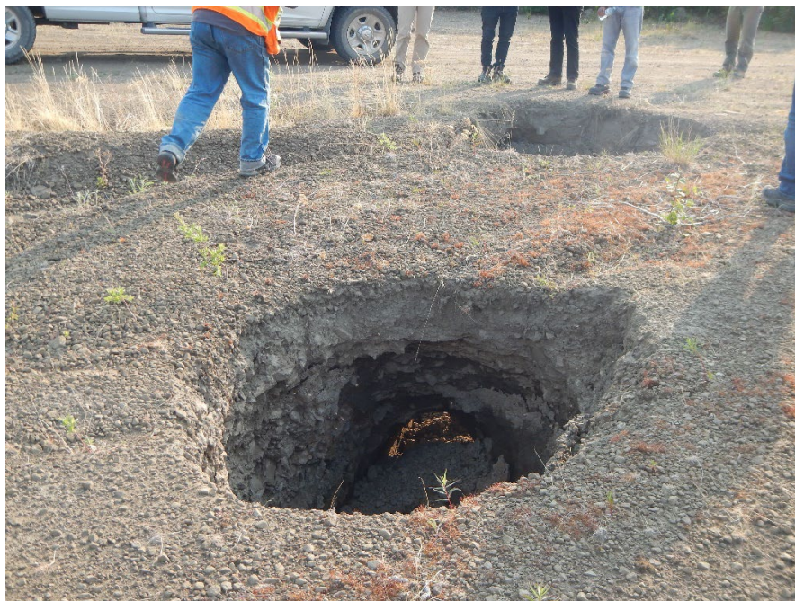
Figure A-3 Connected Sinkholes Formed after Material Site Development (Dempster Highway, Canada)
