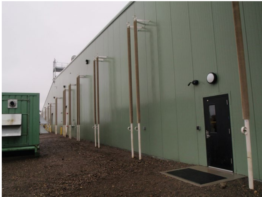
Figure A-13 Flat Loop Thermosyphon Condensers Configured Adjacent to an Aircraft Hangar with Flat Loops Extending Beneath Building Footprint (Deadhorse, Alaska)
