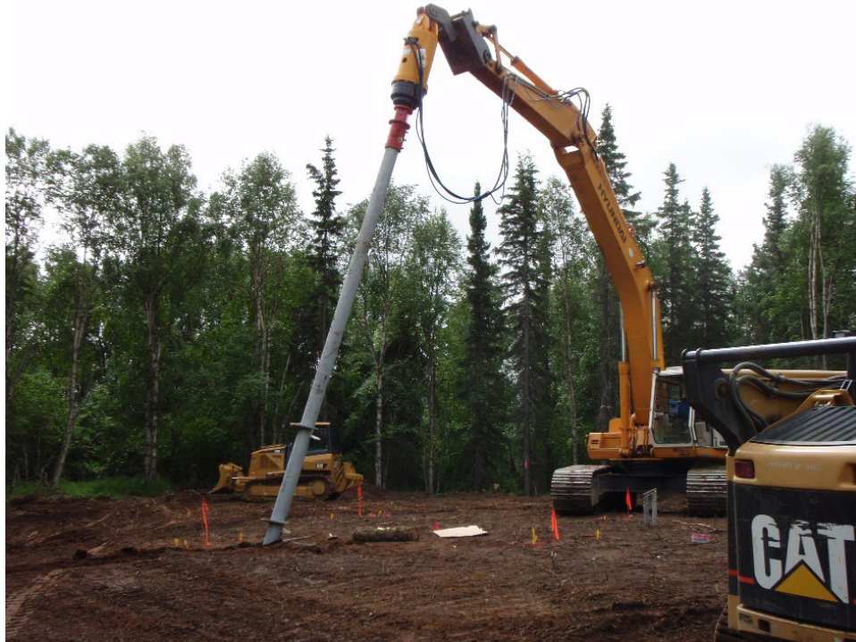
Figure A-19 Example Helical Pile (Western Alaska)
