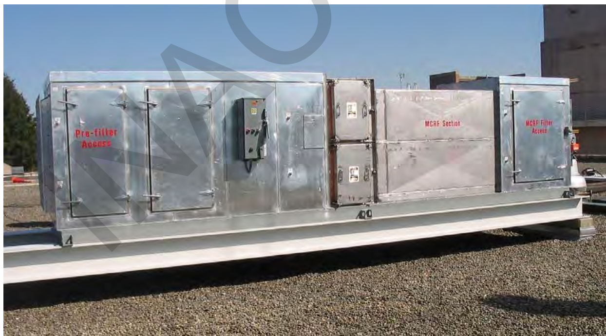
Figure G-12. Multi-Cell Radial-Flow (MCRF) Filtration Unit
