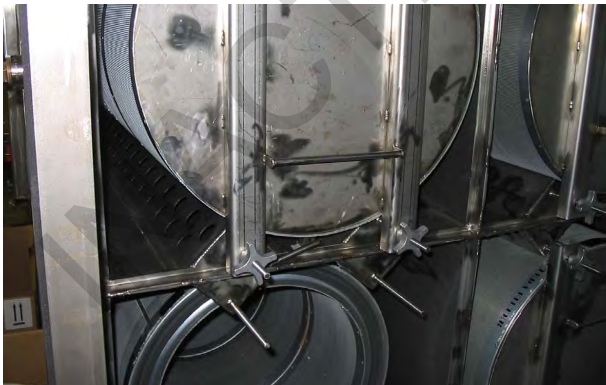
Figure G-14. Radial-Flow Filter Tubes
