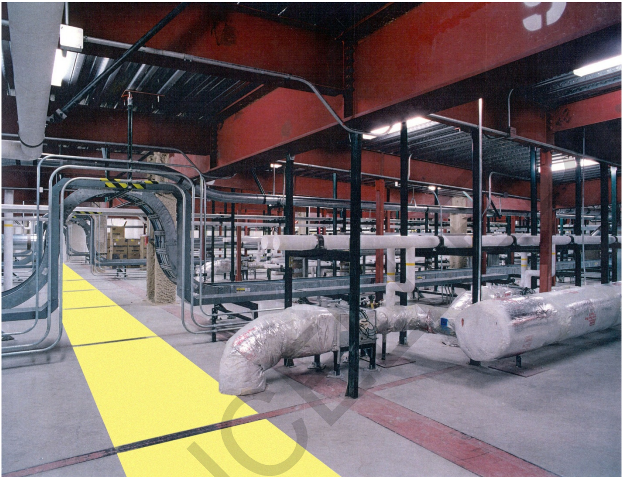
Figure E-3 Interstitial Access-Egress (Typical)
