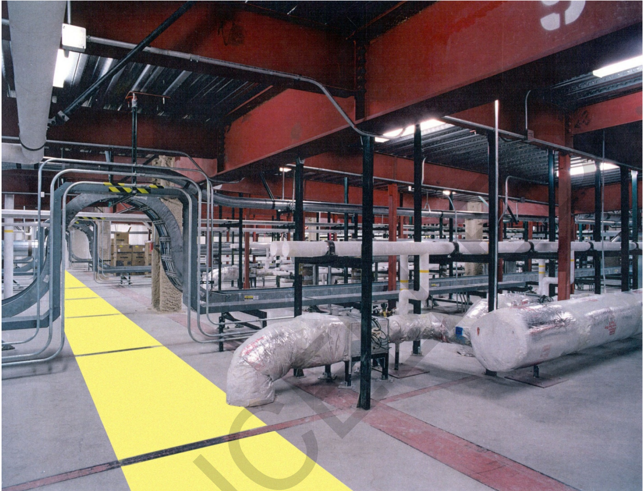
Figure E-3 Interstitial Access-Egress (Typical)
