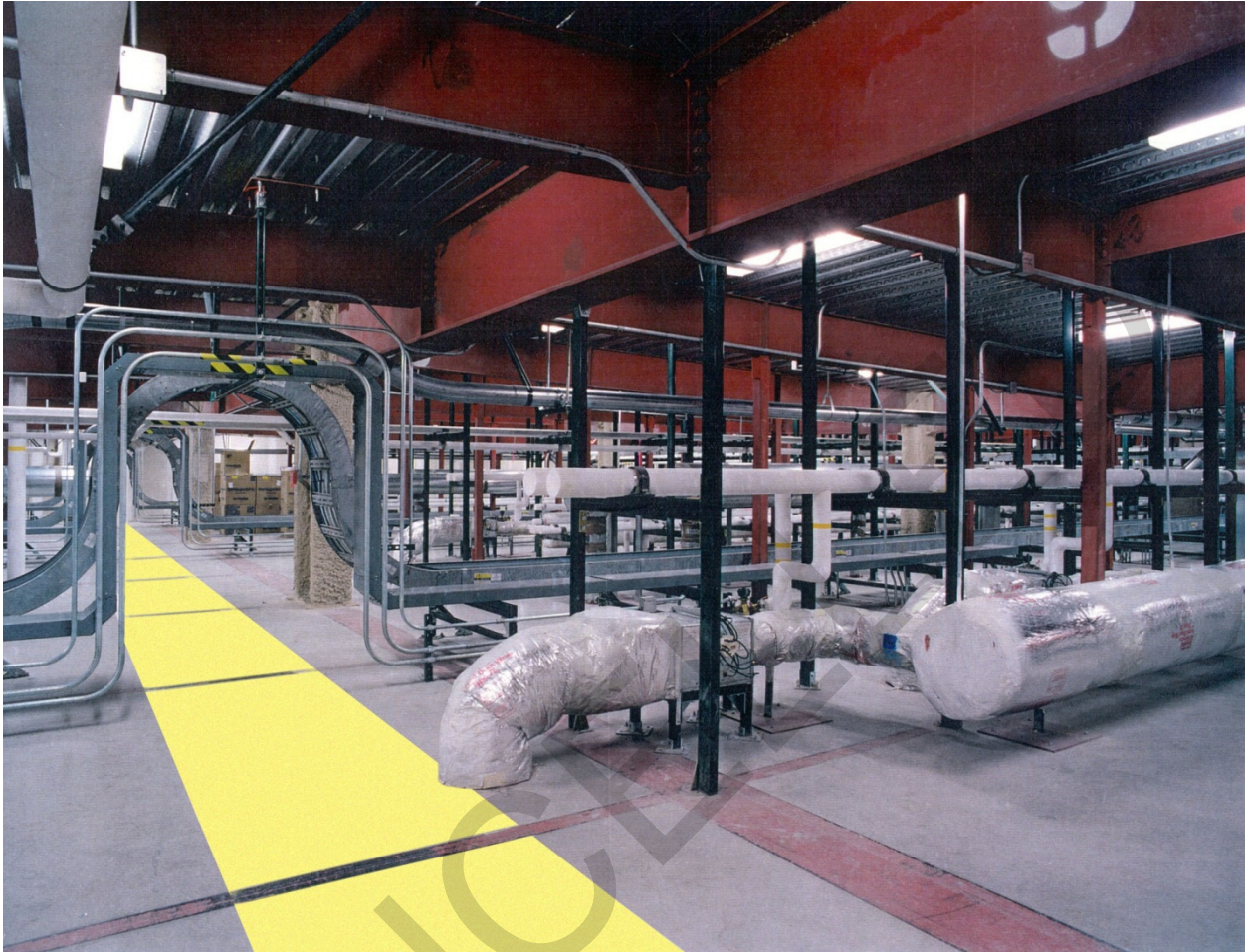
Figure E-3 Interstitial Access-Egress (Typical)
