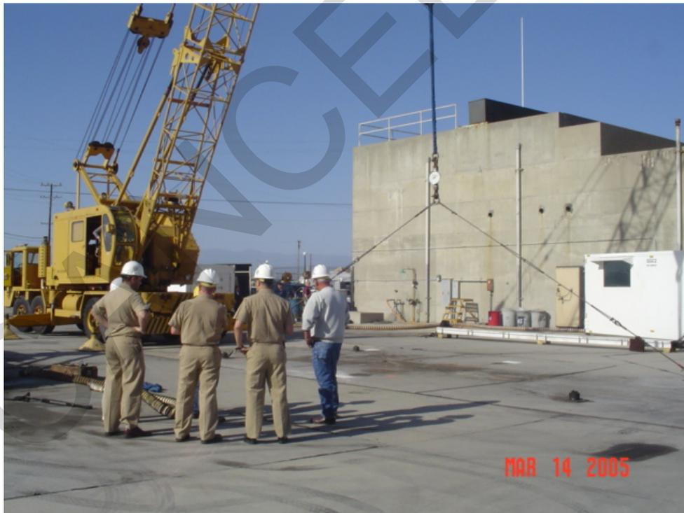
**Note:** This photo shows the detailed preparation necessary for a successful proof test: PW crew, crane, rigging gears and tension gage. The safety barricades were not yet in place when this photo was taken. Caution must be exercised to ensure that personnel and equipment are not injured or damaged due to an unanticipated release of the fitting.
