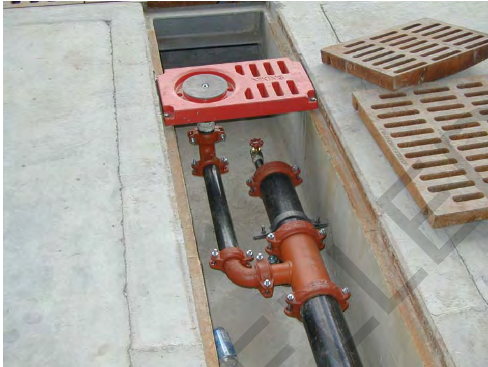
Figure 5-4 Trench Drain Detail
