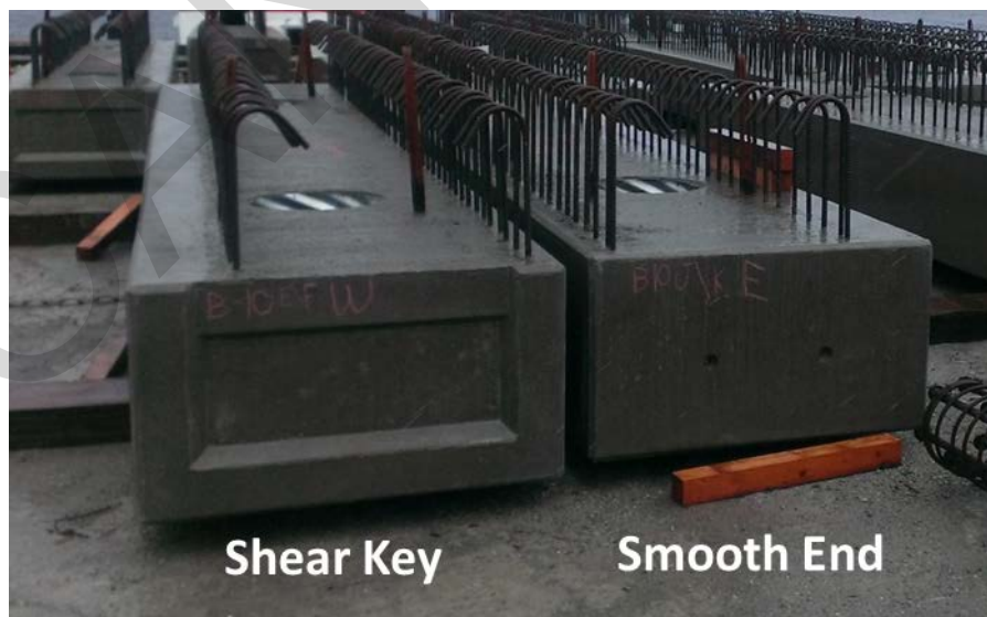
Precast Pile Cap Showing End Configurations
