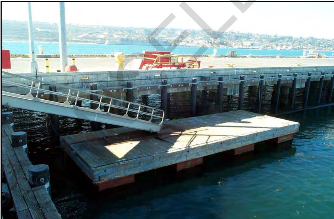
**Figure 5-7 Plastic Fender Pile System.**
