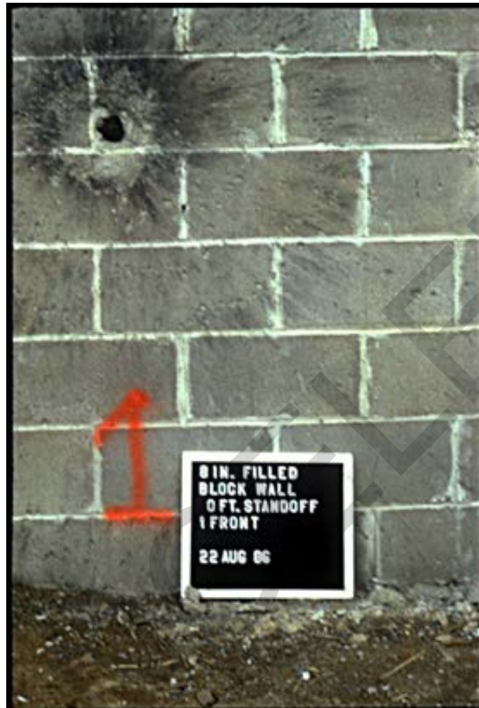
Figure 2-3. Shaped Charge Penetration of Masonry
