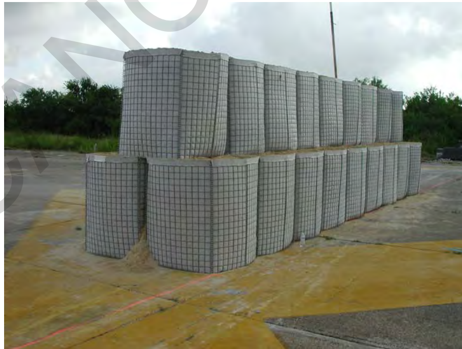
Figure F-3 Hesco Bastion Concertainer Barrier, Oblique View
