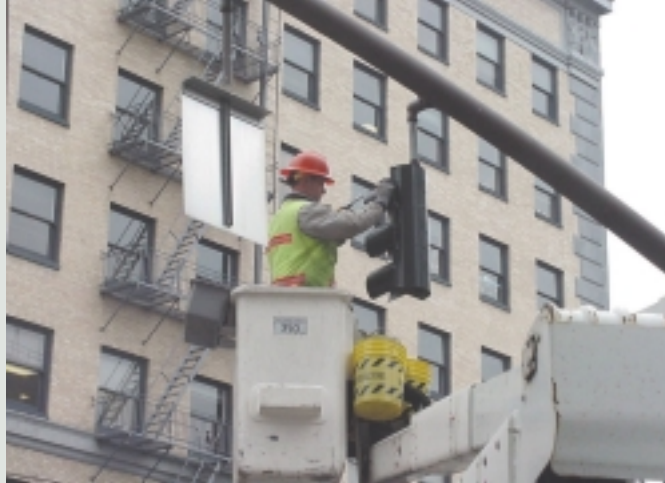
A City-bired contractor installs one of more than 13,000 LED lamps during the fall of 2001.
