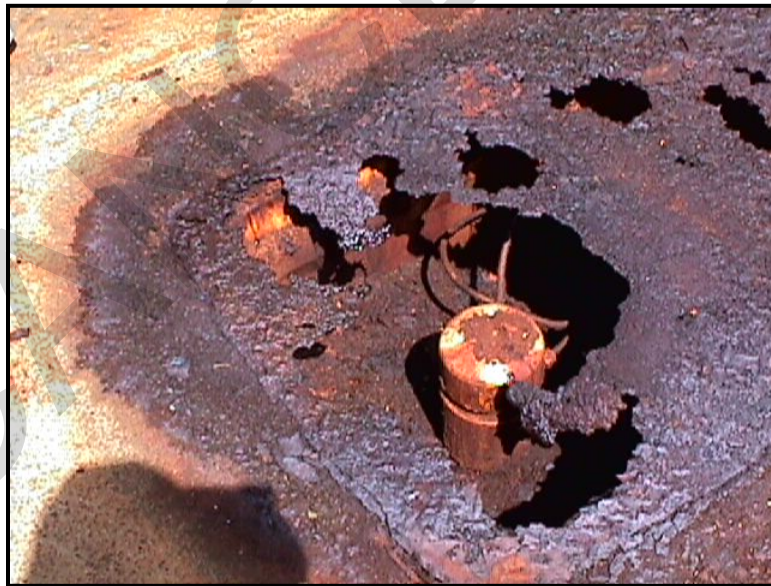
Figure B-24 Severe Corrosion of Cast Iron Cover on the Anode Well Head Box Caused By Chlorine Gas Vented into the Box.
