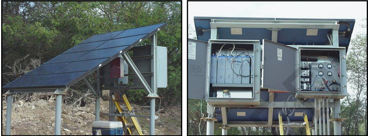
Figure 4-2 Small Solar Powered CP System. Solar Panels Shown in Picture on Left. Battery Bank and Control Center Shown on Right.
