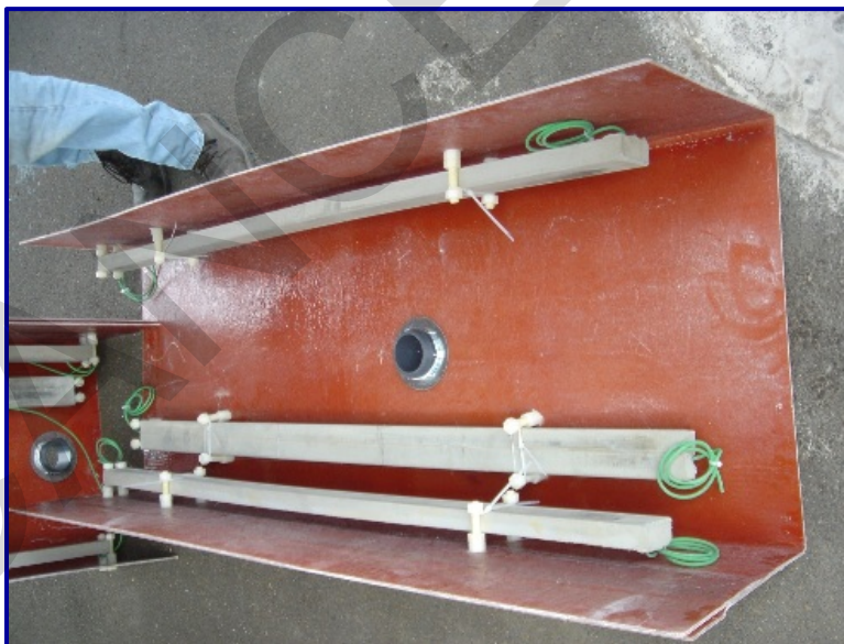
Figure B-28 Discrete Zinc Anodes in Fiberglass Jacket for Pile Installation.
