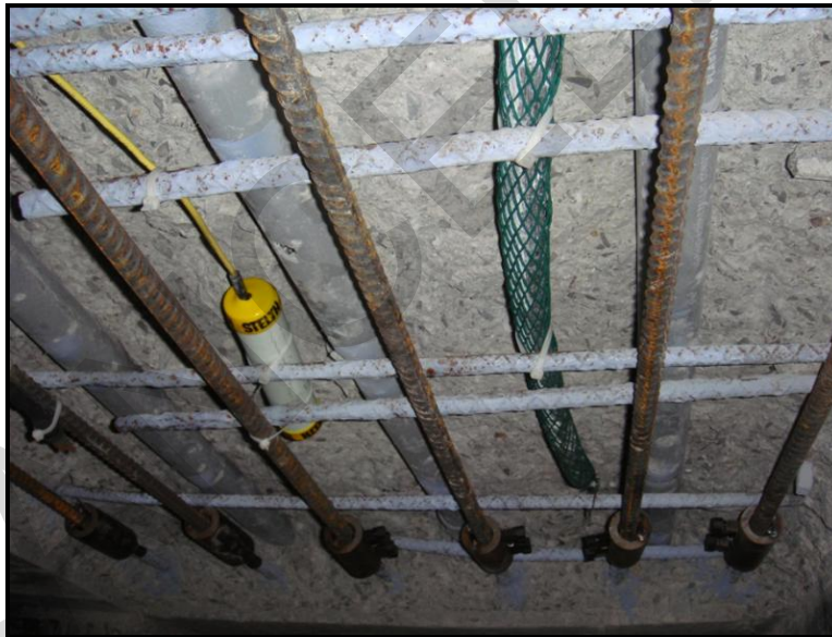
Figure 4-8 Discrete Zinc Anode (Wrapped in Green Mesh) in Concrete Deck Repair. Device with Yellow Lead Wire is a Permanent Reference Electrode.
