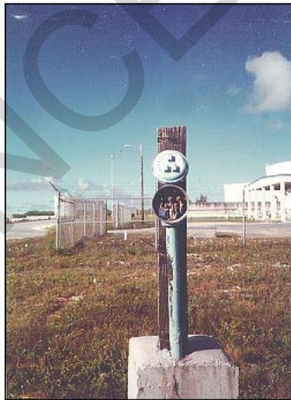
Figure B-7 Above Grade Test Stations. PVC Pipe Mount on the Left, Pole Mount in the Center, and Wall Mount on the Right.
