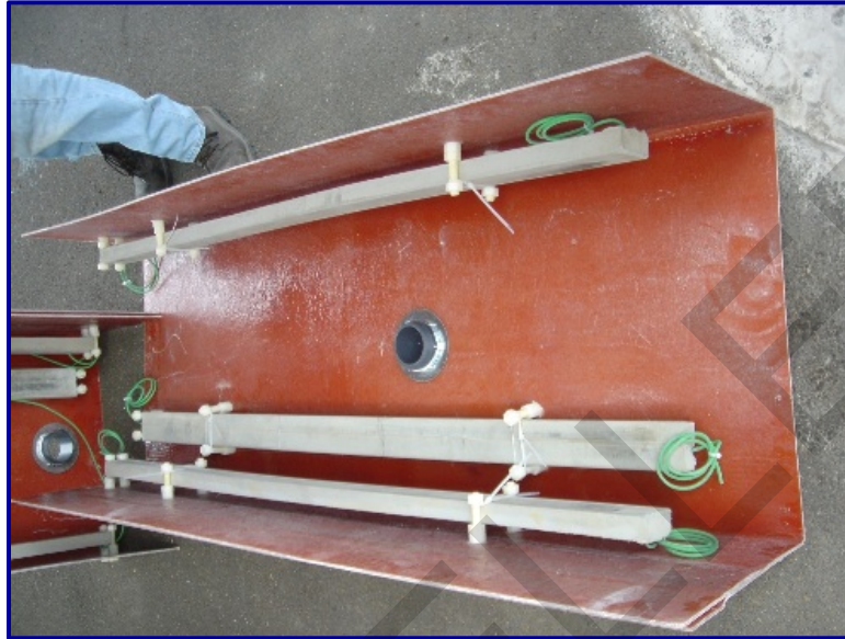
Figure 4-9 Discrete Zinc Anodes in Fiberglass Jacket for Pile Installation.
