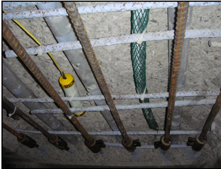
Figure B-27 Discrete Zinc Anode (Wrapped in Green Mesh) in Concrete Deck Repair. Device with the Yellow Lead Wire is a Permanent Reference Electrode.
