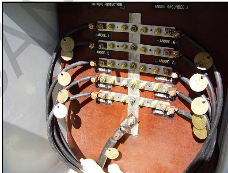
Figure B-18 Anode Junction Box
