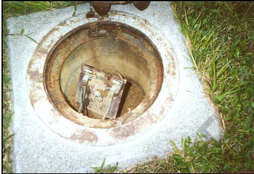
Figure B-9 Flush Mounted Current-Potential Test Station
