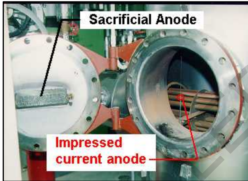
Figure B-34 CP System for a Vertical Hot Water Tank with a Man-Way Access Opening.
