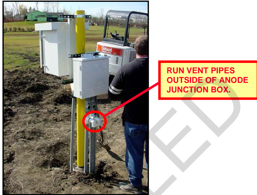
Figure B-23 Anode Column Vent Pipes Run Outside of Anode Junction Box.
