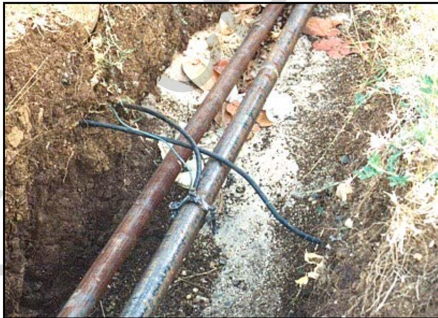
Figure 4-5 Mechanical Connection of Wiring to the Structure
