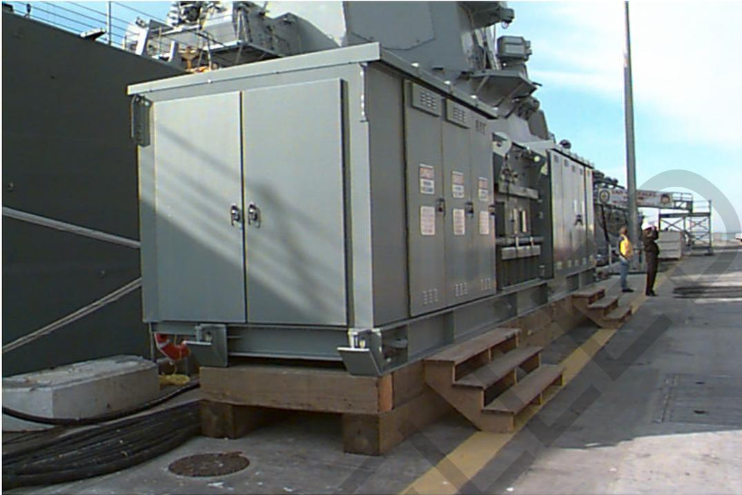
Picture C. A skid-mounted substation
