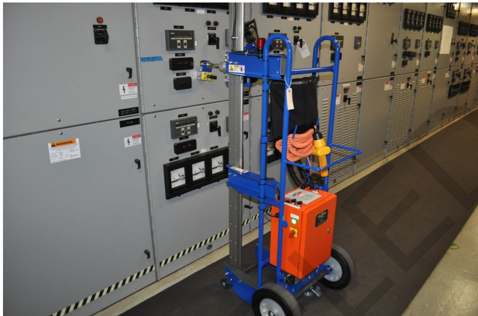
Figure 1. Remote Racking Mechanism
