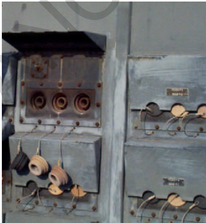
Figure 12-5. Skid-Mounted Substation with Single-Pole Connections
