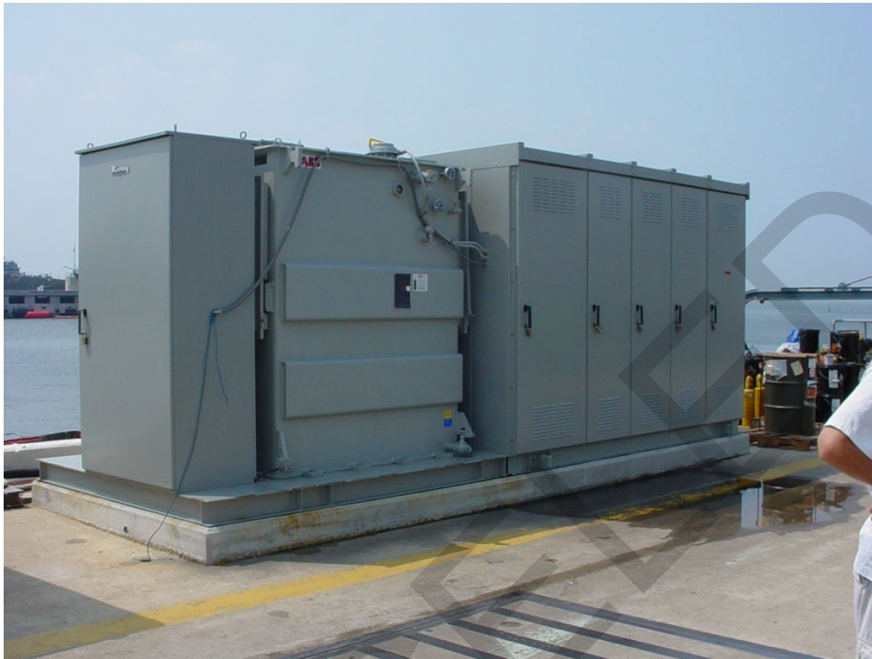
Figure 12-5. Skid-Mounted Substation with Single-Pole Connections
