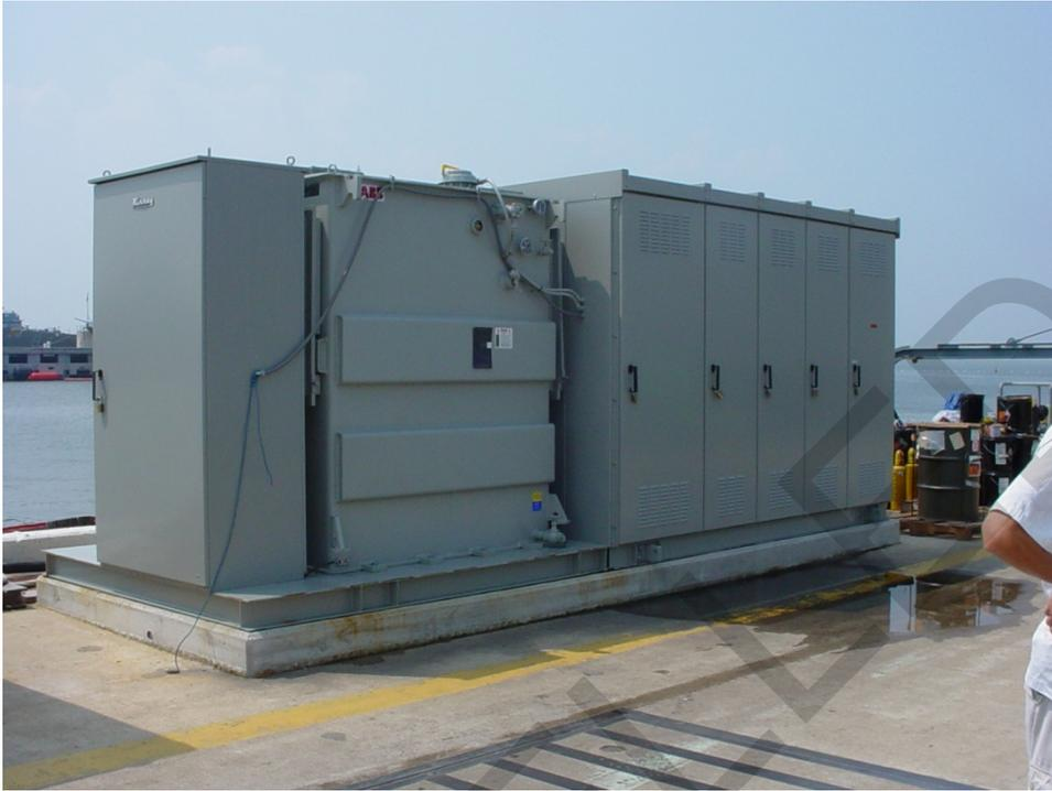
Figure 12-5. Skid-Mounted Substation with Single-Pole Connections
