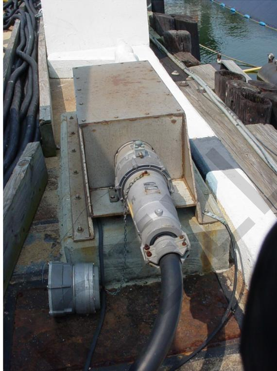
Figure 12-2. Close-Up of Electrical Connection Outlet Assembly
