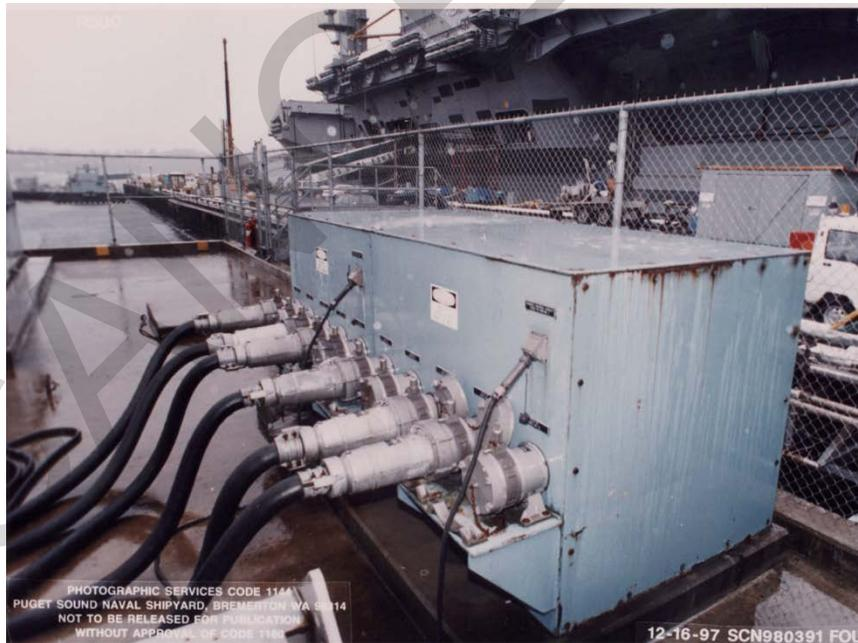
**Figure 12-9. 4.16 kV Pier Electrical Outlet Assembly and Outlets – Newer Designs**
