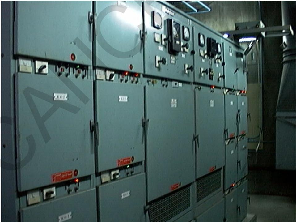
Figure 12-4. Skid-Mounted Substation
