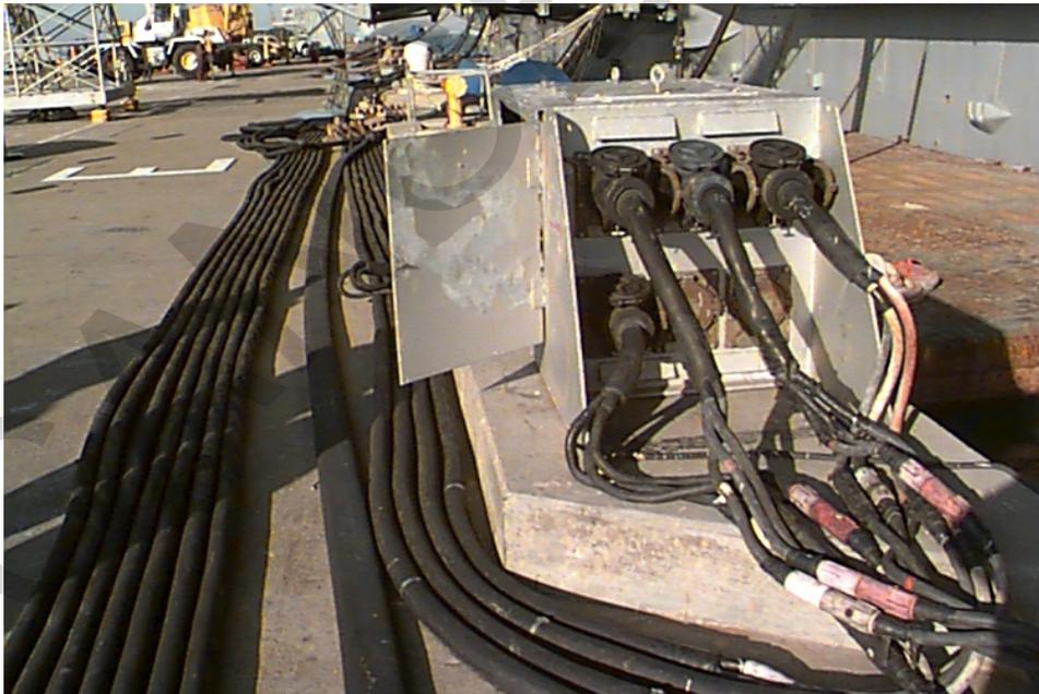
**Figure 12-13. 480 Volt Shore-Cable to Ship-Cable Splice Connection in Place**
